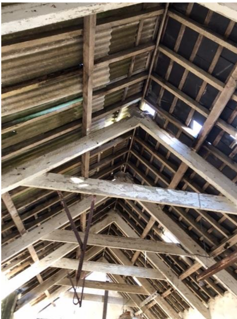
Internal roof structure
