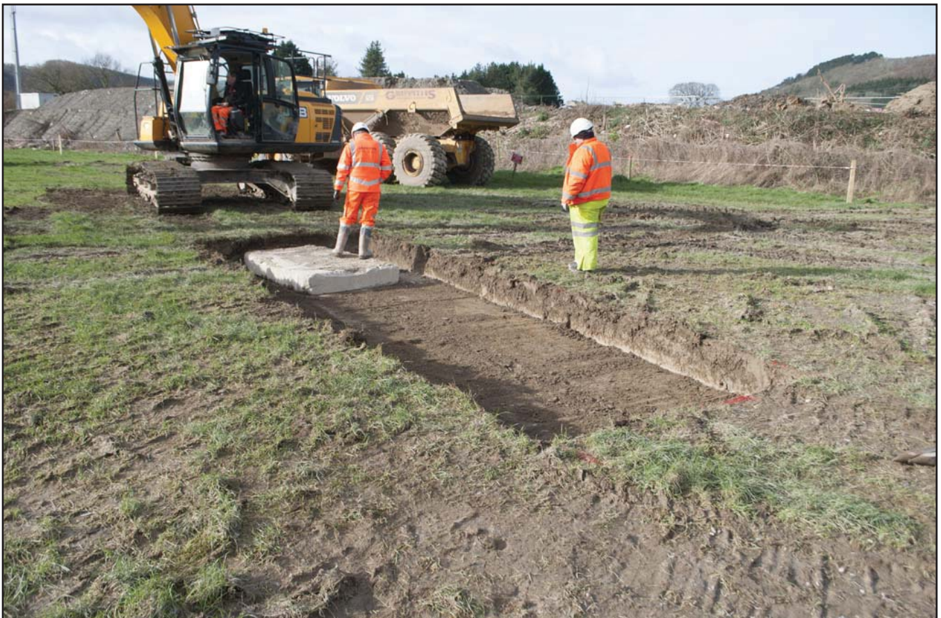
Plate 29: Working shot showing the laying of protective concrete slabs; scale not used; view from NE (archive reference: G2589_117).
