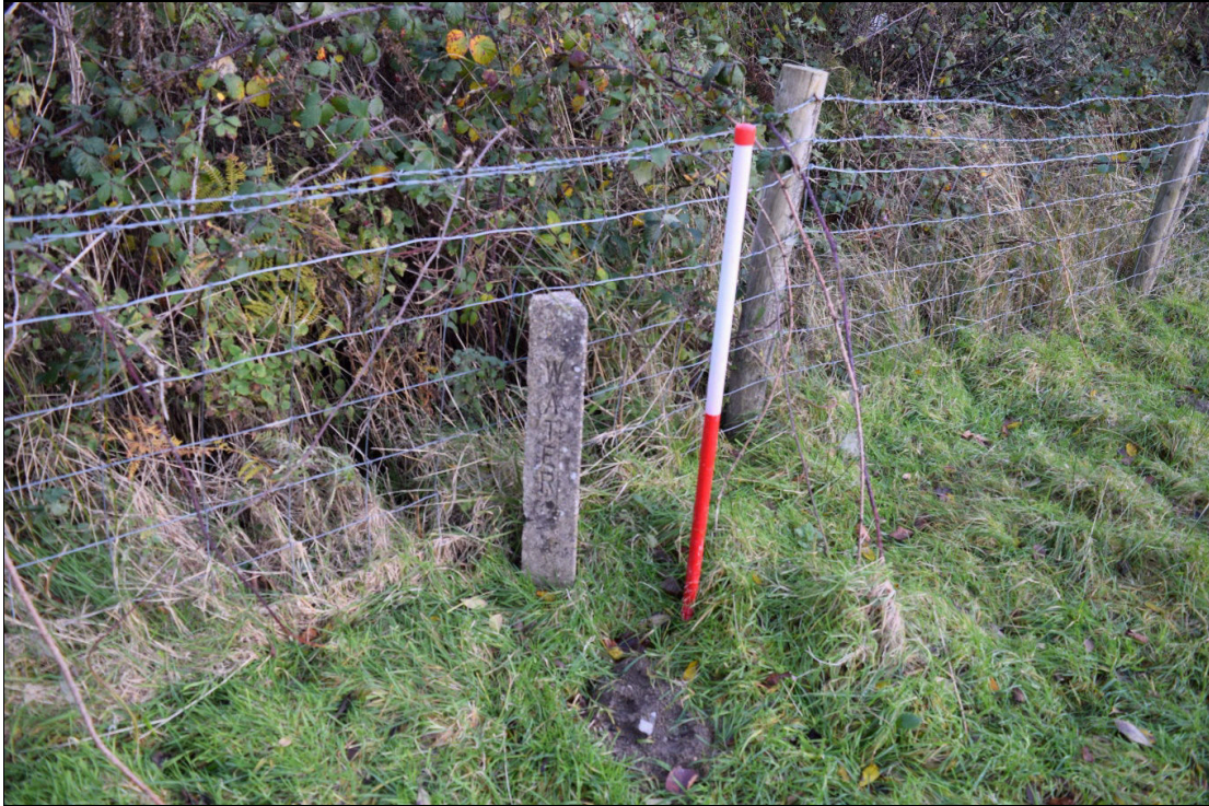
Plate 13 - DOL2022_013: A view of a concrete post marking the line of the water main, on the proposed Active Travel Route. Looking east-southeast.
