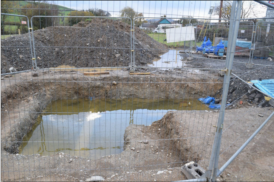
Plate 7 - DOL2022_007: A view of the excavations for the water mains showing the underlying soils. A thin topsoil lies over a boulder clay subsoil. Looking south-southwest.
