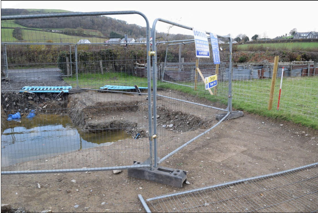
Plate 5 - DOL2022_005: A view of the excavations for the water mains showing the underlying soils. A thin topsoil lies over a boulder clay subsoil. Looking west-northwest.
