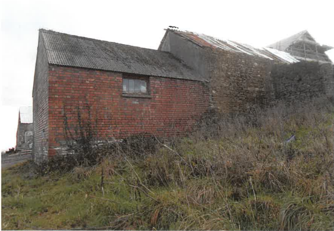
View of north-west elevation showing brick and stone extensions (B9)
