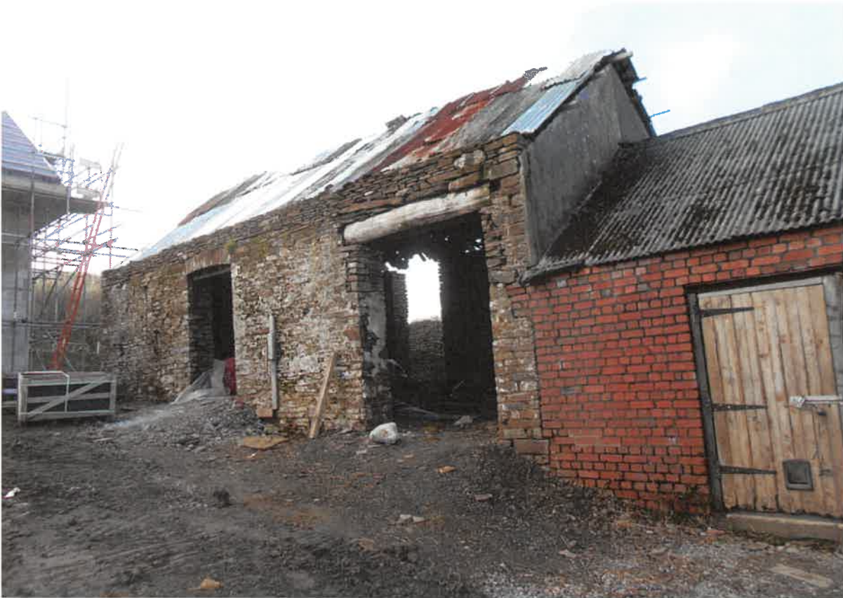
View of the south-east elevation showing the wooden lintel & brick extension (B5)
