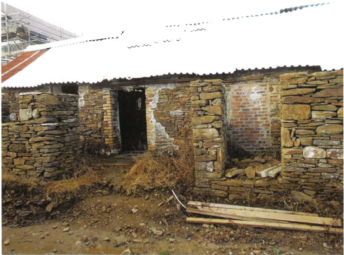
South-east elevation showing brick inserts and freestanding stonework (A3)
