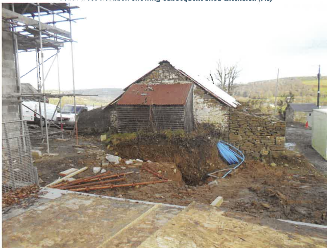
Gable end with shed extension Shows freestanding stonework on south-east elevation (A6)
