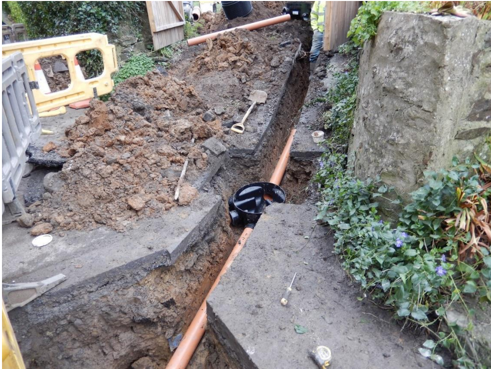
Photo 11 – Trench 2 after excavation, from northeast. The yellow-orange natural clay 008/103 can be seen through the length of the trench, cut by feature 006, with a darker fill 005, to the right.
