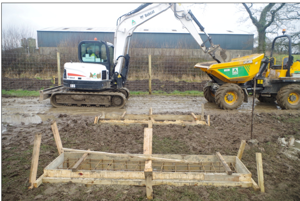
Plate 8: Substation 2, Footing 1 and 2, with concrete moulds in place
