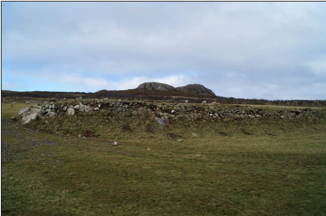
Plate 28. TBS2020_028: Stone revetting appears to have been added to a landform here to create an effective Revetted Boundary, HER PRN 114855.
