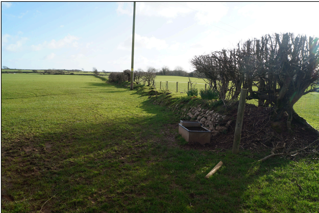
Plate 52. TBS2020_052: Another example of an earth Hedgebank, HER PRN 114874, which has sections of stone facing, with possibly a patched repair around the water trough where animals have damaged the bank.
