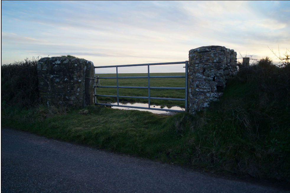
Plate 41. TBS2020_041: Mortared Stone pillars at a field gate at SM8041403807. Not an uncommon sight in this area.
