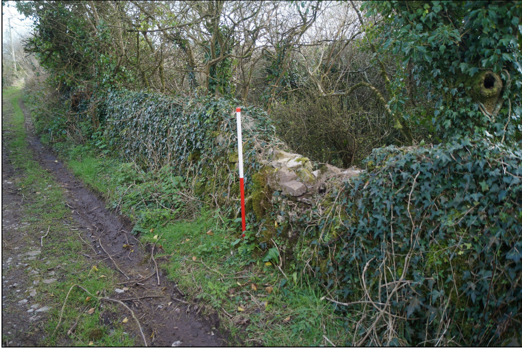
Plate 61. TBS2020_061: Mortared Walls, often relatively thin, are most commonly found along lanes and tracks. They are often slightly damaged. Here, HER PRN 114878, local limestone and lime mortar have been used, in this wall along side Haylands Lane, Jameston.
