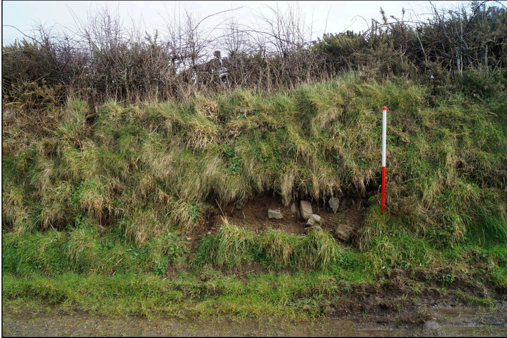
Plate 15. TBS2020_015: A damaged roadside boundary bank, no HER PRN, with exposed stonework revealing that it is a Cloddiau Variant, rather than a simple Hedgebank.
