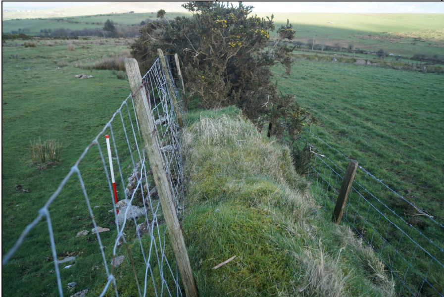
Plate 8. TBS2020_008: The top of the section of boundary, HER PRN 114840, shown in the previous image. Like all Cloddiau Variants there is stone to either side with an earth core, topped with turf and usually a hedge. The hedge is absent here and it is not known if the gorse is a relic of a gorse hedge planted along the boundary when it was constructed.
