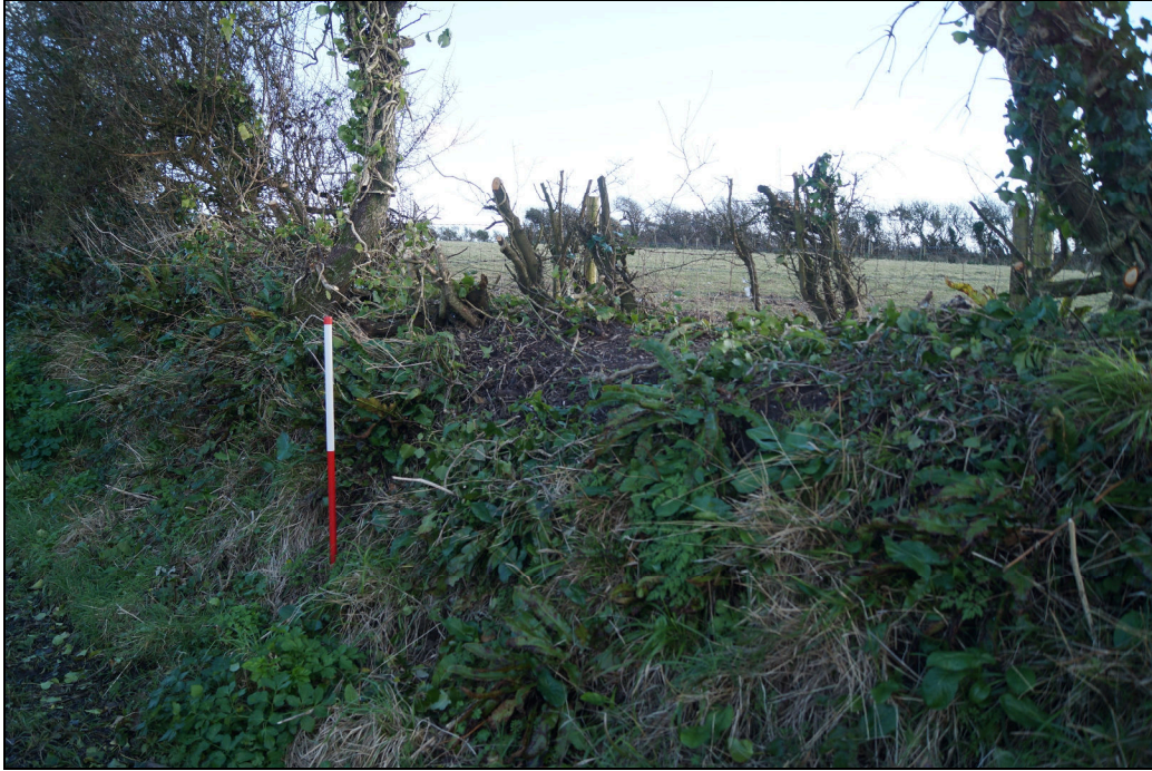
Plate 45. TBS2020_045: A Hedgebank near Jameston, HER PRN 114870. This single bank varied in character with some sections built of earth and others being stone-faced in the Cloddiau style. Individual boundary banks could clearly change character depending on the materials available to construct them.
