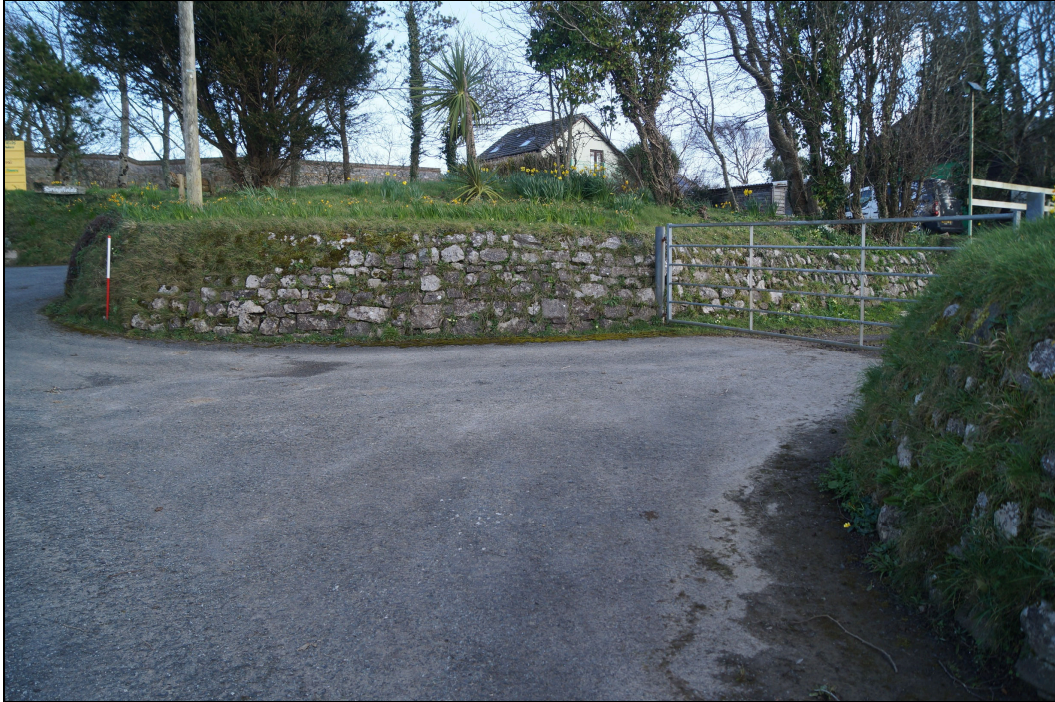
Plate 59. TBS2020_059: A Revetted Boundary close to a farm at SS0675098600. Stone is most commonly used in boundaries in close proximity to houses and gardens. Not recorded.
