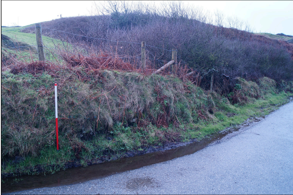
Plate 17. TBS2020_017: A roadside bank, HER PRN 114849, at Ceibwr. Stonework exposed at the base of the bank puts this example in the Cloddiau Variation category. There is no hedge on the bank and a post and wire fence makes the boundary secure.
