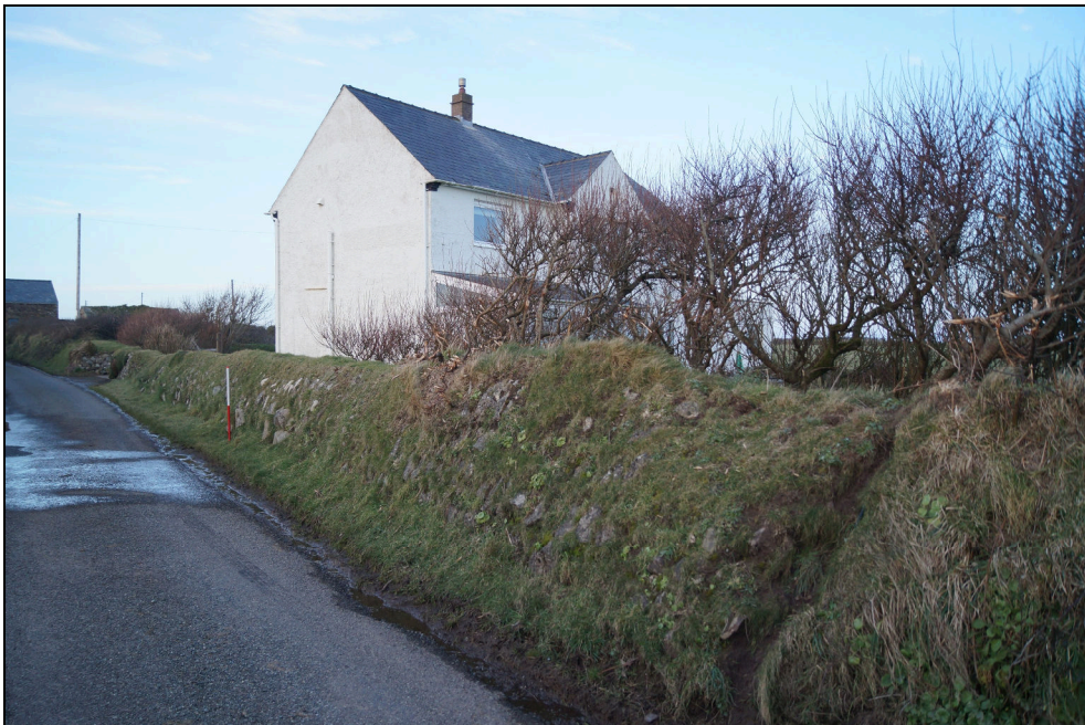
Plate 40. TBS2020_ 040: A Cloddiau Variant, HER PRN 114866, apparently a stone-faced, earth bank, used in a garden boundary at Kete.
