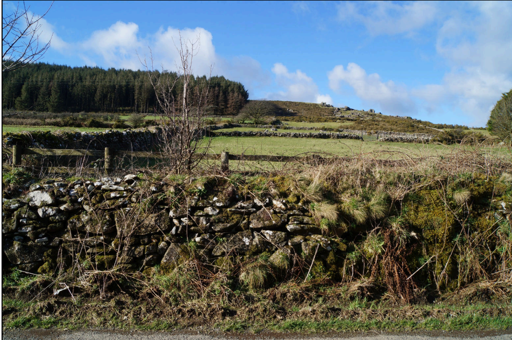
Plate 1. TBS2020_001: A Dry Stone Wall, HER PRN 114832, at the roadside with further Dry Stone Wall boundaries extending up the slope at Llethr. The use of stone reflects the ample supply of outcropping stone here on the south-facing Preseli slopes.
