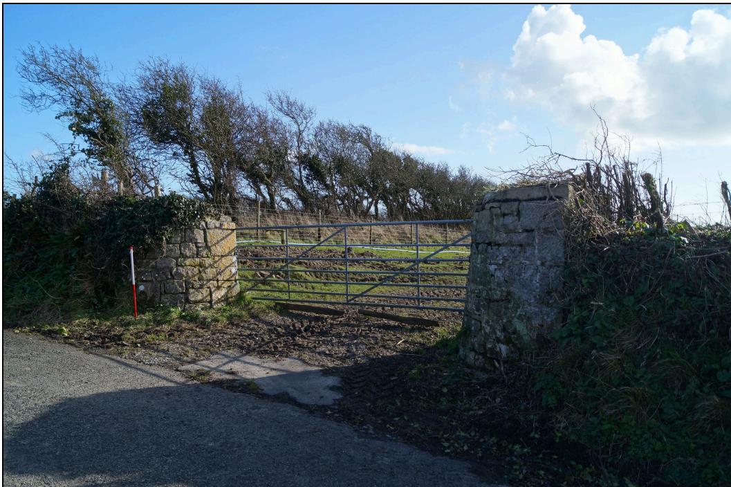
Plate 58. TBS2020_058: Mortared stone pillars at field gates such as these at SS0684398577, are not an uncommon sight in the Manorbier area. Local limestone has been used and presumably locally produced lime mortar.
