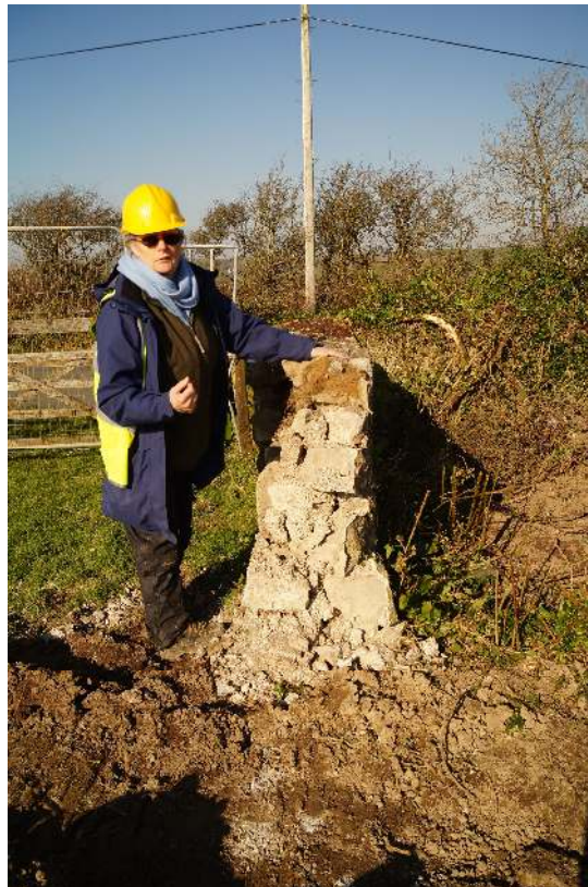
Plate 20: GGJ2019_120, Cross section of wall showing concrete bond, looking north-northeast.
