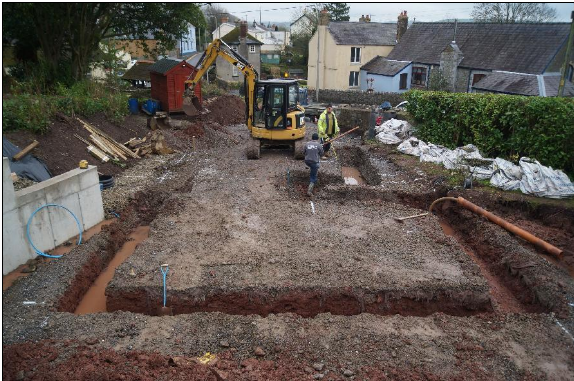
Plate 6: RCL2018_106, From the top of the retaining wall to the west looking east. Trenches visible show subsoil (002) under the layer of scalpings deposited to firm up the ground surface during the construction of the retaining wall.
