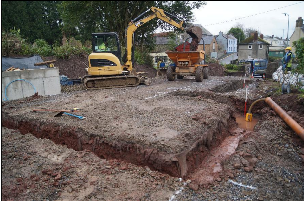
Plate10: RCL2018_110, House foundation trenches looking northeast, the furthest trenches were cut only though scalplings not subsoil.
