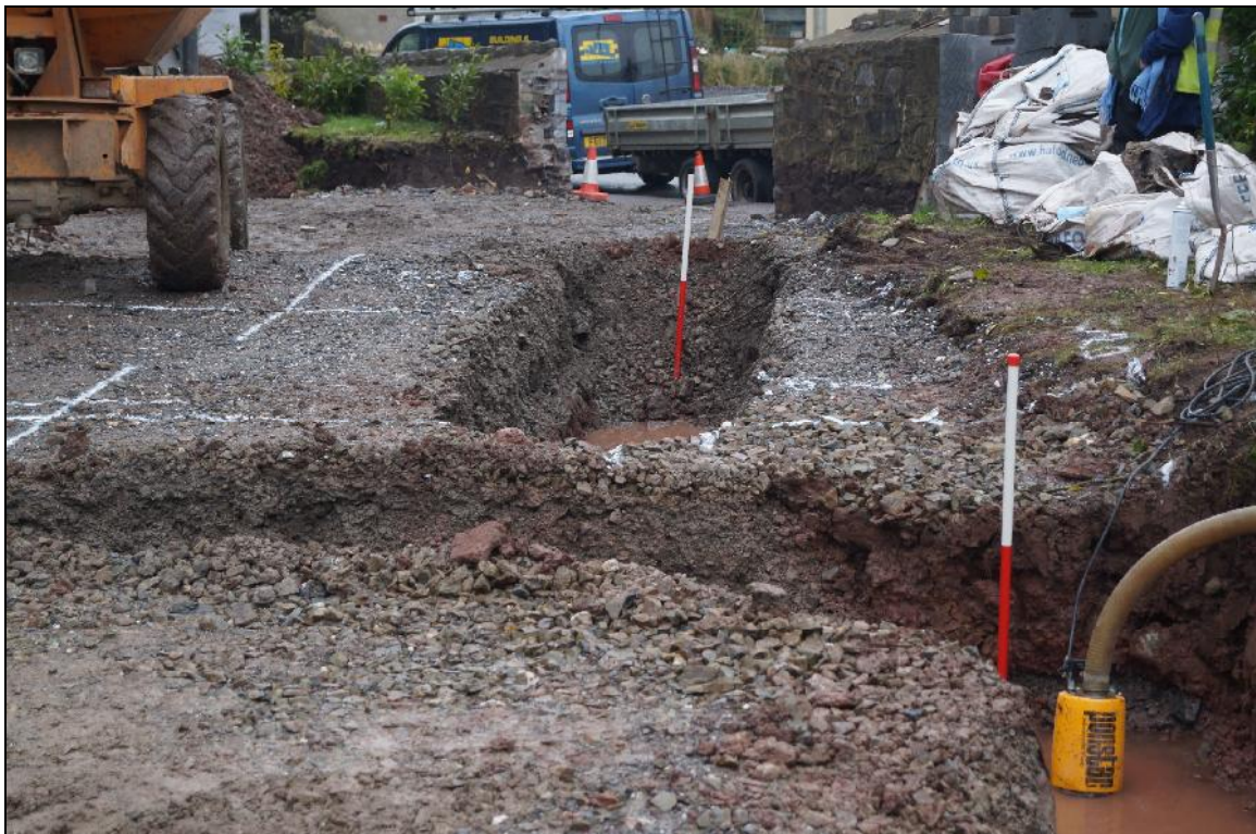
Plate 11: RCL2018_111, Southeastern foundation trench looking east. It can be seen that the eastern trenches cut only though scalplings.
