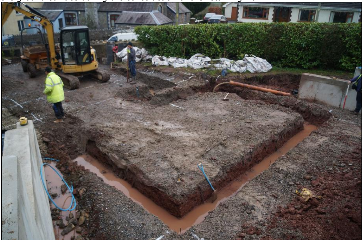
Plate 8: RCL2018_108, From the top of the retaining wall to the west looking south-southeast. Trenches visible show subsoil (002) under the layer of scalpings deposited to firm up the ground surface during the construction of the retaining wall.
