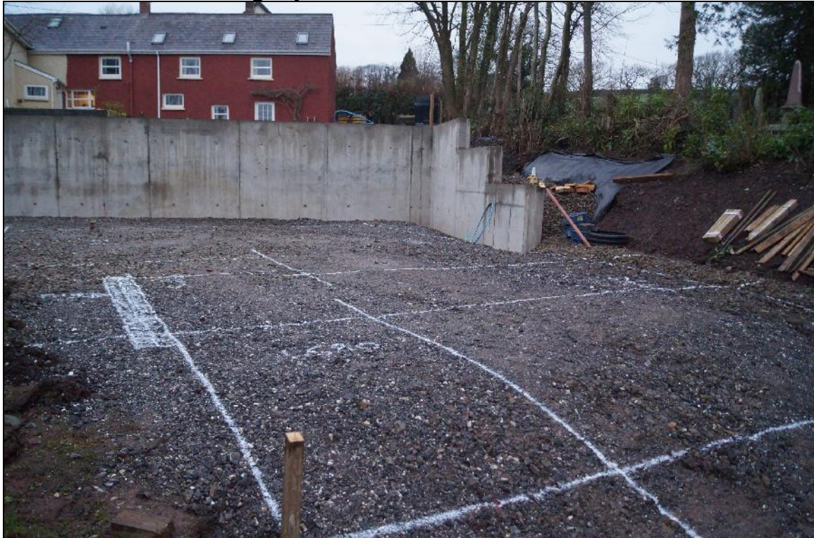
Plate 1: RCL2018_101, General view of the development area before foundation trenches excavated, looking west northwest. Previously the retaining wall, not part of the planning application, was built, and the area to its east reduced and covered in scalplings
