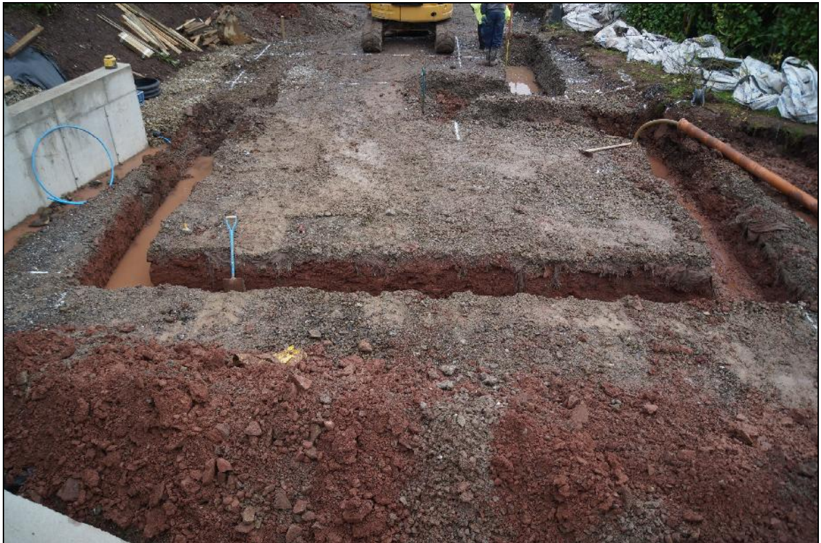
Plate 7: RCL2018_107, From the top of the retaining wall to the west, looking east. Trenches visible show subsoil (002) under the layer of scalpings deposited to firm up the ground surface during the construction of the retaining wall.
