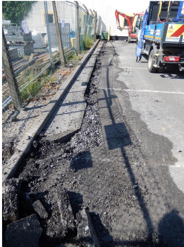
Photo 1 – Cable trench (Trench A), looking southwest towards the football club pavilion at commencement of excavation
