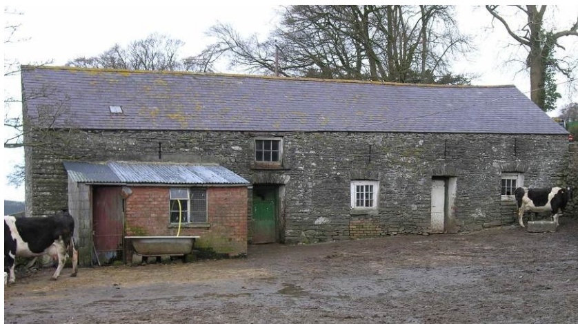
Fig 23. Five-door cow house at Broncaradog (Ystrad Meurig). Two doorways later became windows and a cool house was added in the mid twentieth century.
