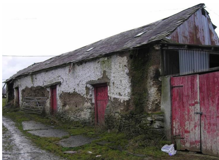
Fig 53. Earth-walled cow house at Cefn Coed (Llangeitho).
