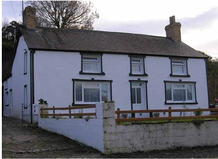
Fig 43. Nineteenth-century farmhouse at Pent-y-rhew (Nantcwnlle), partly clom built.
