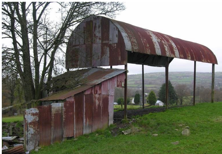
Fig 48. Corrugated-iron Dutch barn at former Hendre Las farm (Llanfihangel Ystrad).
