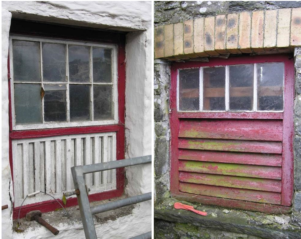
Fig 24. Sliding and louvered wooden vents in cow house windows.
