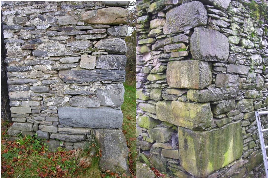
Fig 40. Field stone with large roughly squared quoins at Frith Wen (Nantcwnlle) and on a barn of 1853 at Llwyn-y-gog (Ystrad Meurig)
