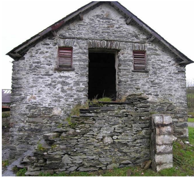
Fig 32. Granary entrance above cart shed at Cwmnewydion Isaf (Trawsgoed), retaining original louvered vents.
