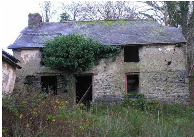
Fig 44. Nineteenth-century house at Lletty-du Uchaf (Llangeitho), the upper storey of which is clom.
