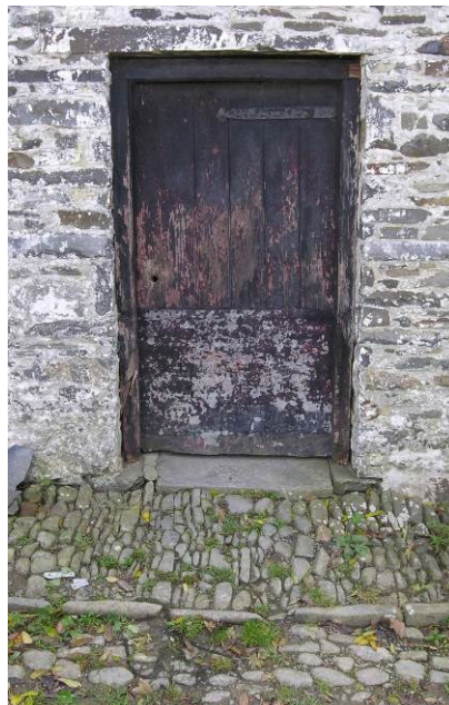
Fig 15. Cobbled surface, with kerb stones, outside a cow house.
