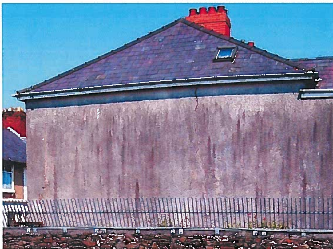
Plate 8: Subsidence crack in the wall of a property, immediately east of Area I
