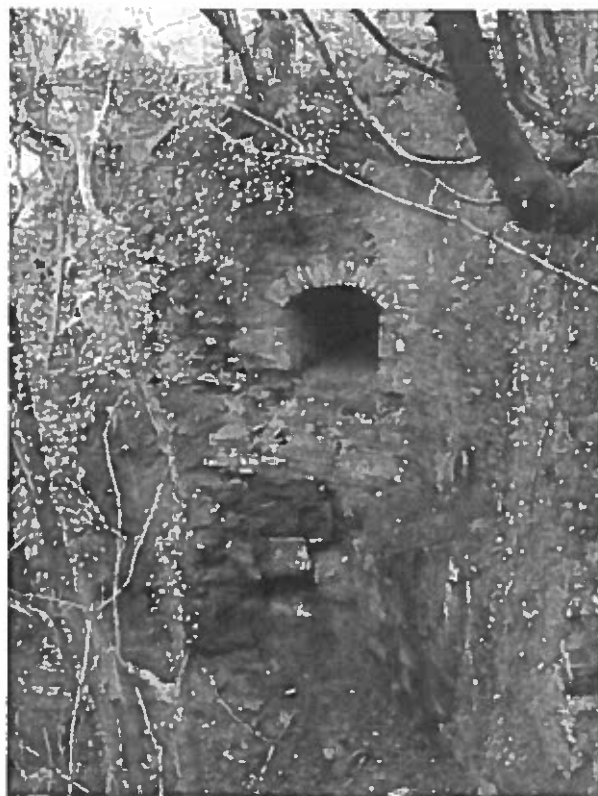
Illus 4 North-facing photograph showing overflow culvert and damage in eastern corner of downstream face of dam
