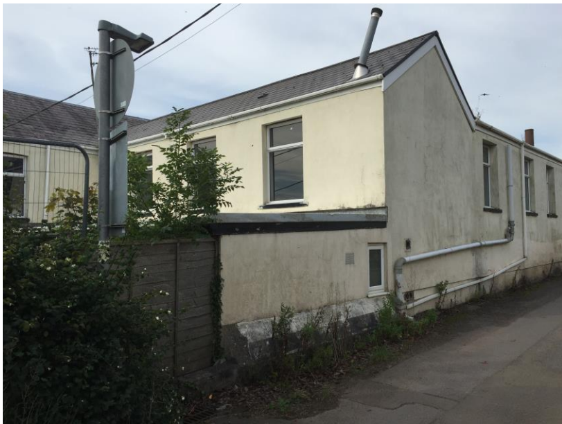
Photo 8 – south-east corner – modern flat roof toilet block to roadside with first floor former hotel accommodation over, comprising white framed upvc windows, cement tiled roof and plastic rainwater goods
