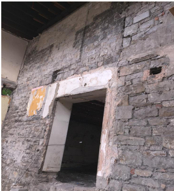
Photo 22 – example of walling with plaster ripped off to expose stone work. Simple concrete lintel above supporting opening
