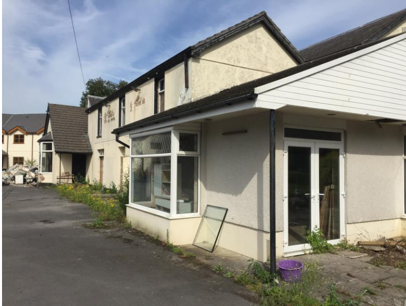
Photo 1 – south-west corner – the central entrance porch as shown in Figure 4 has been completely removed. The south-western corner comprises a modern addition with large upvc framed bay windows.
