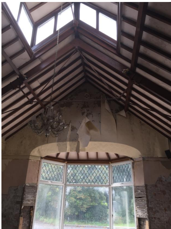
Photo 20 – view within ground floor dining room, illustrating bay window with modern replacement upvc frame. Vaulted ceiling with modern skylight, which projects above original roof ridge. Modern exposed roof trusses, stained for decorative effect
