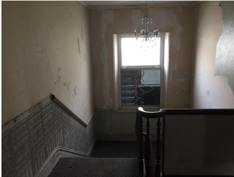
Photo 26 – first floor landing illustrating stairwell with simple moulded treads, painted metal bannisters and stained timber handrail. Decorative wallpaper to original plater elements with modern plaster overlaid above.
