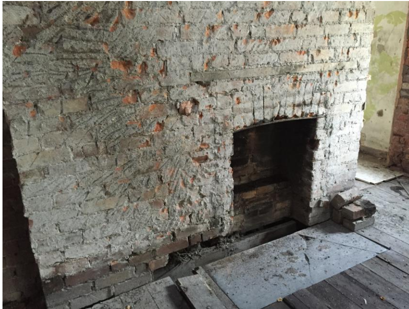
Photo 28 – fireplace exposed within former hotel bedroom, comprising simple engineering brick surround, with thin, narrow flue to roof chimney
