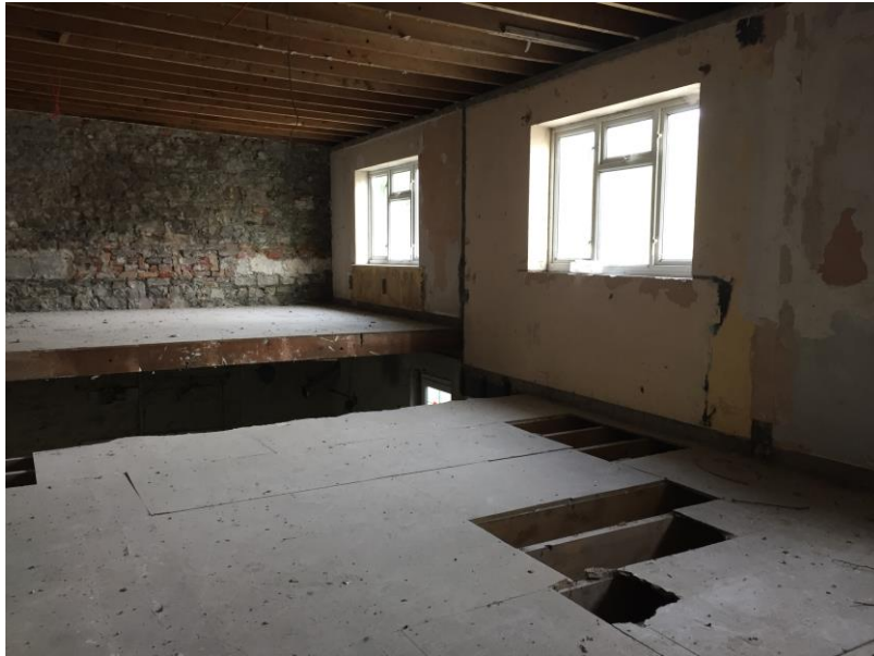
Photo 30 – rear elevation to roadside with floor boards exposed and modern window additions.
