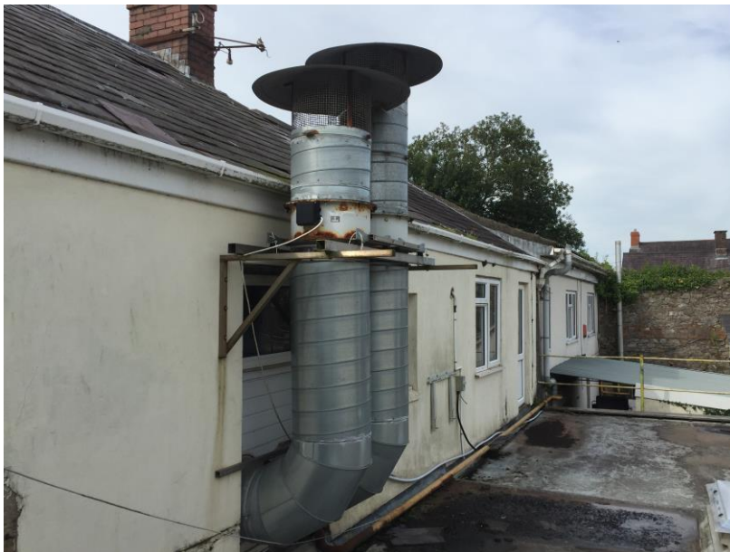
Photo 10 – flat roof over function room, illustrating modern skylights and extraction flues from ground floor kitchens. Former rear of old Gwenllian totally re-modelled with modern windows in white upvc frames
