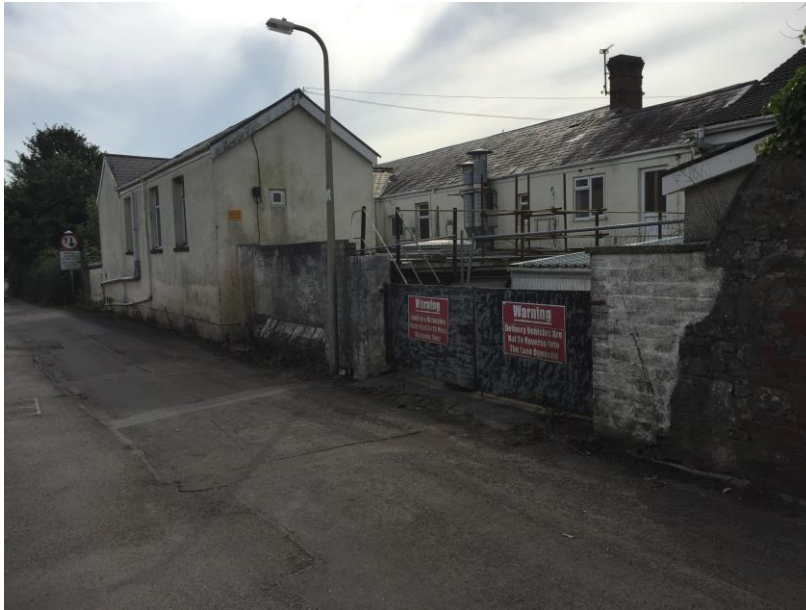
Photo 9 – north-east corner – modern extensions to rear of property, with flat roof over function room, and concrete block walls enclosures to service entrance.
