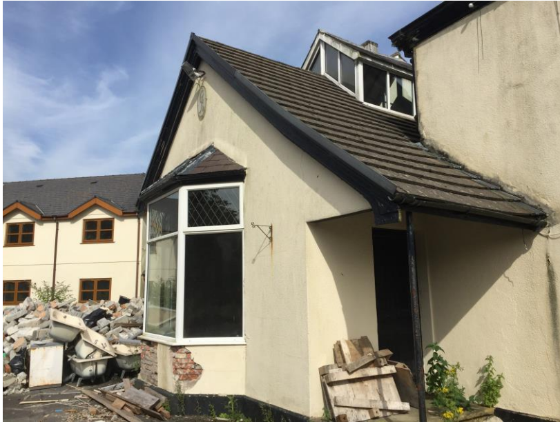
Photo 3 - west elevation – modern bay window extension, with modern roof light, constructed of white upvc frame, with concrete roof tile
