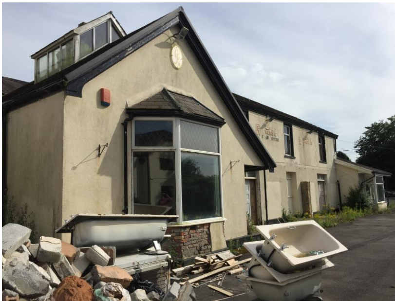
Photo 4 – north-west corner - modern bay window extension, with modern roof light, constructed of white upvc frame, with concrete roof tile
