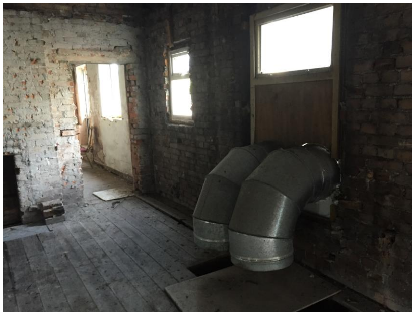
Photo 29 – first floor elevation disrupted by insertion of extraction flues.
