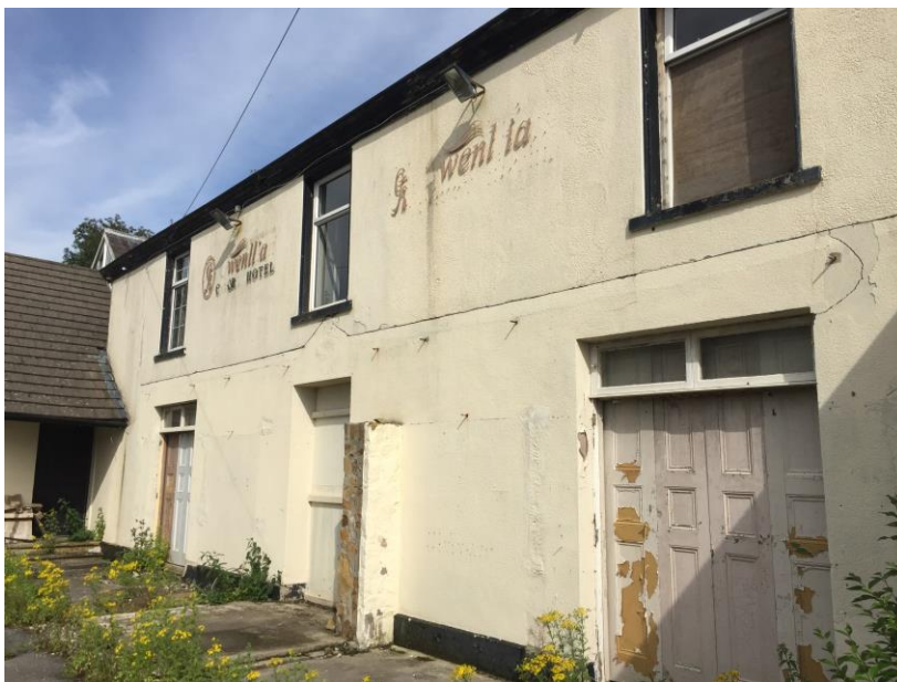
Photo 2 – west elevation – openings have been board up with temporary materials, as have fanlights above.
