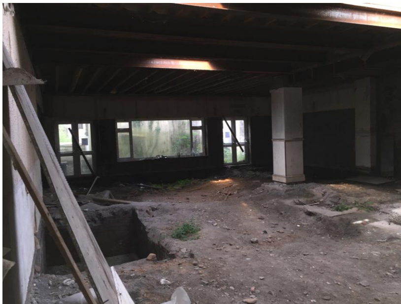
Photo 18 – remains of function rooms with floors removed, exposing modern support pillars.
