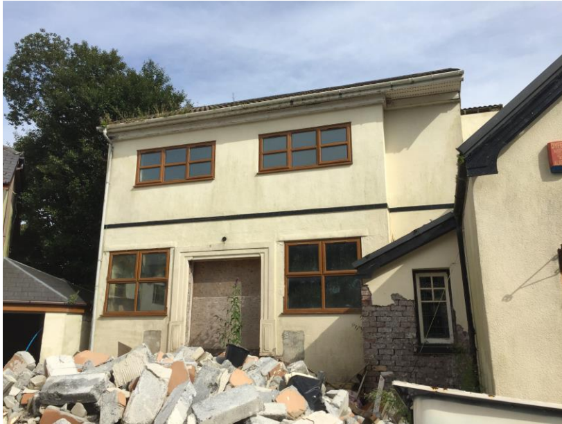
Photo 5 – north elevation – illustrating modern brown framed upvc windows at both floors with modern double doorway, temporarily blocked up. The former entrance steps and walling has been removed from that displayed in Figure 3.
