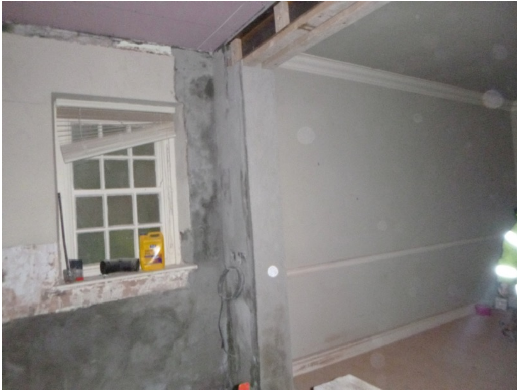
Photograph – view of east wall – cement based plastering can be seen
