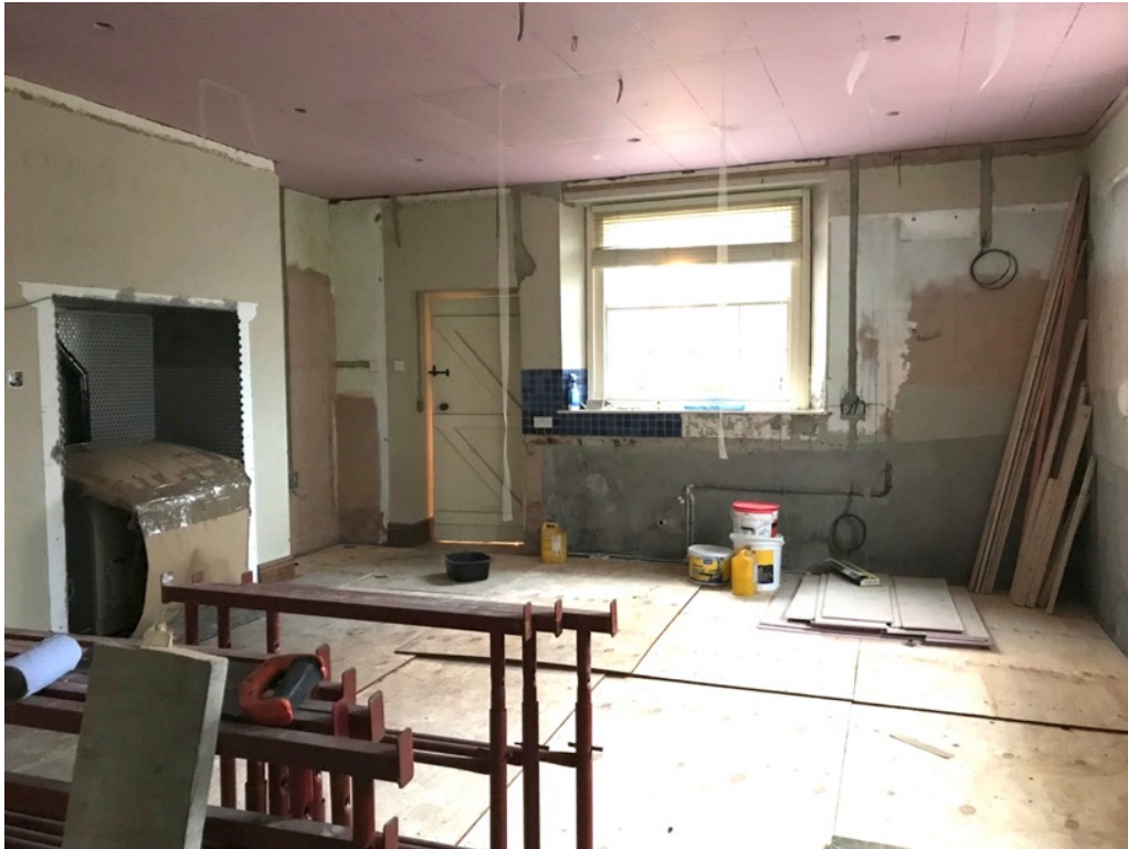
Photograph - View of kitchen. Patches of cement based plastering can be seen
