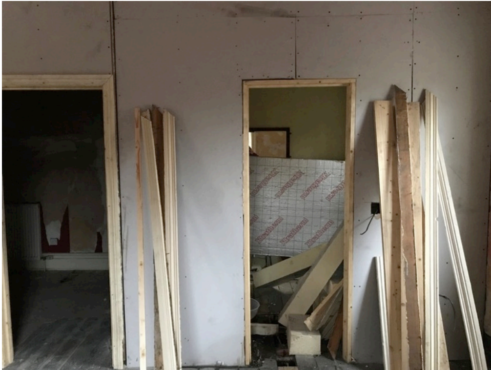
Photograph – View of new plasterboard laid to partition. Existing stud partition from centre door to wall with window
