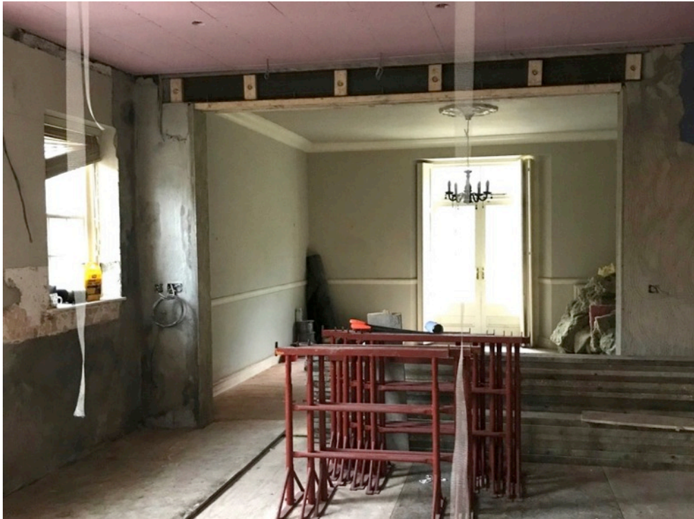
Photo – New opening created in wall between sitting room and kitchen
