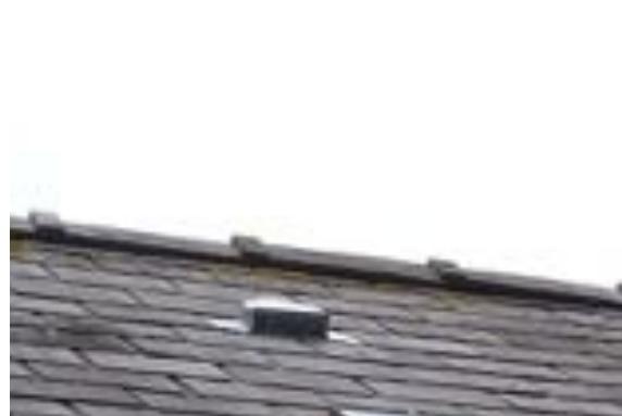
Above: Lead cowl fitted to main house north roofslope serving bathroom
