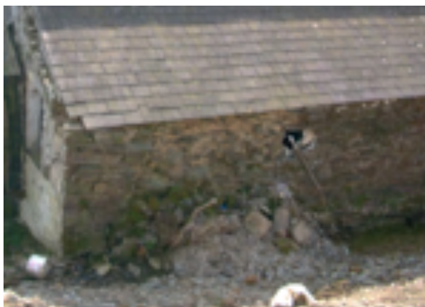
Above: local masonry collapse post excavation
