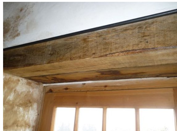
Above: Typical examples of timber lintels replaced with oak lintels used internally and oak lining added to conceal concrete lintels to wall core.
