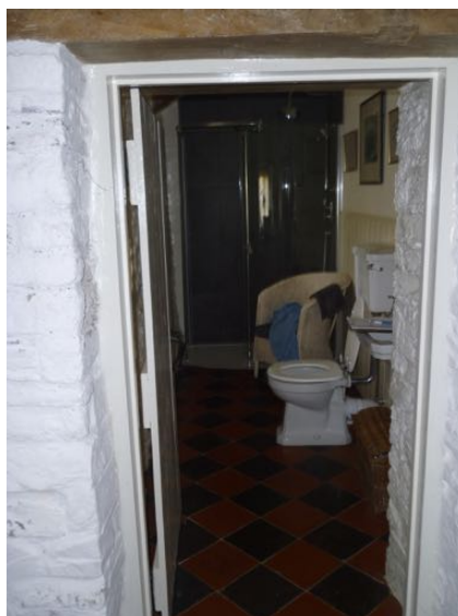
Above: New limewash to stone and localised tiling behind shower to lean-to shower room
