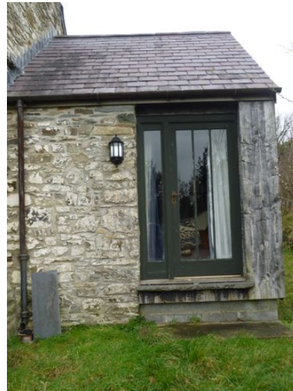
Above: New study room glazed door to south elevation of east extension. Consented pair of doors changed to single door with fixed side light
