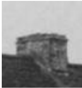
Above: Blain-llain, Llanwenog, Ceredigion with squared rubble course above roofing slate course
