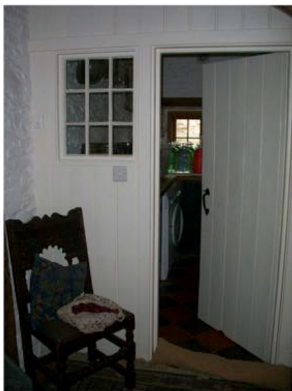
Above: New utility room partition reusing the window and boarding opposite in painted finish
