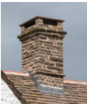
Above: Recently restored chimney with raised slab detail at Llwyn celyn, Monmouthshire within Brecon Beacons National.
