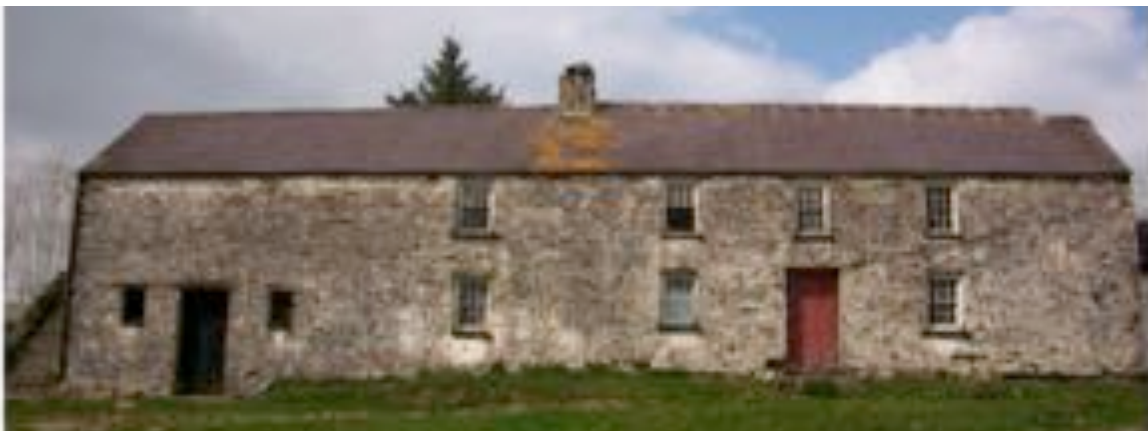
Above: Pre-development south elevation. Sash windows replaced like for like with solid boarded doors modified with addition of small vision panes. Former stable openings with single timber shutter (left) replaced with glazed four pane side hung casements.
