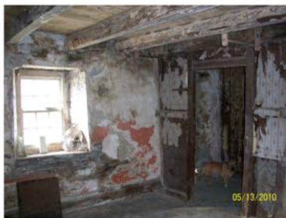
Above: Existing finishes with limewash over plaster, painted and varnished joinery with partial wall paper over partition. Note poor condition
