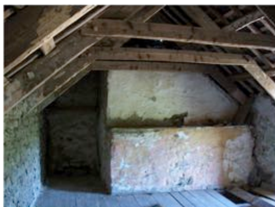
Above: Existing limewashed and bare stone finishes in poor condition and absent ceiling but decoration visible to bottom of rafters
