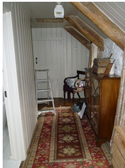
Above: New painted timber boarding to new partitions on first floor hallway
