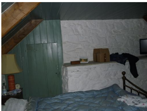
Above: Original boarding to cupboard door refitted and decorated in bedroom with limewash to stone
