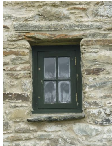
Above: New kitchen window to south elevation of former stable (two in total). Consented single panel changed to four panes.
