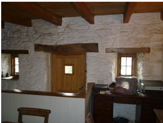
Above: Typical examples of timber lintels replaced with oak lintels used internally and oak lining added to conceal concrete lintels to wall core.
