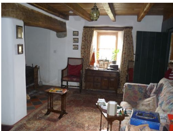
Above: Limewash over lime plaster
