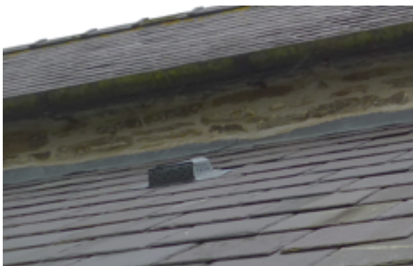
Above: Lead cowl fitted to north lean-to roofslope serving shower room
