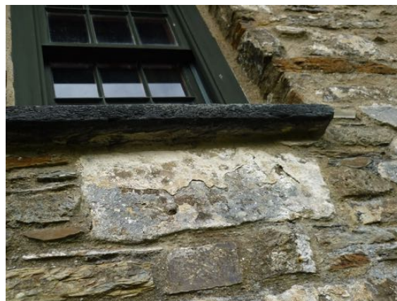
Above: Limewash adhered to bigger stone with loss over smaller stones
