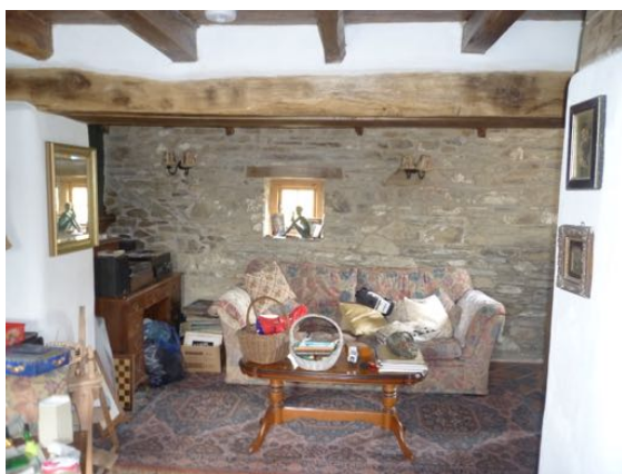
Above: Localised area of exposed stonework pointed in lime to north wall of lean-to area now within sitting room
