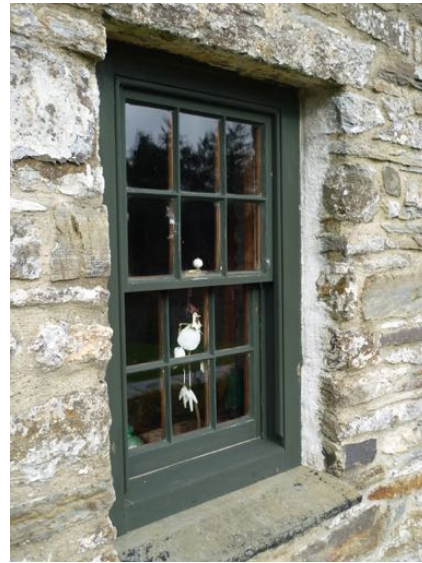
Above: Typical new sash window to south elevation of house (eight in total)
