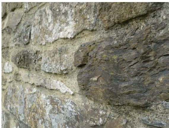
Above: Traces of limewash with complete loss over shaley stone surfaces
