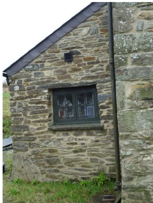
Above: Cast iron air brick fitted to west elevation serving utility room
