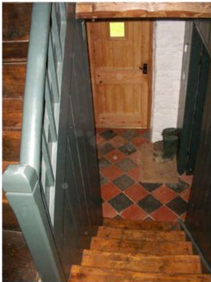
Above: As built varnished and painter joinery finishes to stairwell
