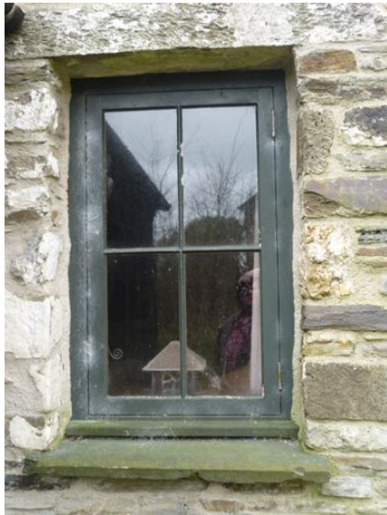
Above: New sitting room window to east elevation of lean-to with window reduced to single casement and four panes to fit original opening
