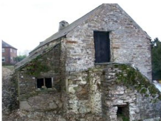
Left: Pre-development west elevation to lean-to and stable with open frame to lean-to window and fully boarded door
