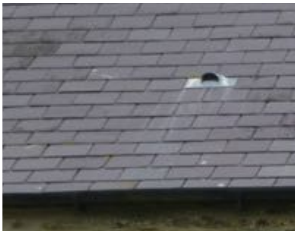
Above: Lead cowl fitted to south roofslope serving ensuite
