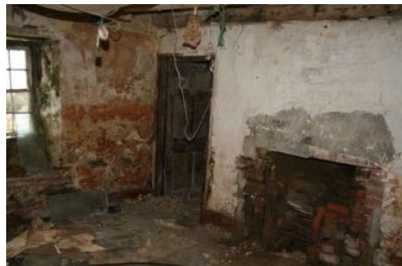
Above: Existing limewash and painted joinery showing condition with patch cementitious repairs, spalling, aglae around windows and peeling limewash
