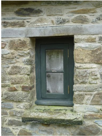
Above: New shower room window to north elevation of lean-to with glazing reduced to two panes to fit original opening (former salting room)
