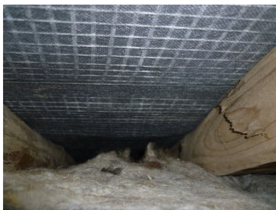
Below: View of the roof void in 2019 with roof timbers, felt and insulation in good order
