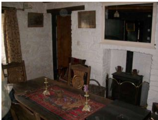
Above: Limewash finish over stone and painted joinery
