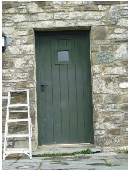
Above: New house entrance door to south elevation (stable door similar). Consented four panel door changed to boarded door to matching existing. Small glazed vision panel added.
