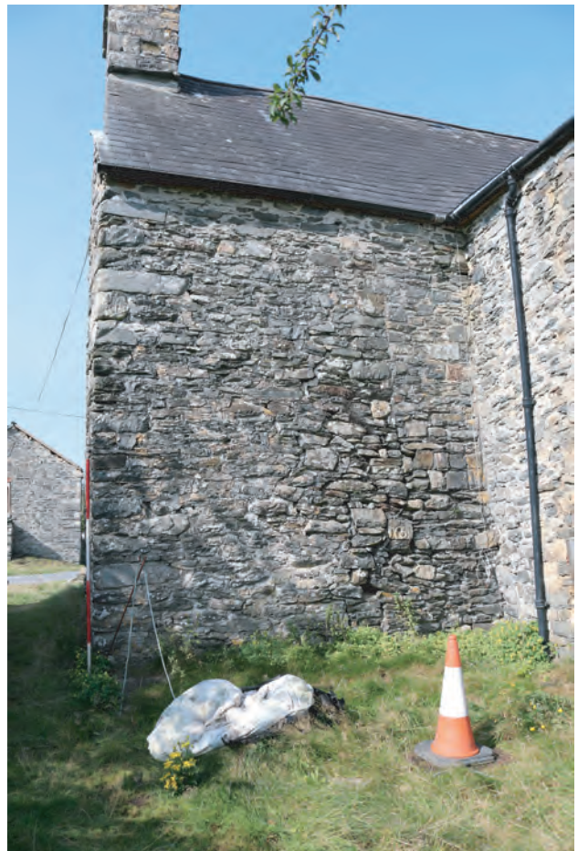
Plate 10(c). Far southern end of east wall of Mynachlog Fawr showing numerous features including apparent line of former tall window.
