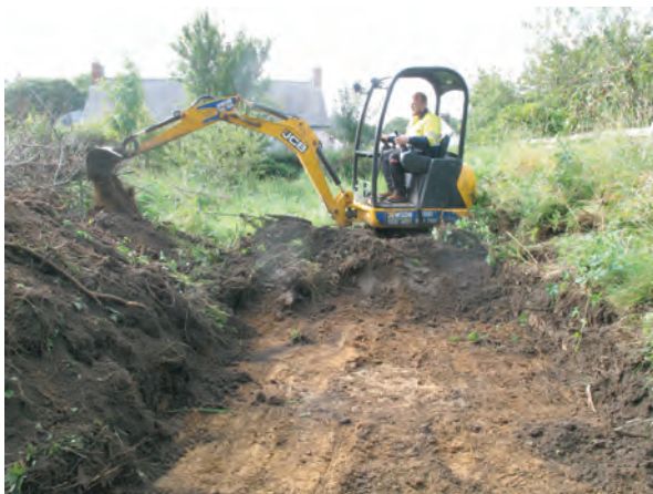
Plate 9. Working shot during turf and top soil clearance. Looking southwards.
