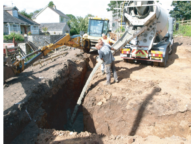
Plate 14. Working shot during concrete delivery to back fill post medieval pit. Looking northwards.
