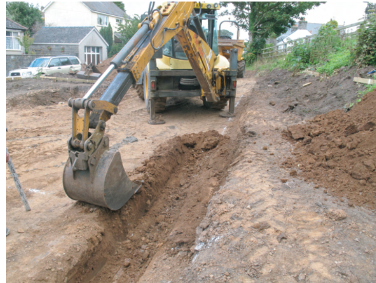
Plate 16. Working shot during continued foundation trench cutting. Looking northwards.
