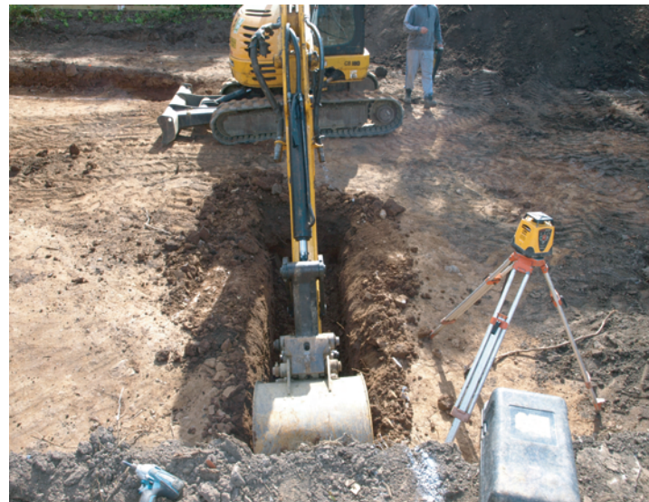
Plate 10. Working shot during cutting of foundation trench. Looking eastwards.
