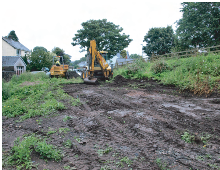
Plate 4. Working shot during turf and top soil stripping. Looking northwards.
