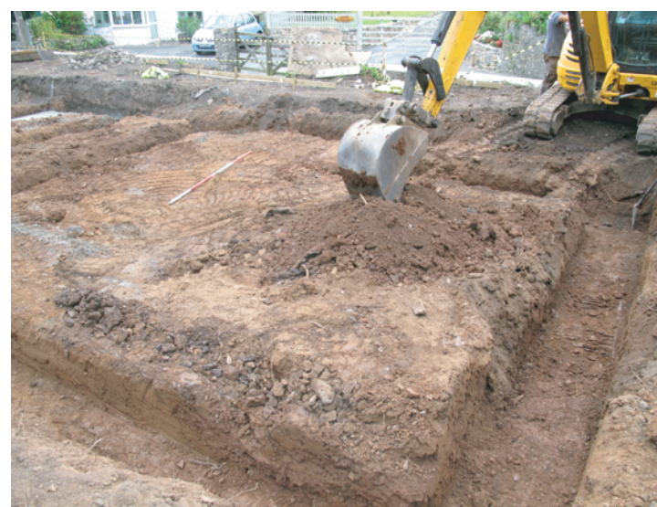
Plate 24. Completed groundwork for foundation cutting. Looking southwest.
