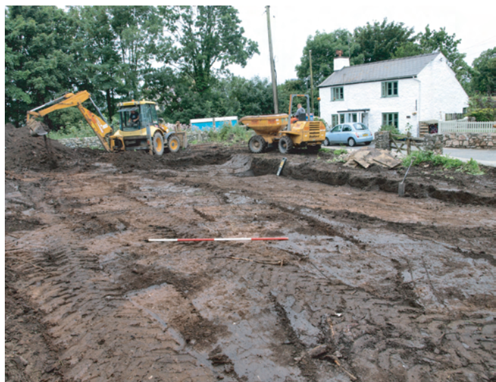
Plate 7. Area of proposed development following turf and top soil strip. Looking southwards.
