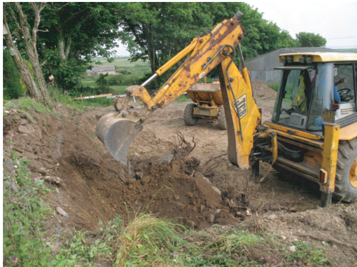
Plate 5. Working shot during ground reduction and top soil strip. Looking east.
