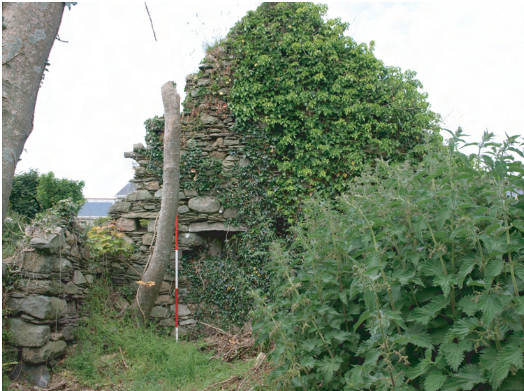
Plate 25. View of Hospitium remains prior to any clearance and consolidation work. Internal east facing gable end. Note blocked in niche and put-log hole. Looking west.
