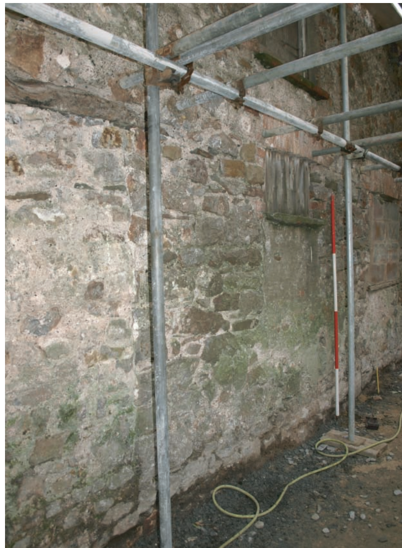
Plate 16. View of external north facing elevation of storage building No.1. Note blocked in former doorways. Looking west.
