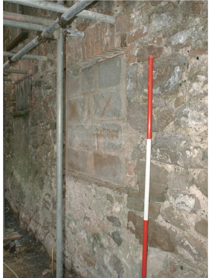
Plate 22. Former window detail (former doorway) in external north facing elevation of storage building No.1. Looking south.
