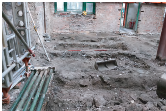
Plate 119. The Old Coal Office, Saundersfoot. 19th Century floor support piers within building following ground reduction.
