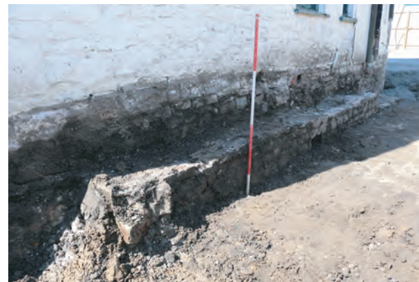
Plate 101. The Old Coal Office, Saundersfoot. Detail of exposed earlier foundation at base of north facing elevation.
