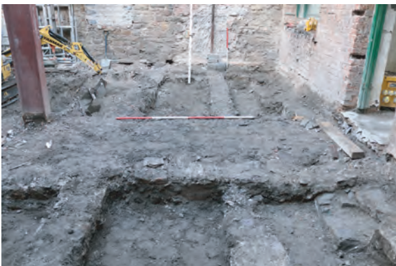
Plate 117. The Old Coal Office, Saundersfoot. 19th Century floor support piers within building following ground reduction.
