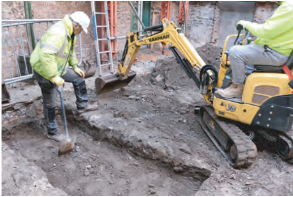
Plate 113. The Old Coal Office, Saundersfoot. Working shot during floor reduction.
