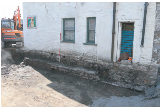
Plate 100. The Old Coal Office, Saundersfoot. Detail of exposed earlier foundation at base of north facing elevation.
