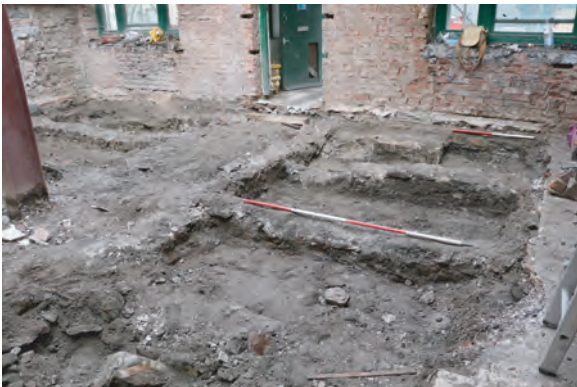
Plate 115. The Old Coal Office, Saundersfoot. 19th Century floor support piers within building following ground reduction.
