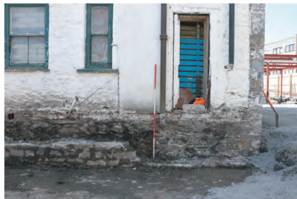
Plate 102. The Old Coal Office, Saundersfoot. Detail of exposed earlier foundation at base of north facing elevation.
