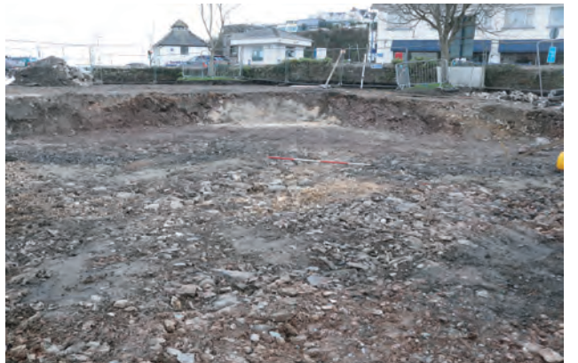
Plate 93. The Old Coal Office, Saundersfoot. Completed ground reduction work at southeast end.
