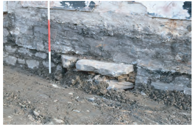
Plate 89. The Old Coal Office, Saundersfoot. Apparent blocked entrance at base of west facing elevation. Likely former coal storage basement
