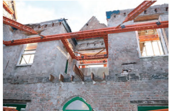
Plate 108. The Old Coal Office, Saundersfoot. Internal view of east wall during floor removal.
