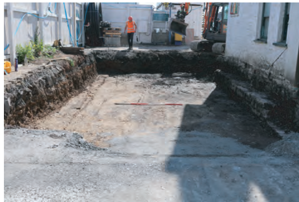
Plate 97. The Old Coal Office, Saundersfoot. Completed ground reduction work in area of north facing elevation of coal office.
