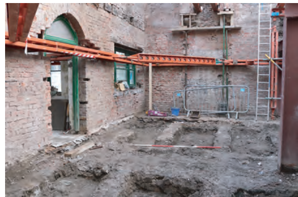
Plate 118. The Old Coal Office, Saundersfoot. 19th Century floor support piers within building following ground reduction.
