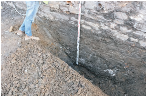
Plate 88. The Old Coal Office, Saundersfoot. Inspection slot against west facing elevation to investigate depth of foundation for engineering purposes.
