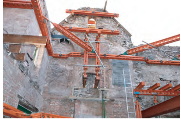
Plate 106. The Old Coal Office, Saundersfoot. Internal view of south wall during floor removal.
