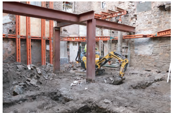
Plate 114. The Old Coal Office, Saundersfoot. 19th Century floor support piers within building following ground reduction.
