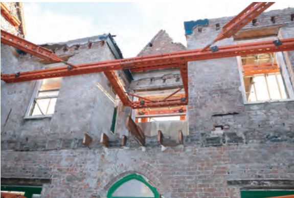
Plate 109. The Old Coal Office, Saundersfoot. Internal view of east wall during floor removal.
