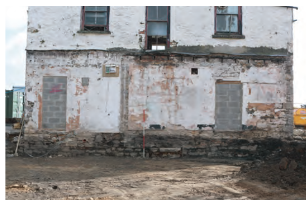
Plate 85. The Old Coal Office, Saundersfoot. West facing elevation of coal office following shopfront demolition and ground reduction.
