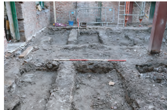
Plate 116. The Old Coal Office, Saundersfoot. 19th Century floor support piers within building following ground reduction.
