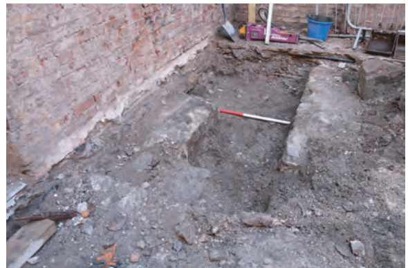
Plate 112. The Old Coal Office. Floor support piers exposed during ground reduction work within interior of coal office.
