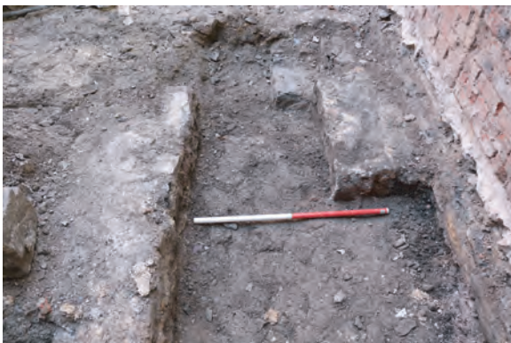
Plate 111. The Old Coal Office, Saundersfoot. Floor support piers exposed during ground reduction work within interior of coal office.
