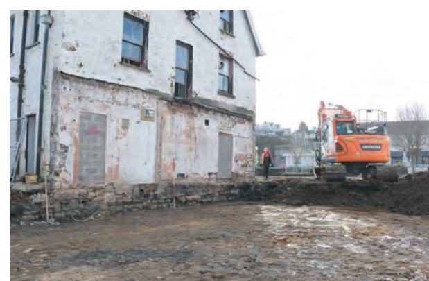
Plate 87. The Old Coal Office, Saundersfoot. West facing elevation of coal office following shopfront demolition and ground reduction.
