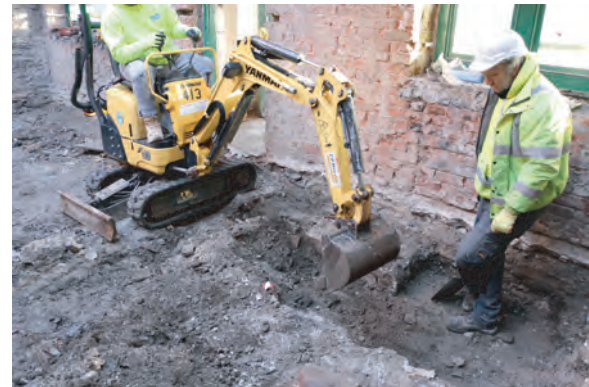
Plate 110. The Old Coal Office, Saundersfoot. Working shot during floor reduction within interior. East end.
