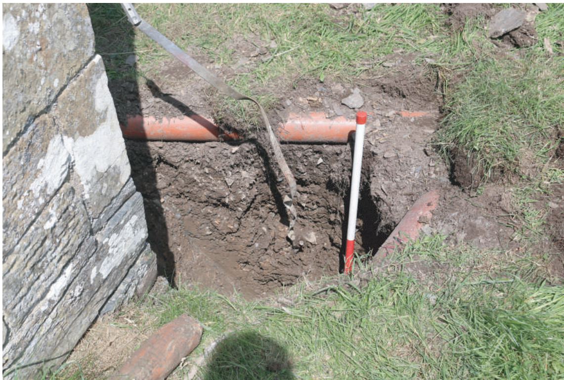
Plate 30. St. David's Church, Blaenporth - Completed Trench for Lightning Conductor Plate 2 at eastern corner of church. Looking N.
