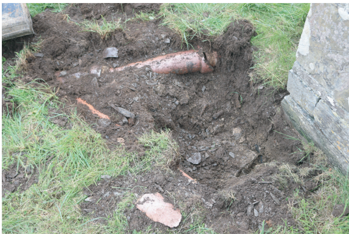
Plate 29. St. David's Church, Blaenporth - Working shot during cutting for Lightning Conductor Plate 2. Note 1930s/50s stone drainage pipe. Looking E.
