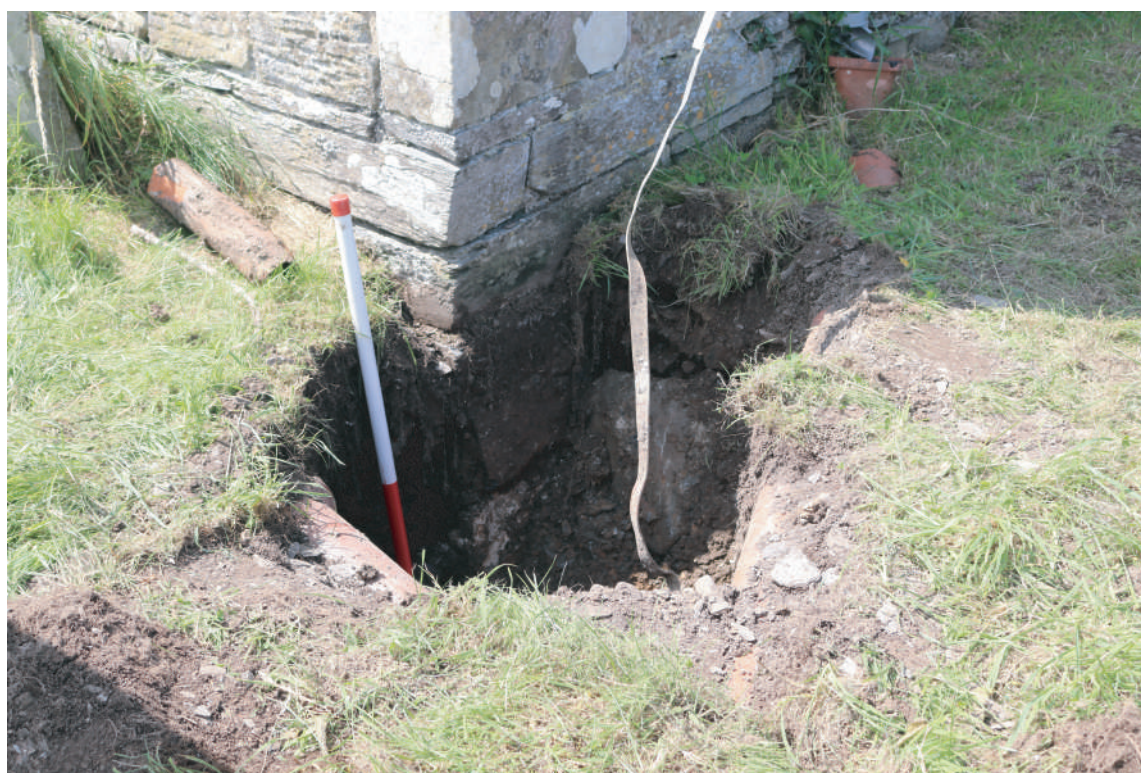
Plate 31. St. David's Church, Blaenporth - Completed Trench for Lightning Conductor Plate 2 at eastern corner of church. Looking SW.
