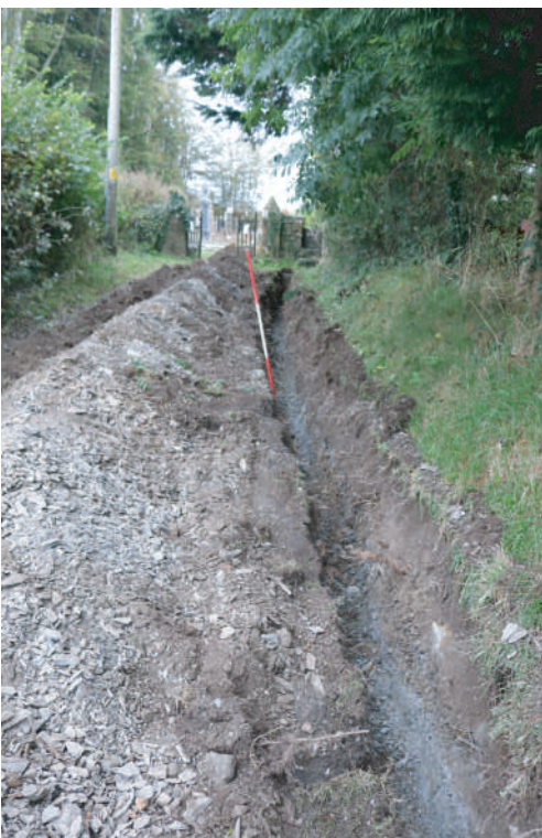
Plate 22. St. David's Church, Blaenporth - View of completed cut trench for proposed water pipe outside of cemetery entrance. Looking N.
