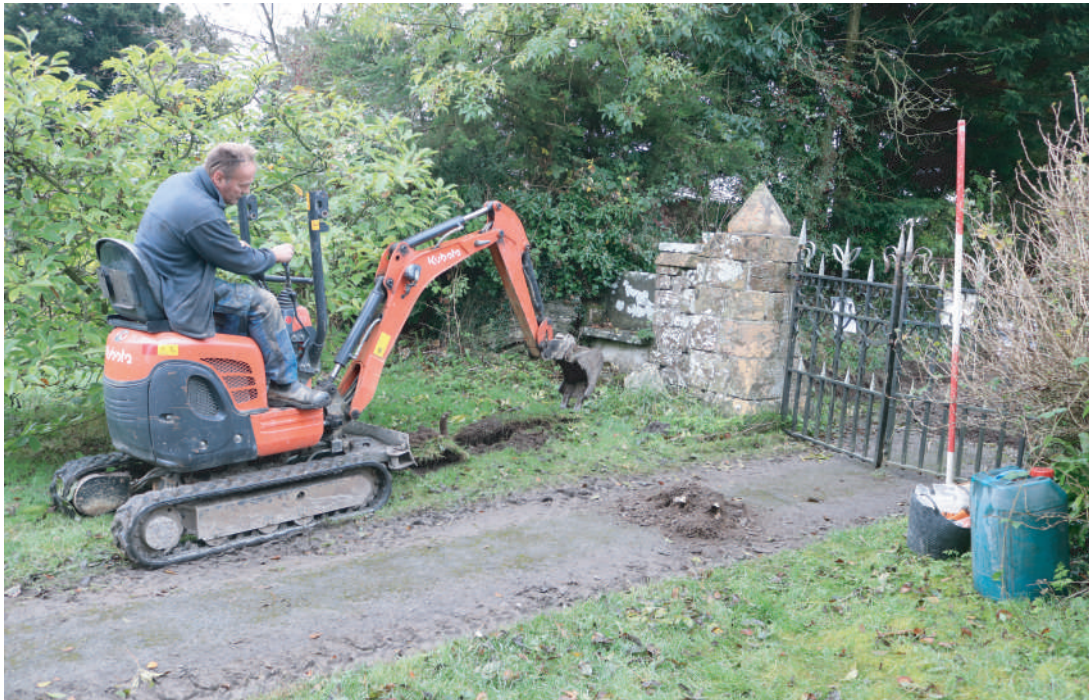
Plate 17. St. David's Church, Blaenporth - Working shot during initial cutting of water service trench at entrance of cemetery. Looking SE.
