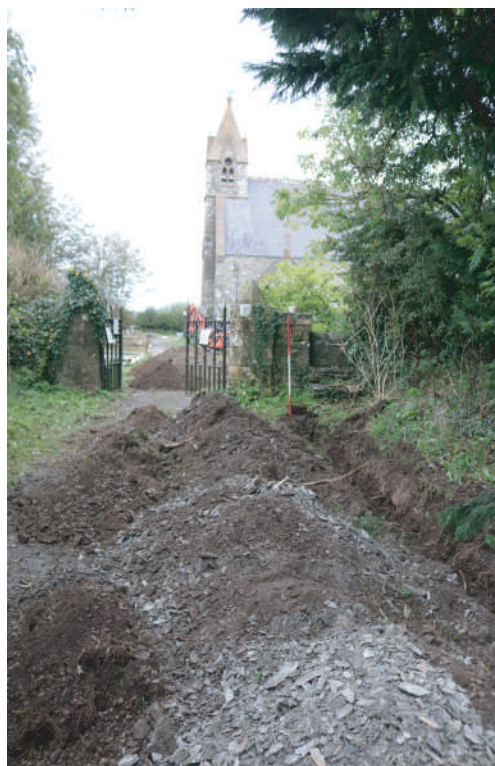
Plate 21. St. David's Church, Blaenporth - View of cut trench for proposed water pipe outside of cemetery entrance. Looking N.
