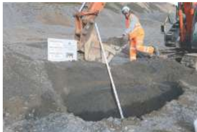
Plate 59. Machine dug Trench 21 (TP21). Trench 21 ground works completed at 1.60m due to trench sides collapsing. Looking NE.
