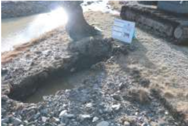
Plate 47. Machine dug Trench 14 (TP14). Groundworks completed following water ingress at only 0.40m below surface. Looking S.
