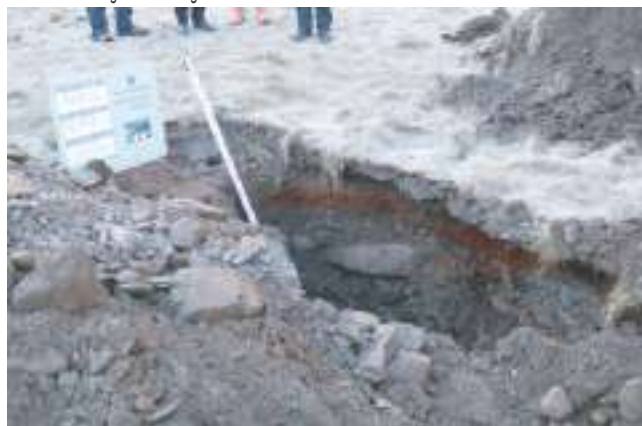
Plate 30. Machine dug Trench 11 (TP11). Trench following ground investigation works. Note orange sub base of grit for cobbled surface packing. Looking SE.
