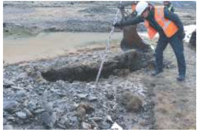
Plate 46. Machine dug Trench 14 (TP14). Groundworks completed following water ingress at only 0.40m below surface. Looking S.
