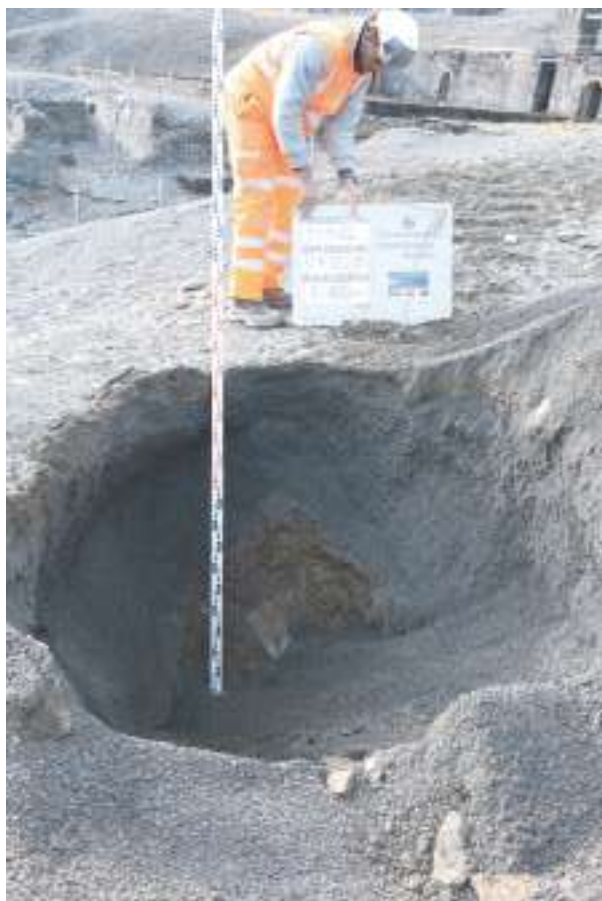
Plate 58. Machine dug Trench 21 (TP21). Trench 21 ground works completed at 1.60m due to trench sides collapsing. Looking NW.
