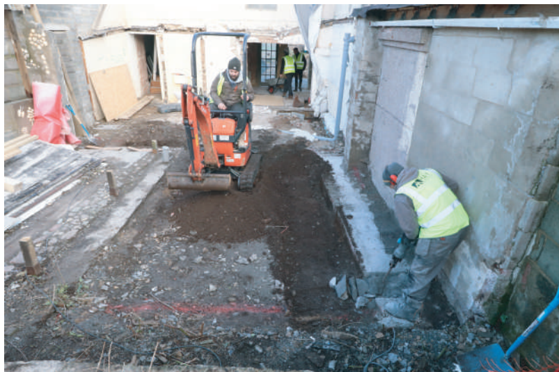
Plate 14. Stripping back of exposed ground surface at rear of Village Store following demolition of existing extensions. Looking N.
