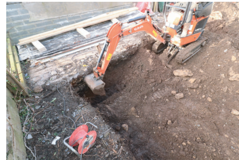
Plate 21. Working shot during cutting of foundation trench alongside culverted stream. Looking NW.
