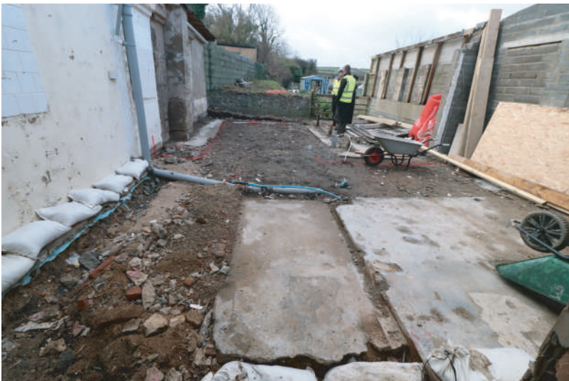
Plate 07. View of rear area of Village Store following demolition of former extensions and marking out of foundation trenches. Looking southward.
