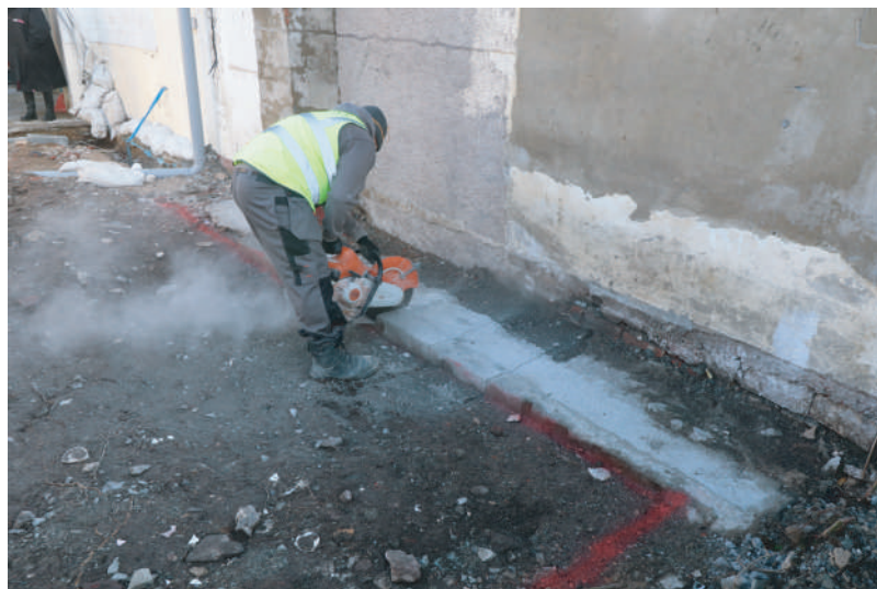
Plate 12. Working shot during cutting of concrete on east side of proposed garden area in order to initially create foundation trench. Looking NE.
