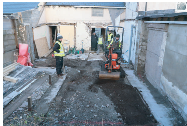
Plate 13. Stripping back of exposed ground surface at rear of Village Store following demolition of existing extensions. Looking N.
