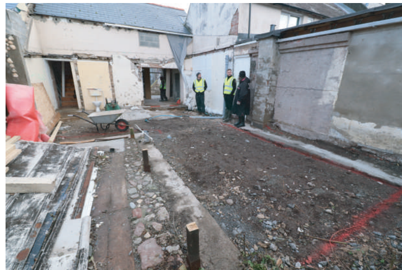
Plate 06. View of rear elevation of Village Store following demolition of former extensions and marking out of foundation trenches. Looking northward.
