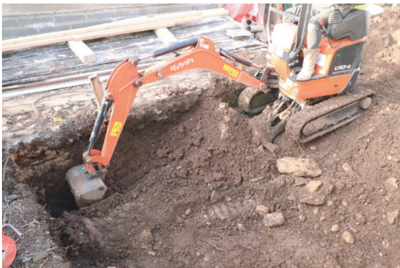
Plate 20. Working shot during cutting of foundation trench alongside culverted stream. Looking NW.
