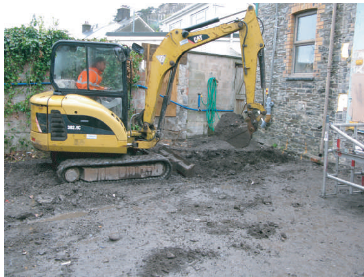
Plate 15. Working shot during cutting for service trench. Looking westwards.
