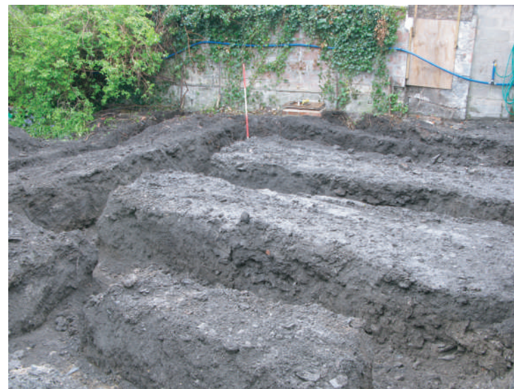
Plate 25. Completed foundation trenches. Looking westward.
