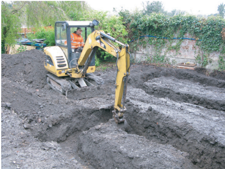
Plate 21. Working shot during cutting of service trench. Looking southwest.
