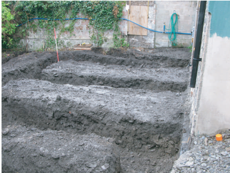
Plate 26. Completed foundation trenches. Looking westward.
