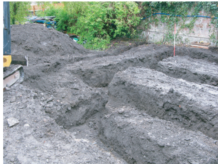
Plate 24. Completed foundation trenches. Looking southwest.
