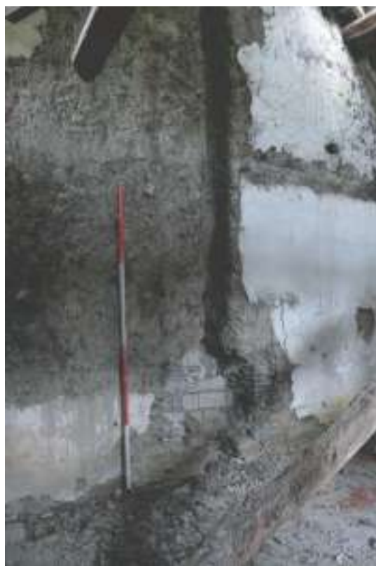
Plate 43. Remains of Rhosygraigina cottage. Interior view of former fireplace with flue incorporated into mud wall in north wall of Parlour/Bedroom. Looking northeast.
