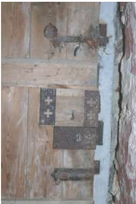
Plate 47. Remains of Rhosygraigina cottage. Interior detail of front door locks. Looking east.
