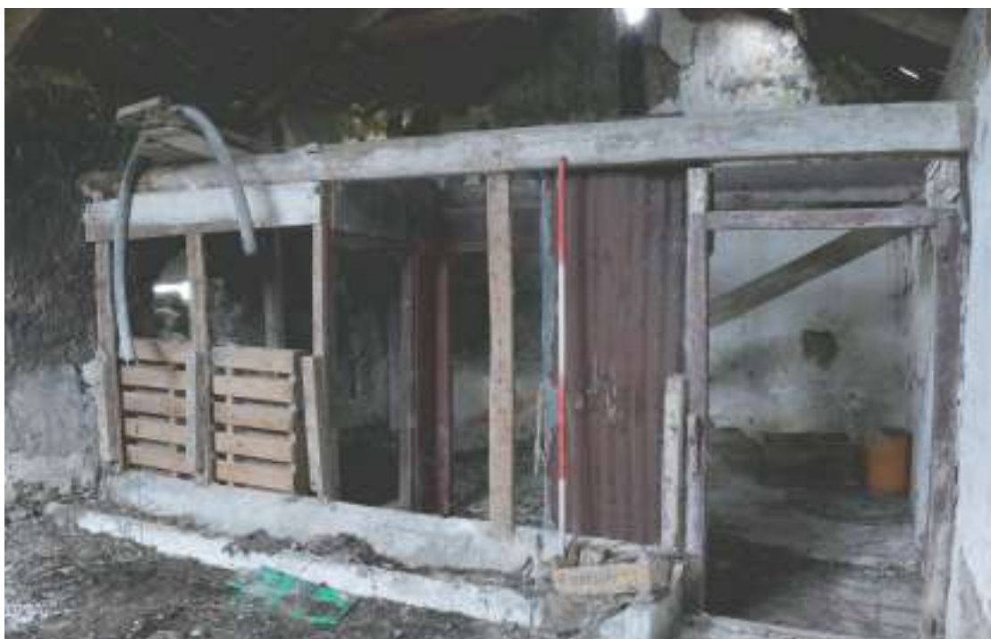
Plate 34.. Remains of Rhosygraigina cottage. Interior view of partition between Living Room/Kitchen and Parlour/Bedroom. Looking northward.
