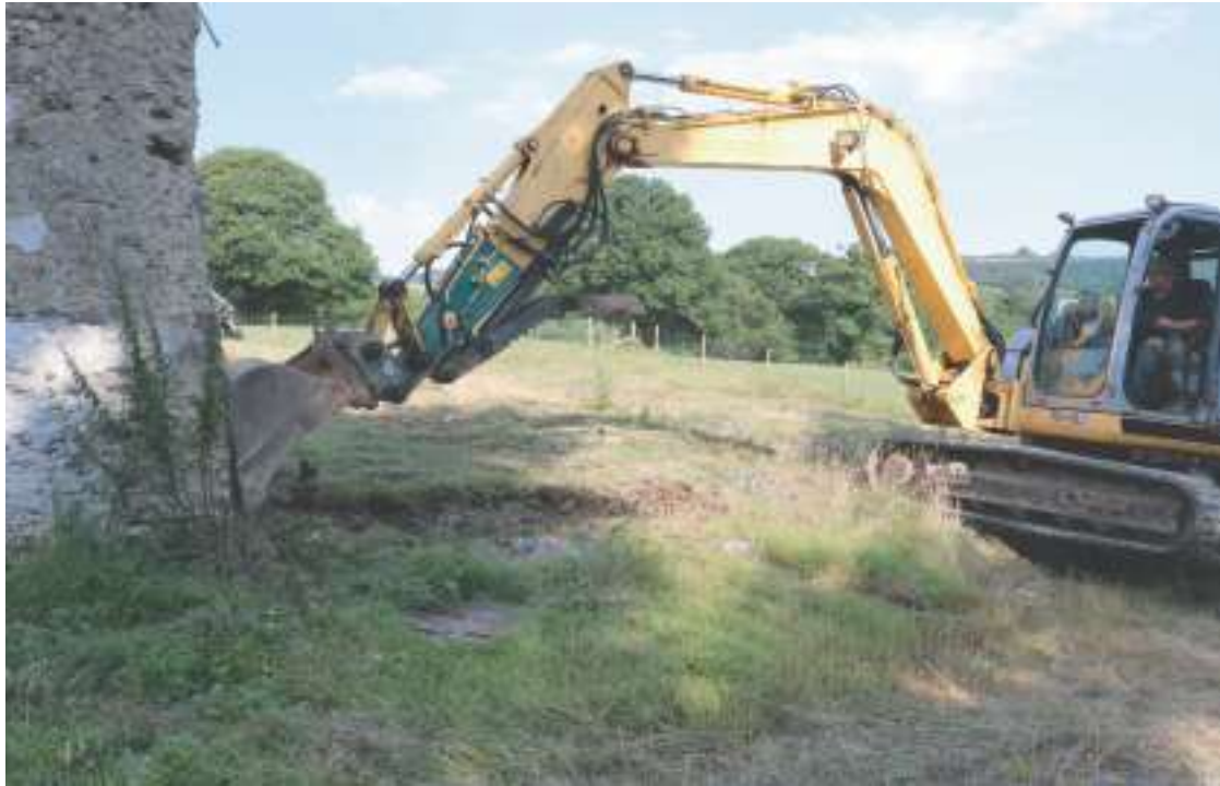
Plate 54. Rhosygraigina cottage - Working shot during foundation cutting for proposed extension at north end of cottage. Looking W.
