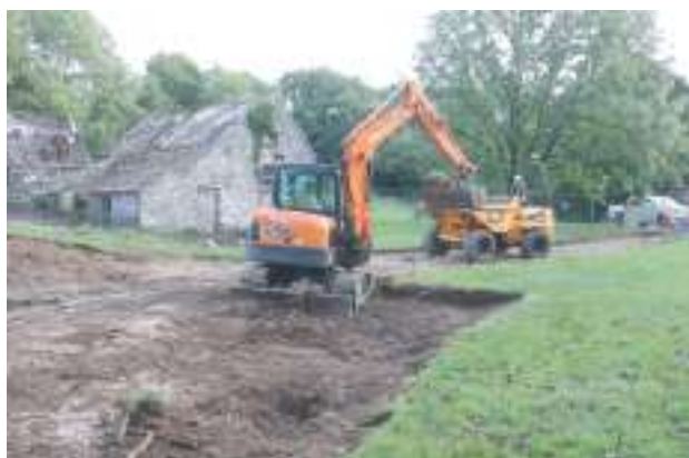
Plate 57. Canolfan yr Urdd, Pentre Ifan - Working shot during stripping of turf and top soil. Looking NE.
