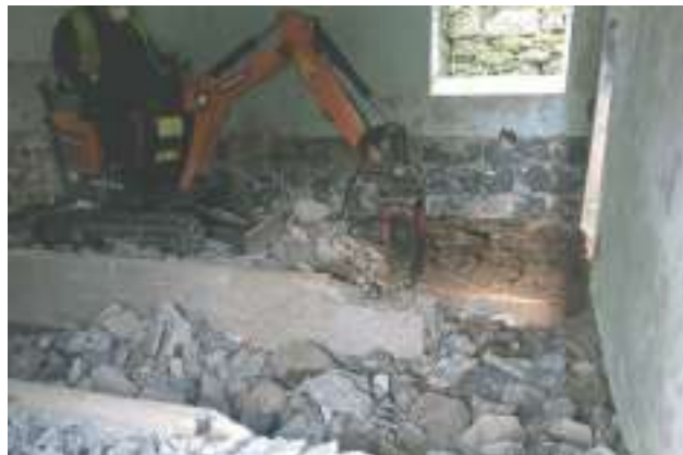
Plate 71. Canolfan yr Urdd, Pentre Ifan - Clearance by machine of concrete floor within Milking Parlour. Looking W.
