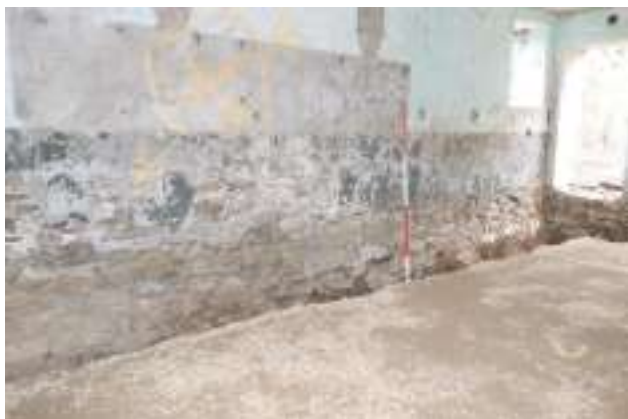
Plate 81. Canolfan yr Urdd, Pentre Ifan - Milking Parlour. Cut in floor for proposed concrete ring beam. Looking NW.
