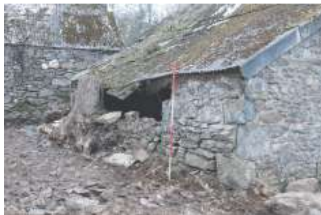
Plate 84. Canolfan yr Urdd, Pentre Ifan - Milking Parlour. View of tree stump compromising west wall following ground work. Looking N
