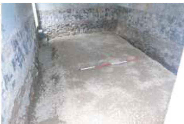
Plate 83. Canolfan yr Urdd, Pentre Ifan - Completed floor reduction and ring beam cut. Looking S.
