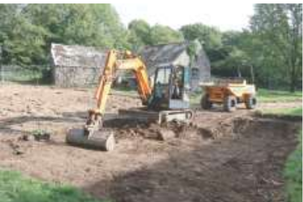
Plate 58. Canolfan yr Urdd, Pentre Ifan - Working shot during stripping of turf and top soil. Looking NE.
