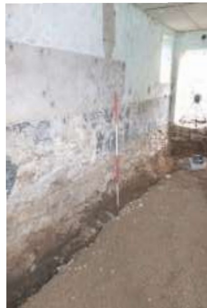
Plate 80. Canolfan yr Urdd, Pentre Ifan - Milking Parlour. Cut in floor for proposed concrete ring beam. Looking W.
