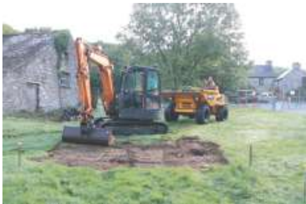
Plate 51. Canolfan yr Urdd, Pentre Ifan - Working shot during stripping of turf and top soil. Looking E.
