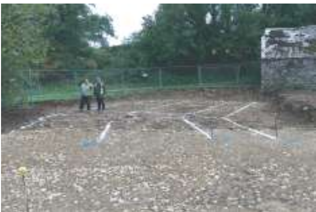
Plate 64. Canolfan yr Urdd, Pentre Ifan - Cleared area of ground marked out for foundation cutting. Looking N.
