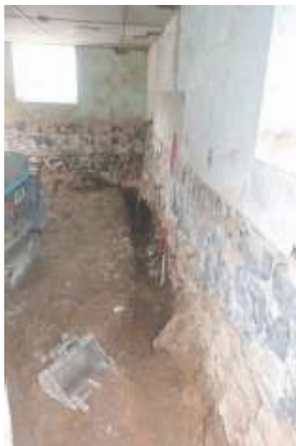
Plate 79. Canolfan yr Urdd, Pentre Ifan - Milking Parlour. Cut in floor for proposed concrete ring beam. Looking S.
