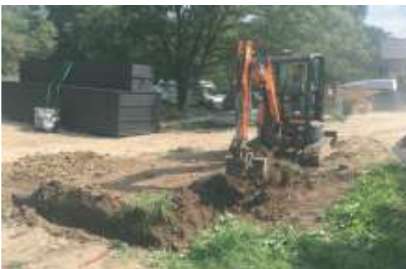
Plate 109. Canolfan yr Urdd, Pentre Ifan - Working shot during excavation of trench for Sewage Treatment Plant. Looking NE.
