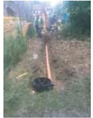
Plate 106. Canolfan yr Urdd, Pentre Ifan - Working shots during cutting of drainage trench at rear of Stables/Gatehouse. Looking E
