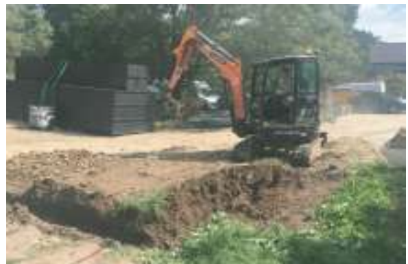
Plate 110. Canolfan yr Urdd, Pentre Ifan - Working shot during excavation of trench for Sewage Treatment Plant. Looking NE.
