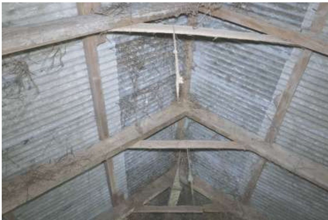
Plate 30. Canolfan yr Urdd, Pentre Ifan - Cart Shed. View of modern roofing timbers and corrugated asbestos roof. Looking W.
