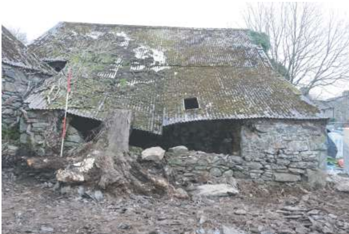
Plate 85. Canolfan yr Urdd, Pentre Ifan - Milking Parlour. View of west facing elevation of Parlour where tree rooting had compromised extension. Looking E.
