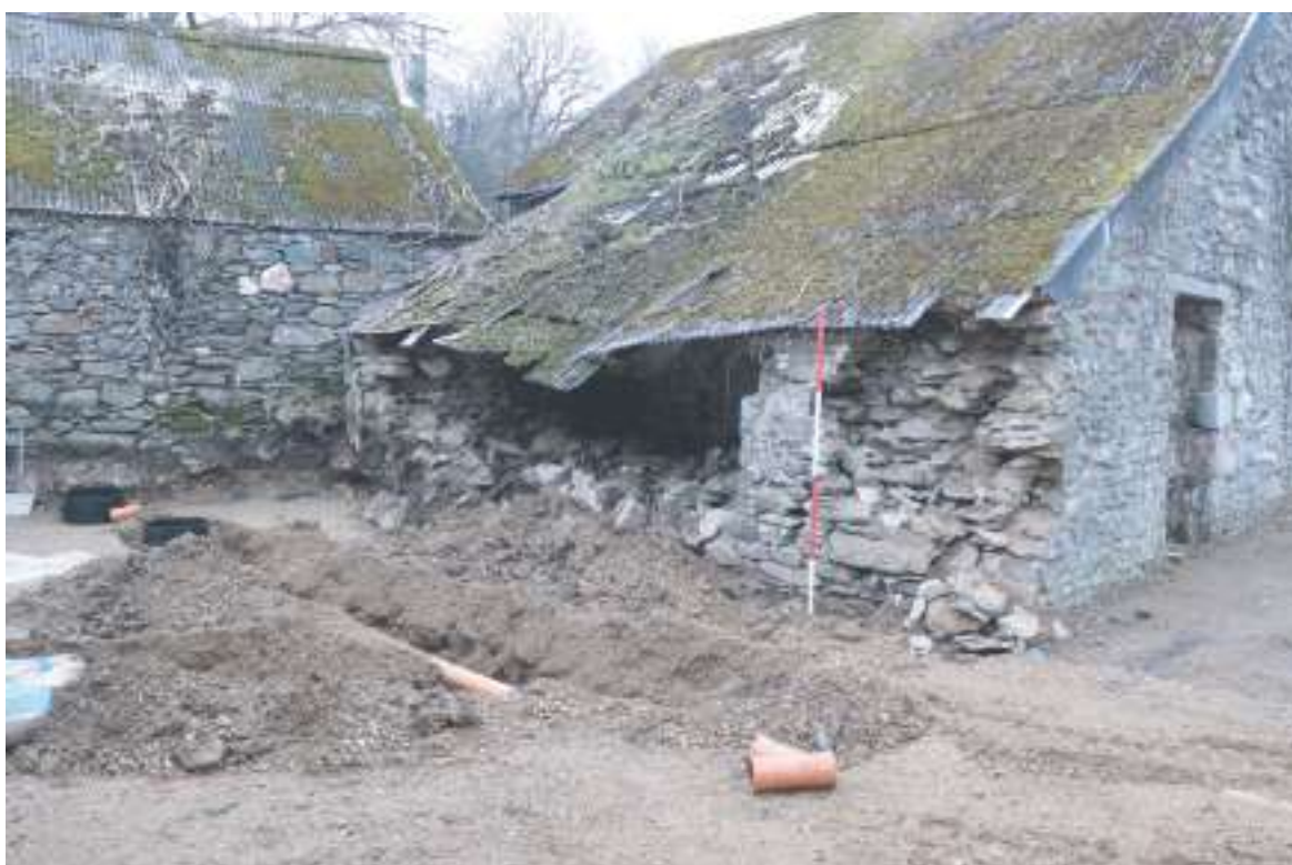
Plate 86. Canolfan yr Urdd, Pentre Ifan - Milking Parlour. View of west facing elevation of Parlour following removal of tree stump and excavation of drainage trench. Looking NE.
