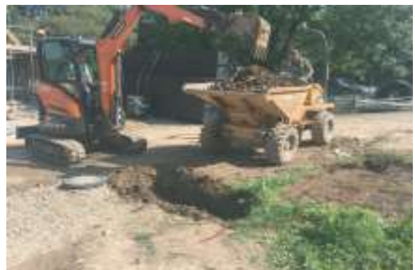
Plate 108. Canolfan yr Urdd, Pentre Ifan - Working shot during excavation of trench for Sewage Treatment Plant. Looking NE.
