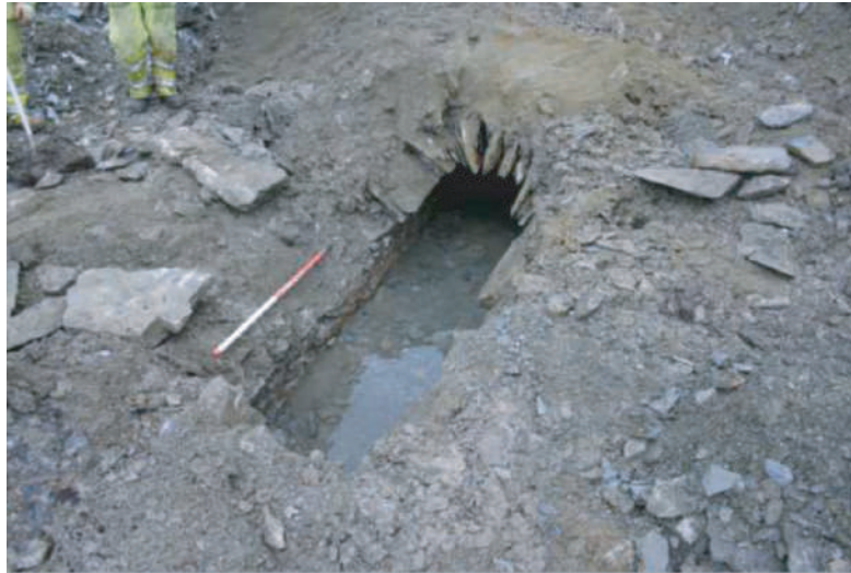
Photo 18: View of stone culvert (4000) following breach of arched roof.
