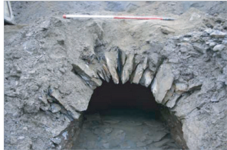
Photo 19: View southeast of arch in stone culvert (4000).
