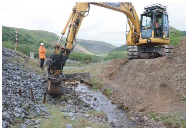
Plate 10. Working shot during removal of part of base of mine spoil tip alongside discharge point in preparation for Gabion baskets. Looking southwards.
