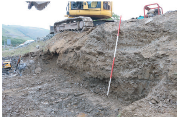
Plate 20. Groundwork complete on western bank for new Gabion baskets. Looking SW.
