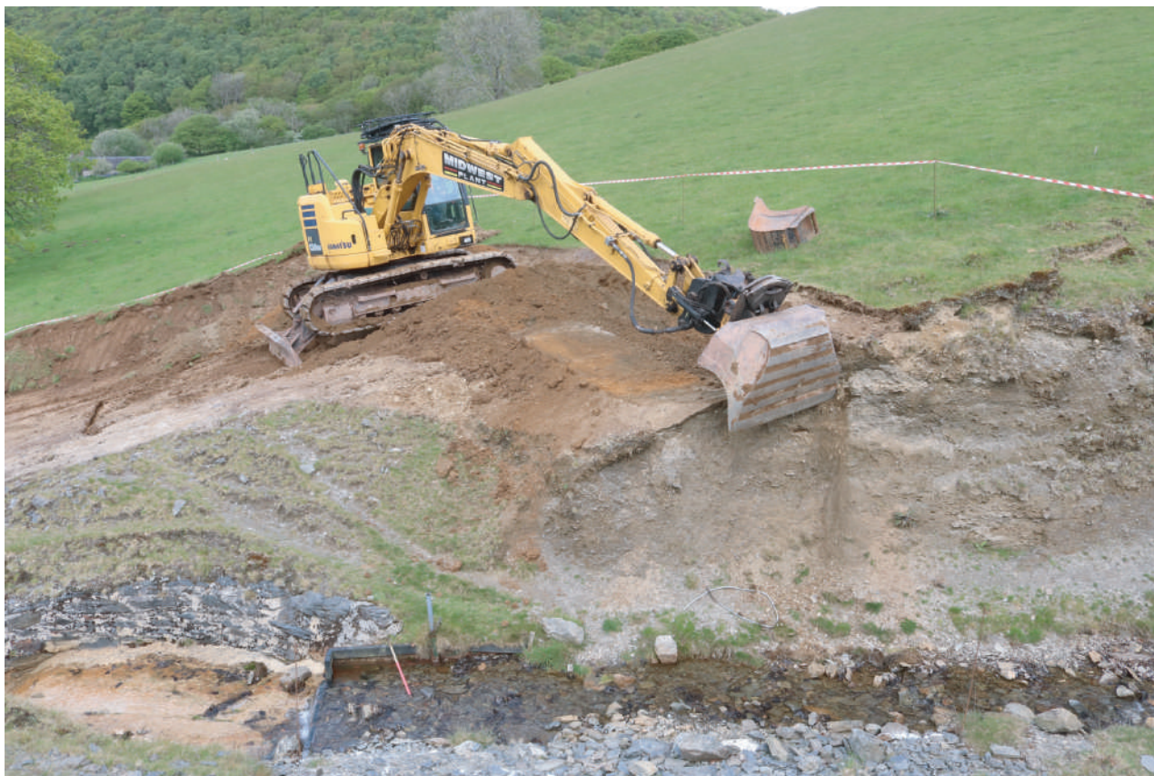
Plate 08. Working shot during turf and sub soil stripping in machine working area. Looking west.
