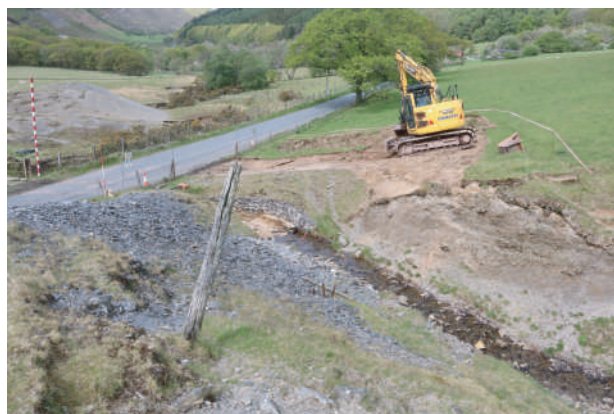
Plate 09. Working shot during turf and sub soil stripping in machine working area. Looking southwest.
