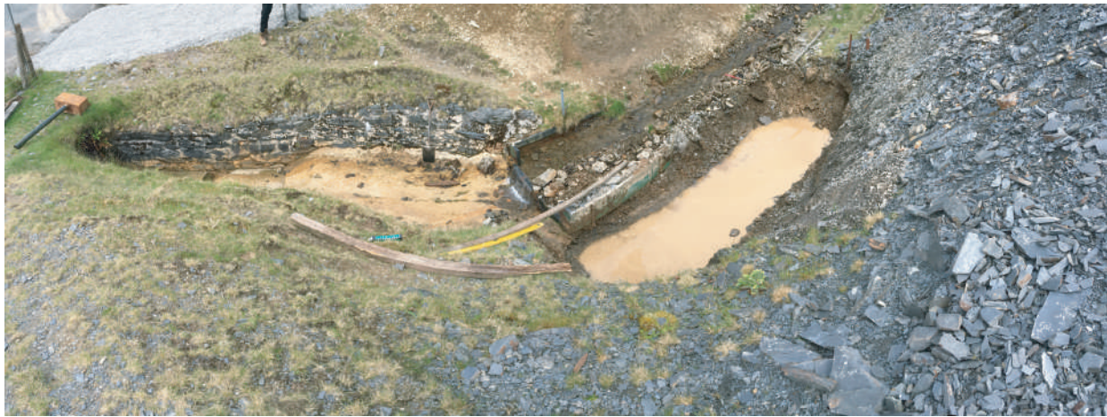
Plate 16. Spliced panoramic view looking west to north of partly dismantled existing flow gauge and area prepared for new Gabion baskets. in preparation for Gabion baskets at base of spoil tip.
