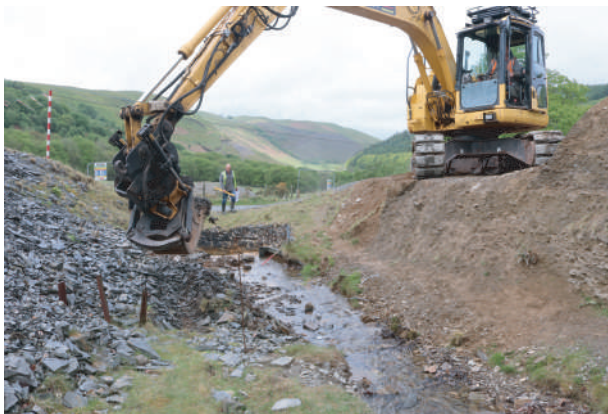
Plate 11. Working shot during removal of part of base of mine spoil tip alongside discharge point in preparation for Gabion baskets. Looking southwards.
