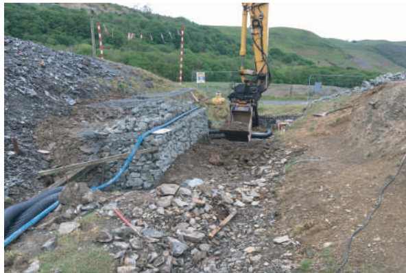
Plate 17. Working shot during clearance of stream bed and western bank in preparation for opposing Gabion baskets. Looking southwards.
