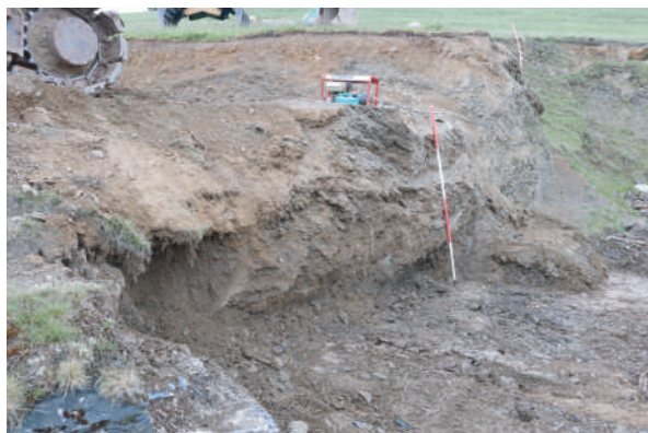
Plate 21. Groundwork complete on western bank for new Gabion baskets. Looking SW.
