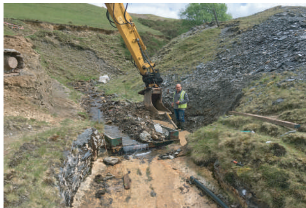
Plate 12. Working shot during removal of part of base of mine spoil tip alongside discharge point in preparation for Gabion baskets. Looking northwards.
