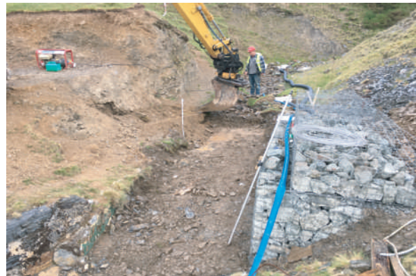
Plate 18. Working shot during clearance of stream bed and western bank in preparation for opposing Gabion baskets. Looking northwards.
