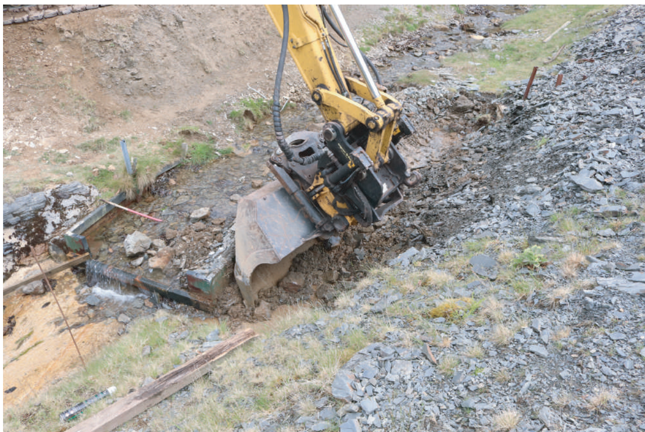
Plate 13. Working shot during removal of part of base of mine spoil tip alongside discharge point in preparation for Gabion baskets. Looking southwards.
