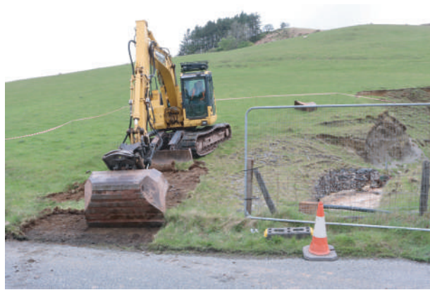
Plate 07. Working shot during turf and sub soil stripping in machine working area. Looking northwards.
