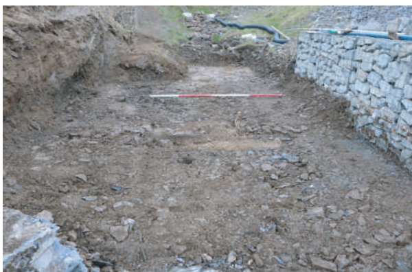
Plate 22. Groundwork complete in stream bed in preparation for concrete and new flume. Looking N.
