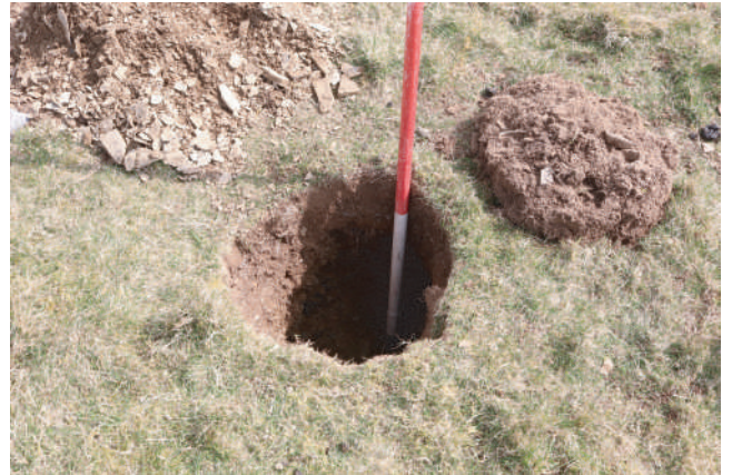
Plate 03. Trial Pit No. 2 (Hand dug).
