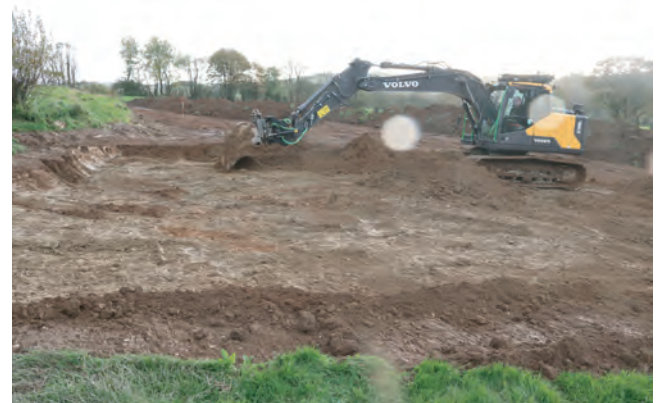
Plate 15. View of proposed Menage development area during turf and top soil strip. Looking southwards.
