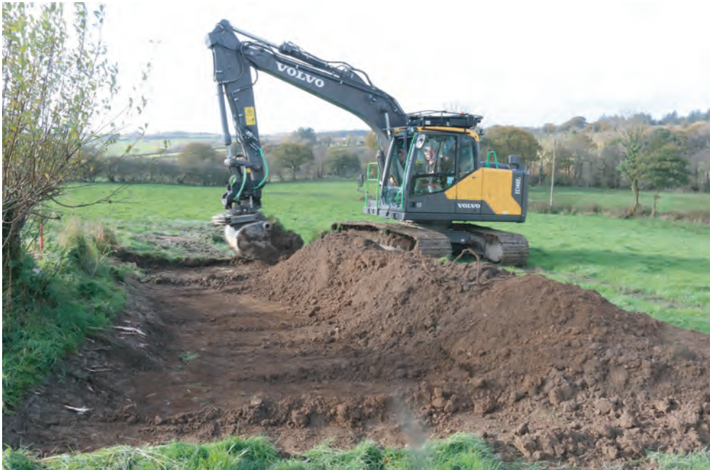
Plate 10. View of proposed Menage development area during turf and top soil strip. Looking southwest.
