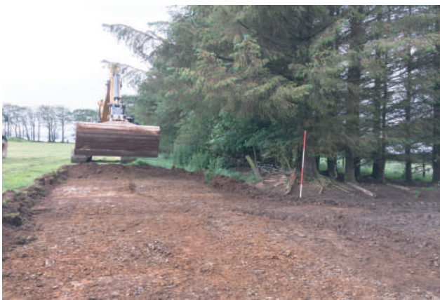
Plate 05. Working shot during access track creation. Looking west.
