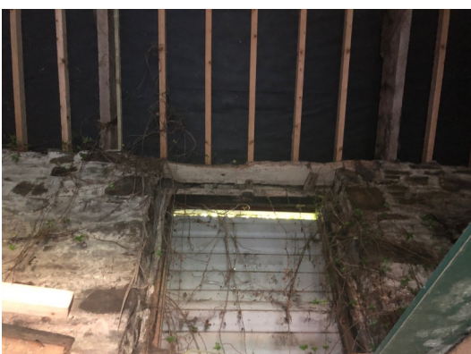
Internal view of roof space of cowshed showing new felt and battens
