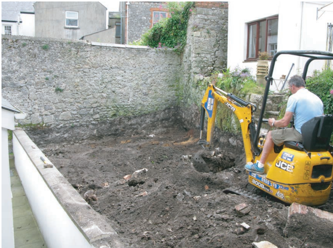
Plate 12. Working shot using mechanical excavator during ground reduction work in lower garden area, following removal of tree stumps. Looking east.
