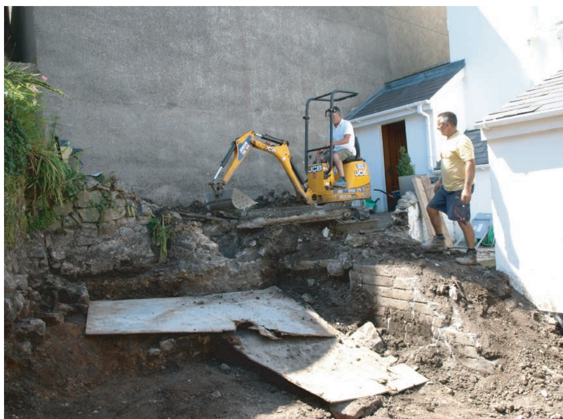
Plate 26. Working shot showing removal of concrete slab covering water well. Looking northwest.
