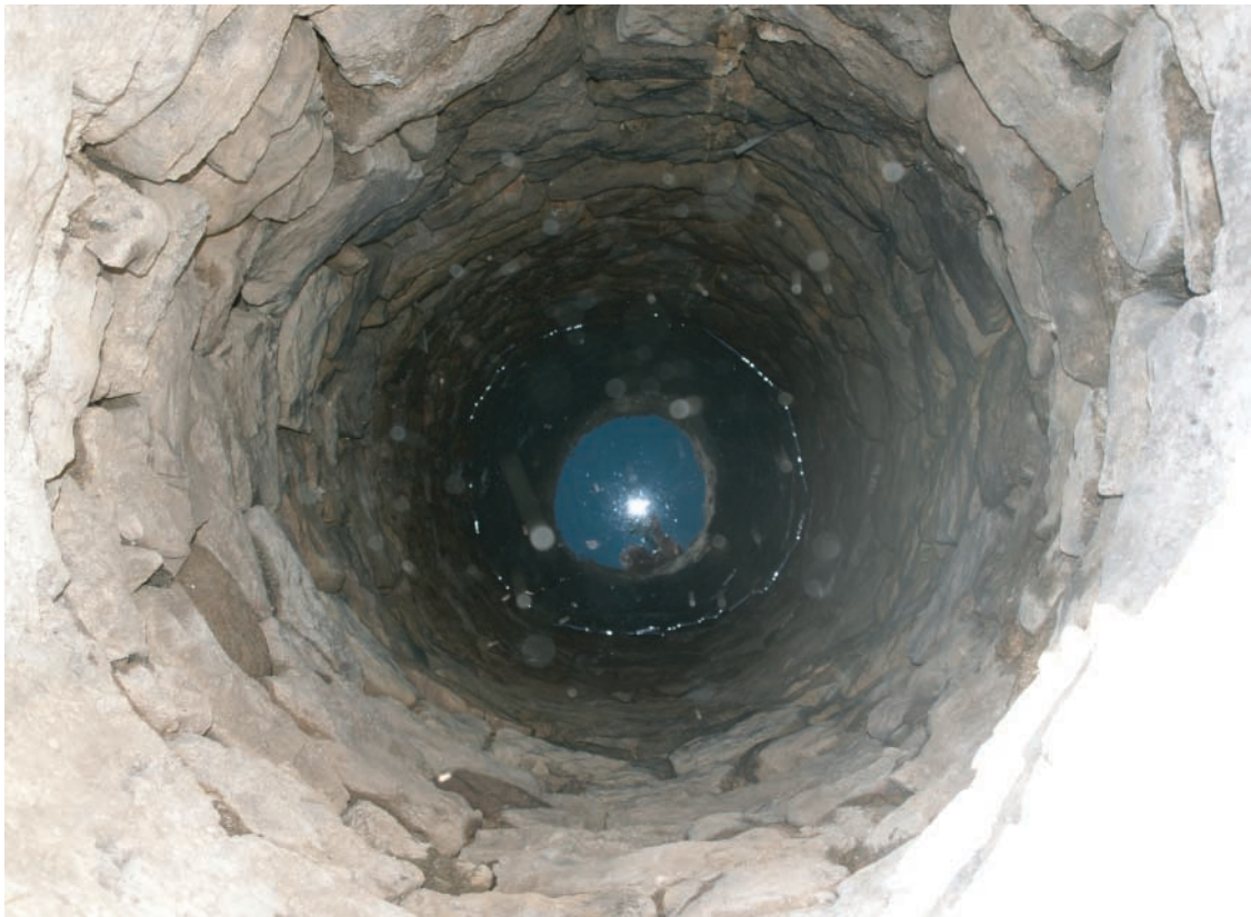
Plate 48. View down stone built well. Approximately 6.7 meters deep.
