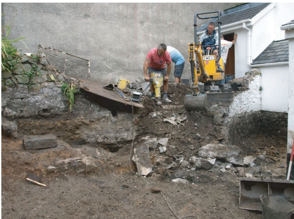
Plate 27. Working shot showing removal of concrete slab on northern side of water well. Looking northwest.
