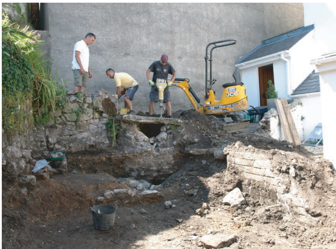
Plate 25. Working shot showing removal of concrete slab covering water well. Looking northwest.
