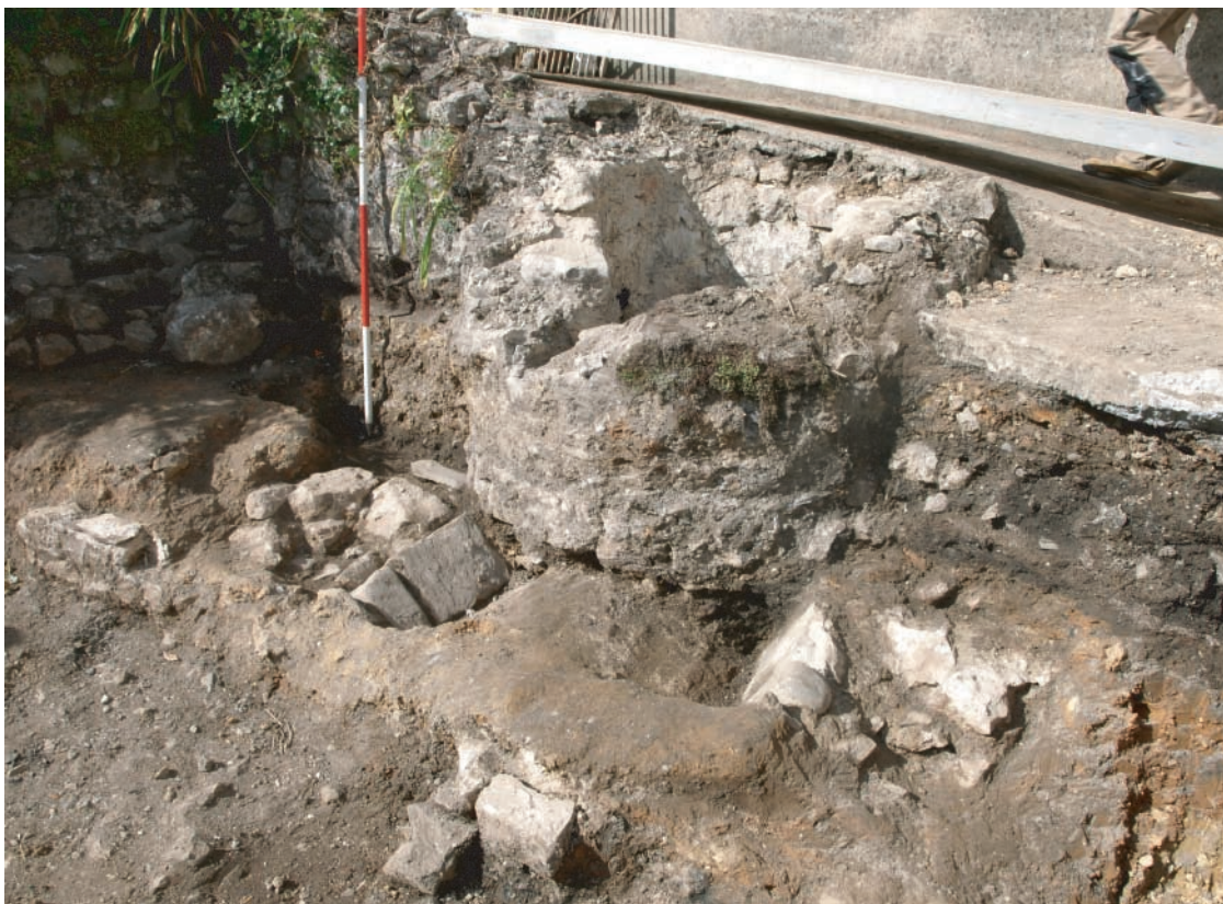
Plate 40. View of remains of stone built water well following ground reduction. Note cut slots at base of well through natural sandstone, which likely acted as locking slots to support a timber 'A' frame. Looking southwest.
