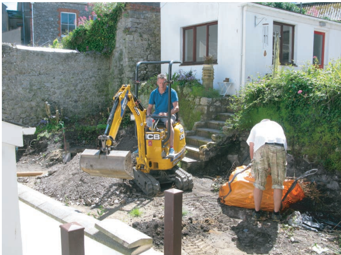
Plate 10. Working shot using mechanical excavator during ground-work for ground reduction, in lower garden area. Looking east.
