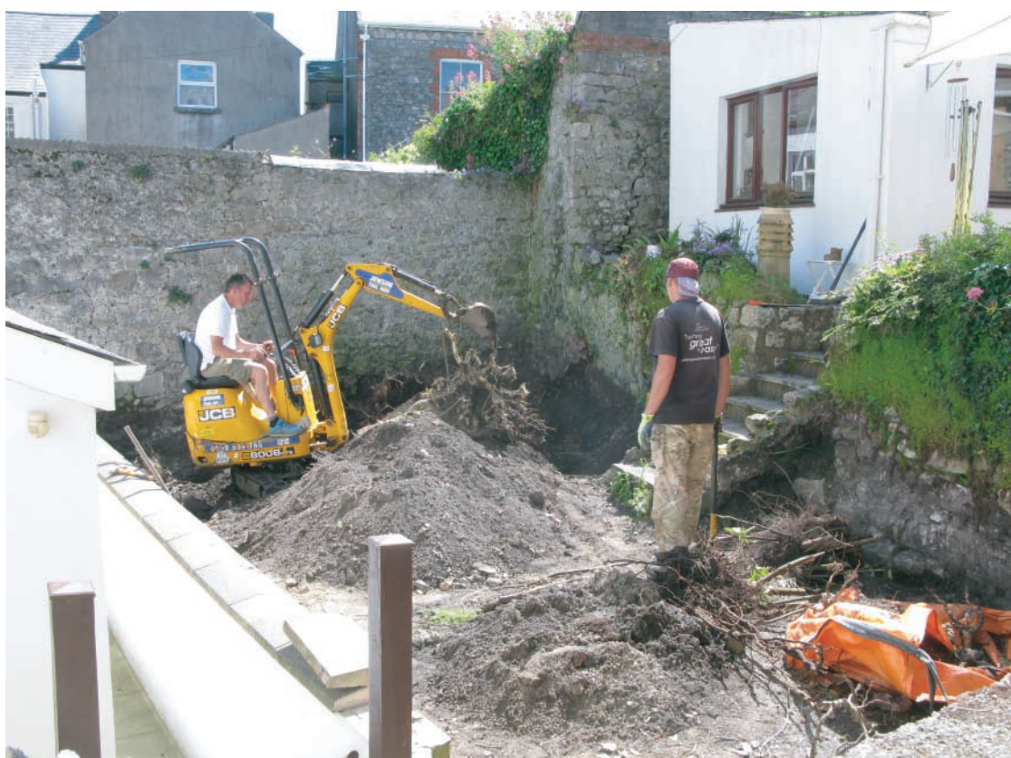
Plate 11. Working shot showing mechanical excavator removing tree stump during groundwork for ground reduction in lower garden area. Looking east.
