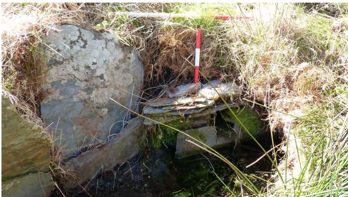
Photo 11: Glasffrwd Well PRN 36494/SAM CD183. Edge of the cistern, showing the wooden inlet pipe. 1m & 0.3m scale.
