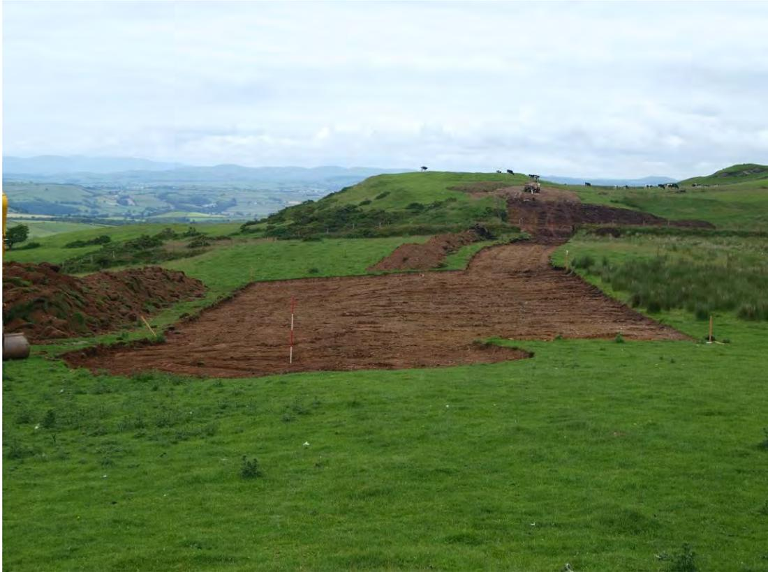
Photo 13: North facing shot of the stripped area, including the turbine base and crane pad. 2m scale.
