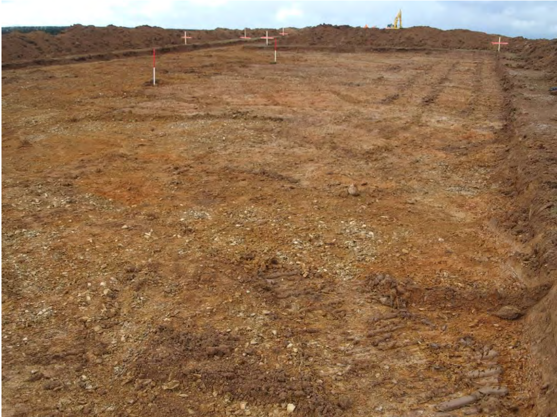
Photo 7: Area stripped for the crane pad foundations, facing N. 1m scales.
