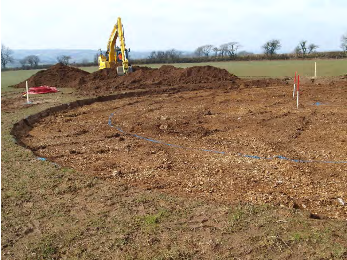
Photo 9: Area stripped for the Turbine foundations, facing NW. 1m scales.
