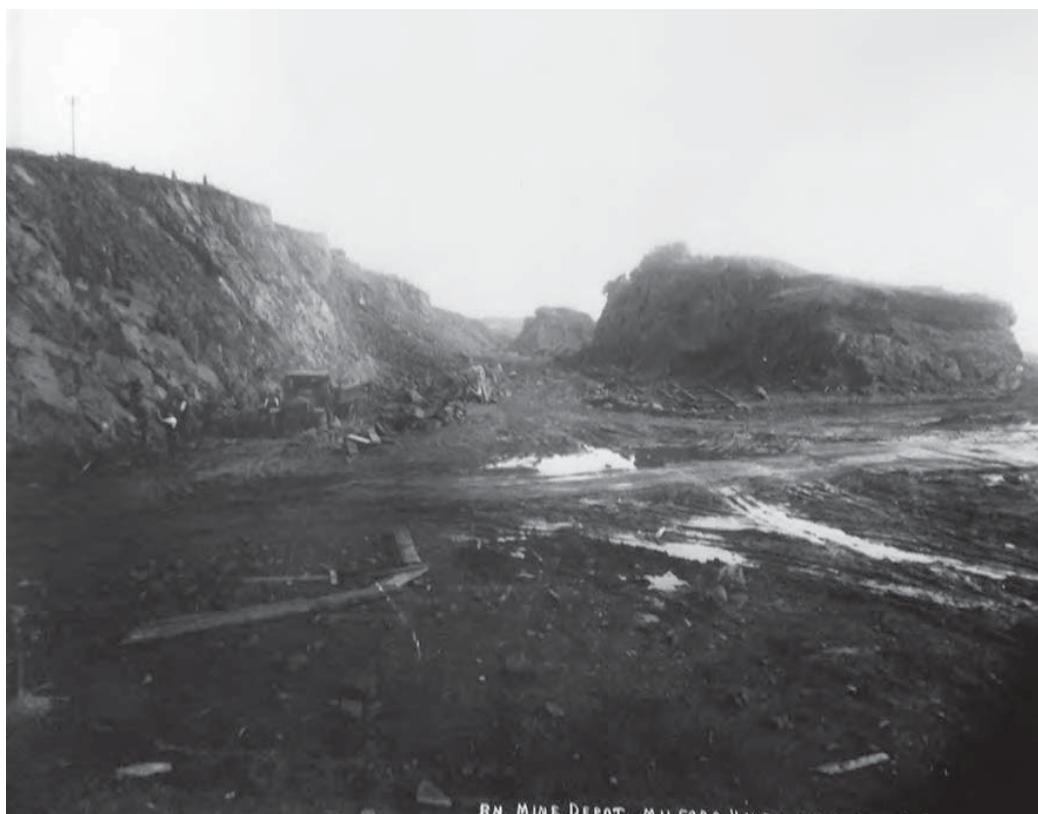
Photo 7: Photo taken in the mid-1930s during construction work on the RNAD site. Showing cutting of railway PRN 34525. The rock face to the left was quarried vertical, the outcrop to the right was removed and the Bulk Store built at that location. Image courtesy of Scolton Manor Museum.
