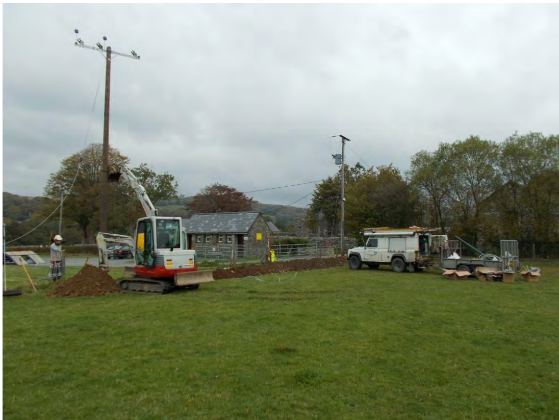
Photo 20: Northeast facing shot of the new electricity pole installation and cable trench excavation, both of which were archaeologically evaluated.
