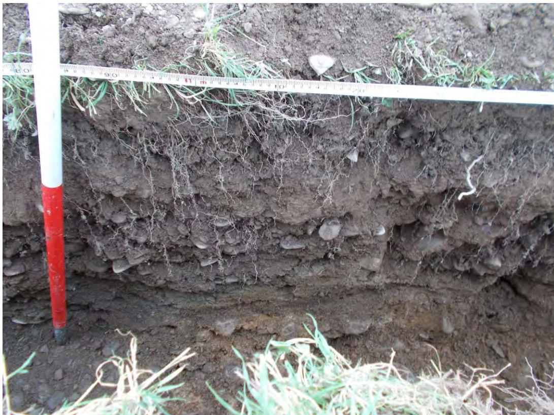
Photo 22: South facing shot of the cable trench, taken at an acute angle due to the narrow width of the trench. Shows topsoil overlying natural fluvial deposits. 1m scale.
