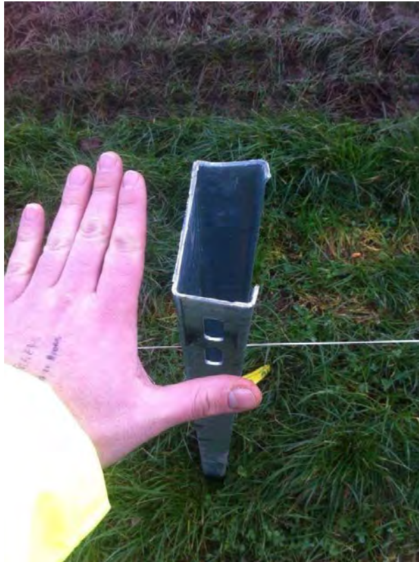
Photo 29: A preformed C section pile, of the type used in the areas adjacent to the area of archaeological significance.
