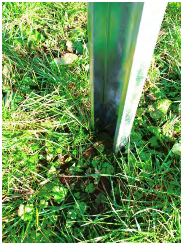
Photo 30: A preformed C section pile, of the type used in the areas adjacent to the area of archaeological significance.
