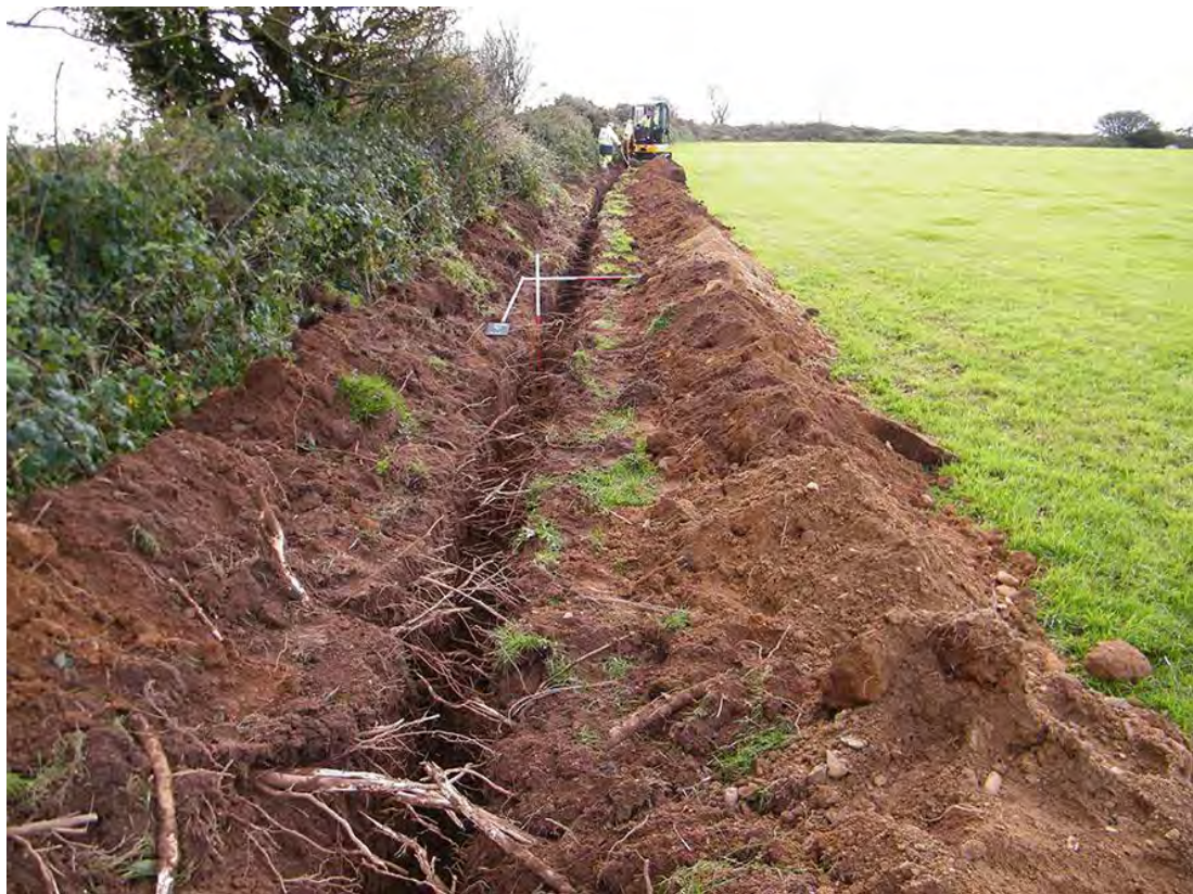
Photo 4: Working shot of the excavation of the cable trench (Trench 1) in the field to the south of the village.
