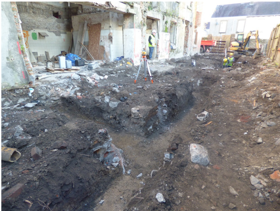
Plate 5: Detail of the excavated foundation trenches in Monitoring Area 2
