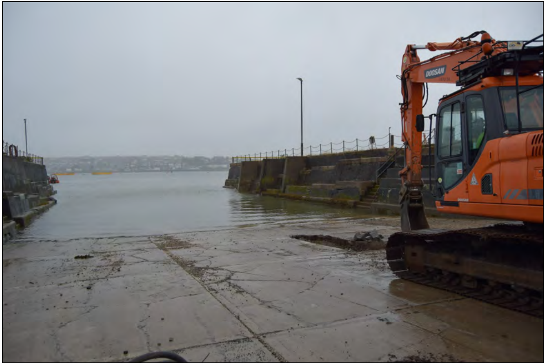
Plate 3: Slipway 1, view to the NNE.
