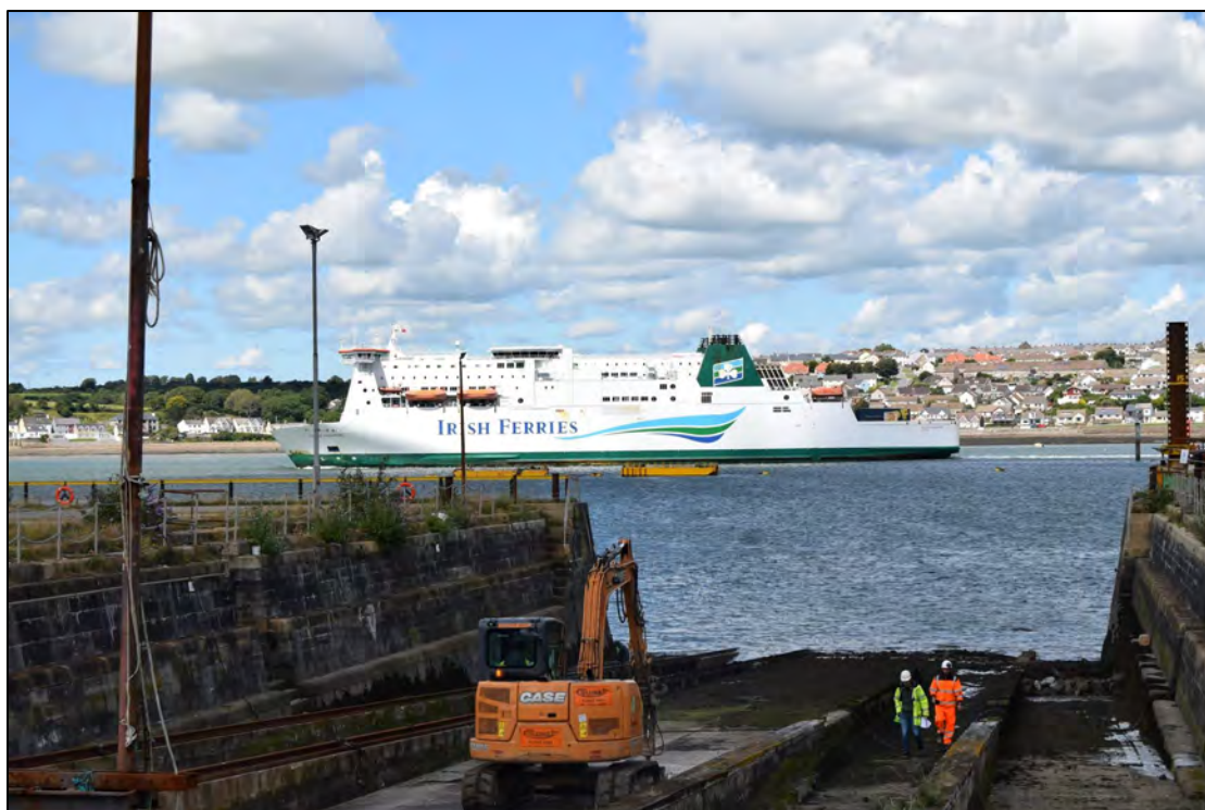
Plate 1: Historic Building Slip Number 1, view to NNW.
