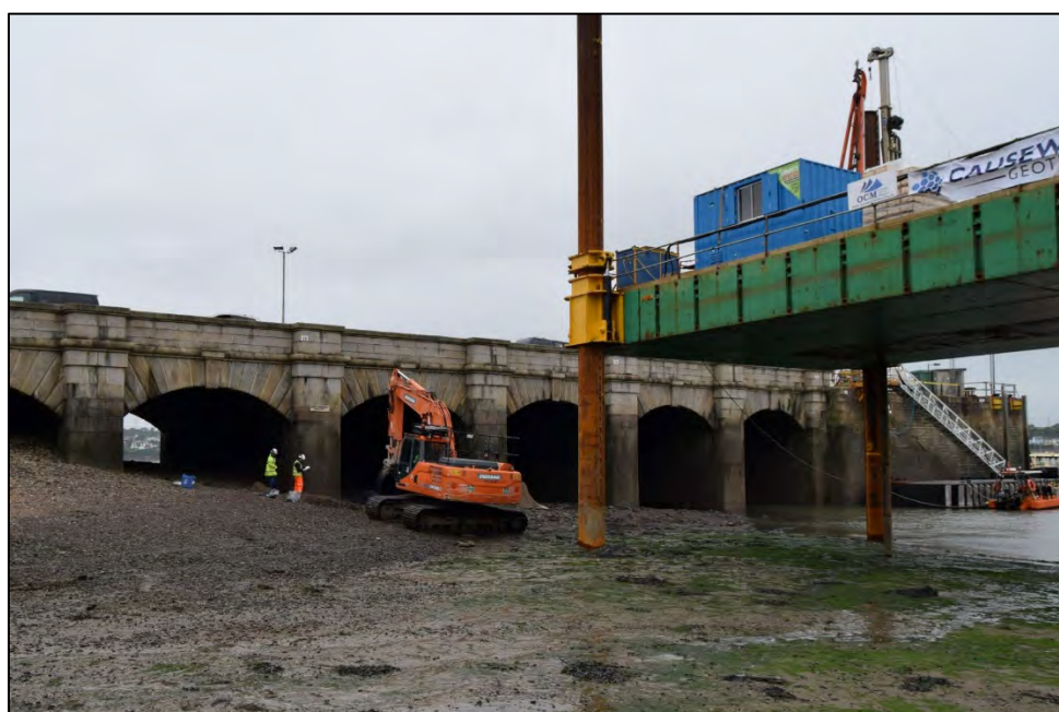
Plate 40: STP403 working shot, view to the west.
