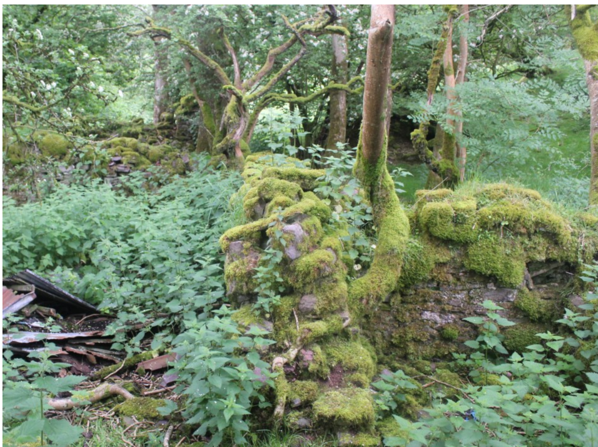
Figure 19. Trees growing within the masonry.
