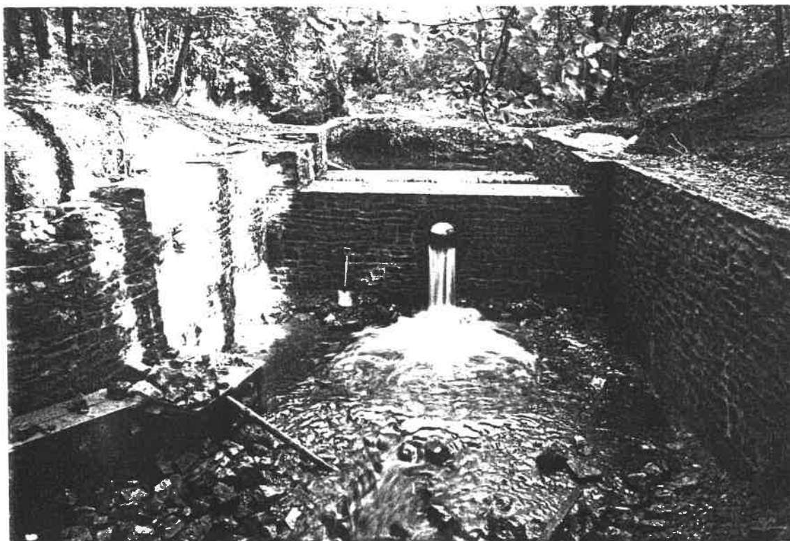
The Fish Pond Cascade: photographs taken during and after rebuilding. The upper photographs clearly shows damage caused by floodwaters at this site. The double-weir arrangement of this feature is visible in the lower photograph.
