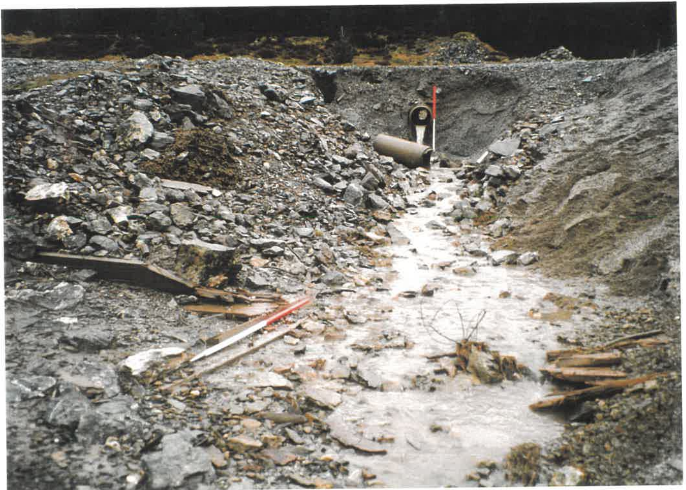
Plate 3: Dressing floor area at Location 4, prior to works. View from south shows part of a damaged wooden collection box for slimes. 1m ranging pole in the background shows the concrete pipe to be replaced.
