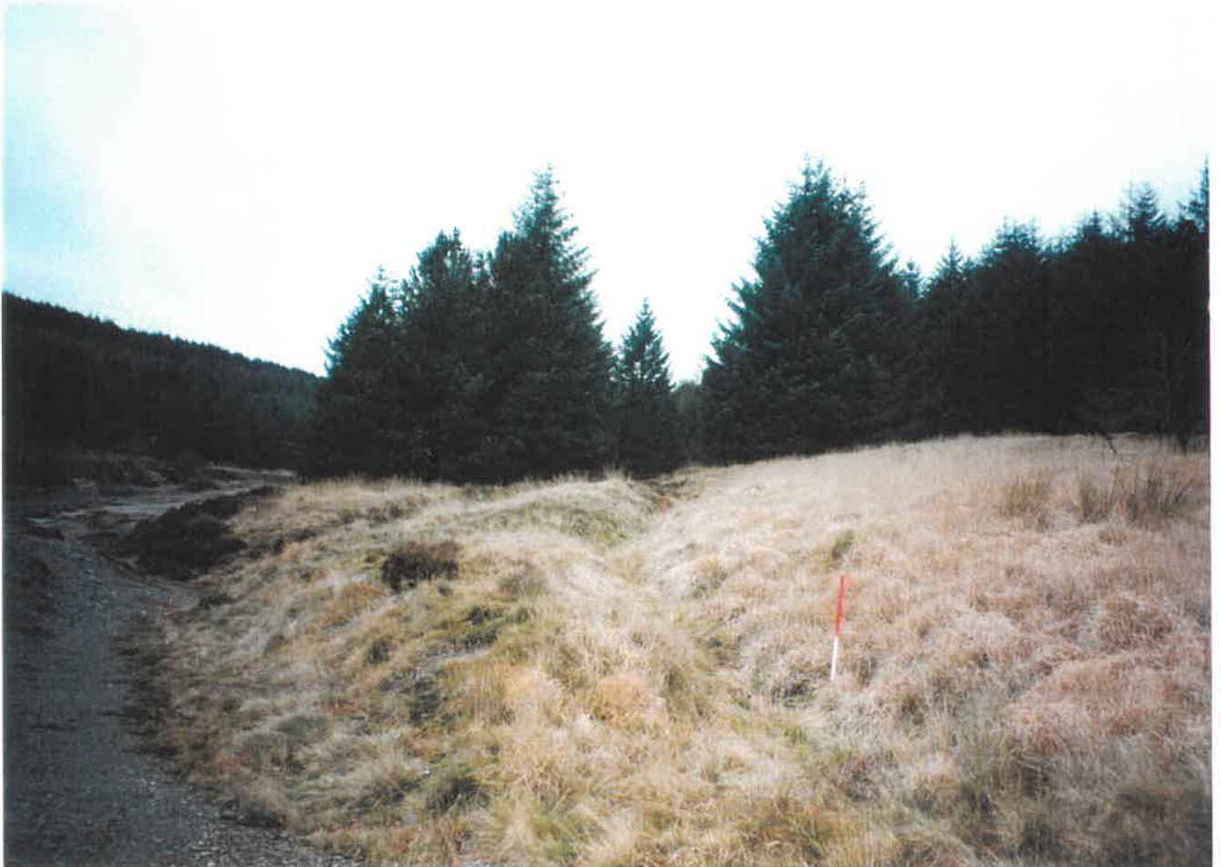
Plate 6: View from east from Location 3, prior to works. 1m ranging poles show the embanked leat/watercourse of upland stream, which has dried up since the flow of water was cut off presumably during forestry work in the 1950s. The dry bed will be utilised as the run-off as outlined in Fig. 1. To the left of the photograph, south of the rough grass, is the line of leat PRN 28195, with its embankment covered in fine waste.
