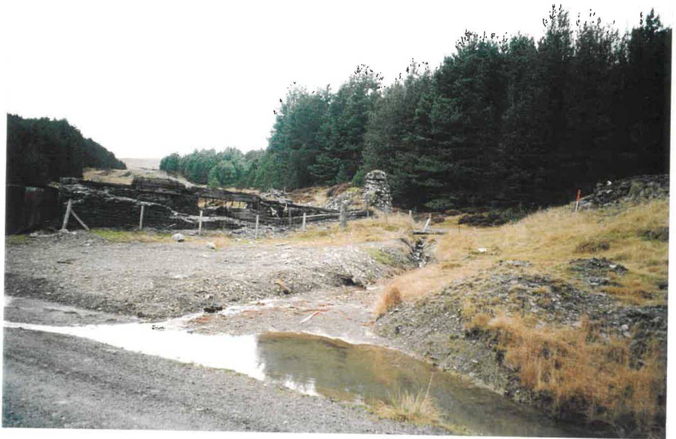
Plate 1: Crusher house wheelpit ( PRN 38065 ), prior to works. View from SE shows the flow of water running down-hill from the forestry RUPP. The water has followed the N side of the tramway which is visible on the right side of the photograph.
