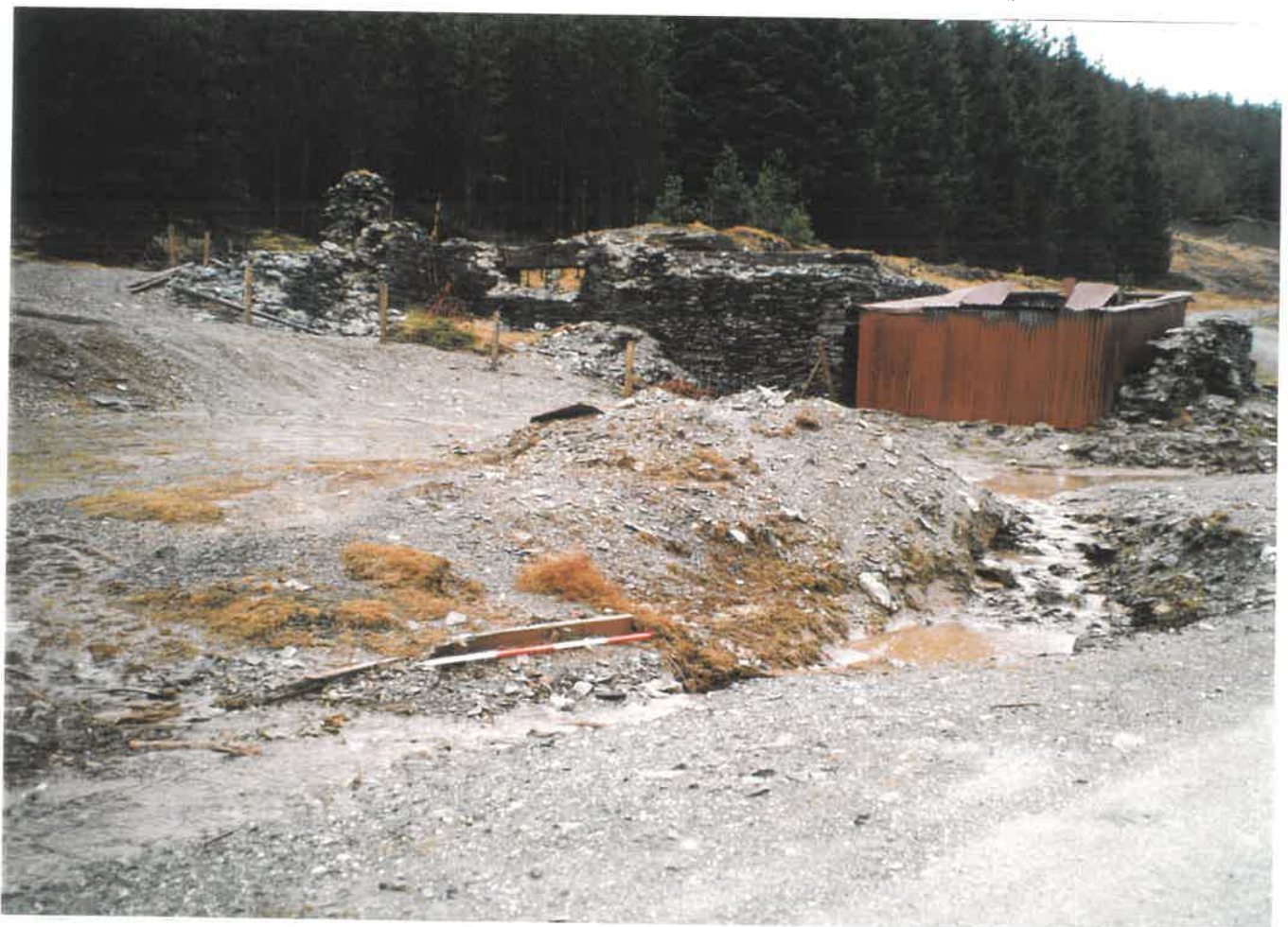
Plate 2: View from east, showing the natural collection point for run-off water, prior to works. 1m ranging pole identifies part of a damaged wooden launder box, N side of the forestry road.
