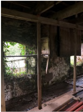
PHOTO 23: Internal image of the timber boxing between windows 02 and 03.
