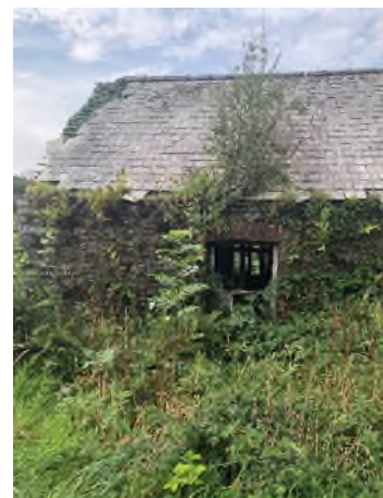
PHOTO 27: External image of window 08 and roof damage at eaves.
