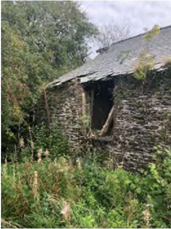
PHOTO 34: External image of window 05, roof damage at eaves and immediate surroundings.
