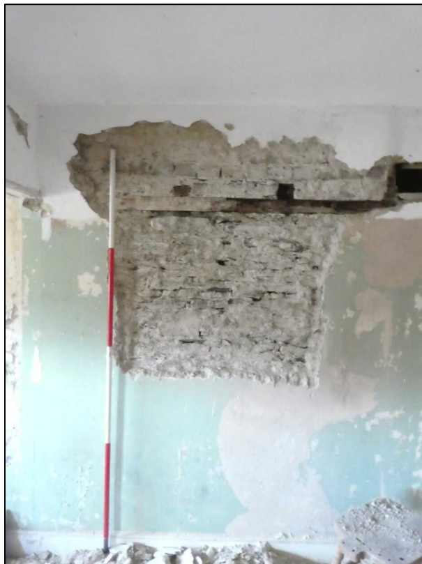
Plate 112: Timber in eastern wall of Bathroom 1
