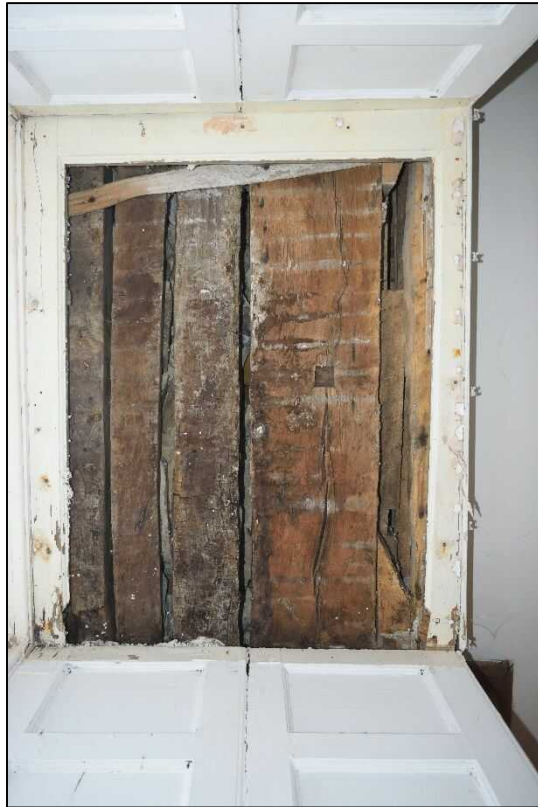
Plate 91: Timber work above window (GW10) in the Office
