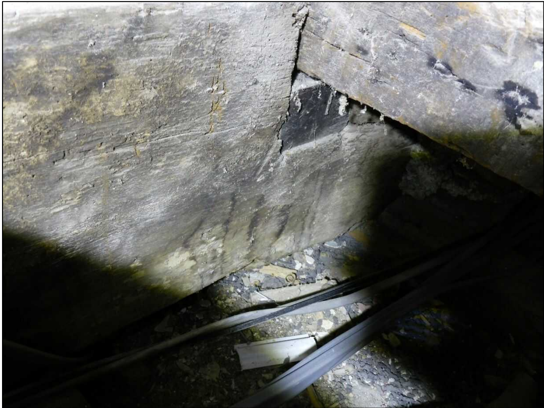
Plate 101: Packing below the joists of the beam between Bedrooms 2 and 3
