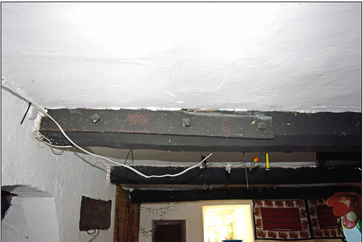
Plate 20: Iron support for the ceiling beam over the fireplace
