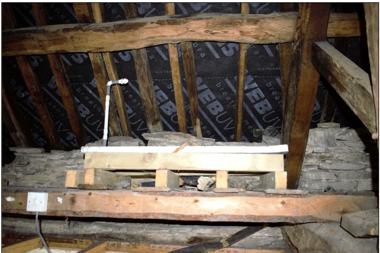
Plate 84: Platform for the water tank above Bathroom 2
