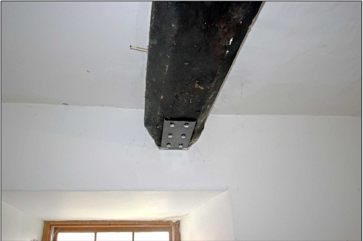
Plate 21: Metal support at southern end of ceiling beam 4
