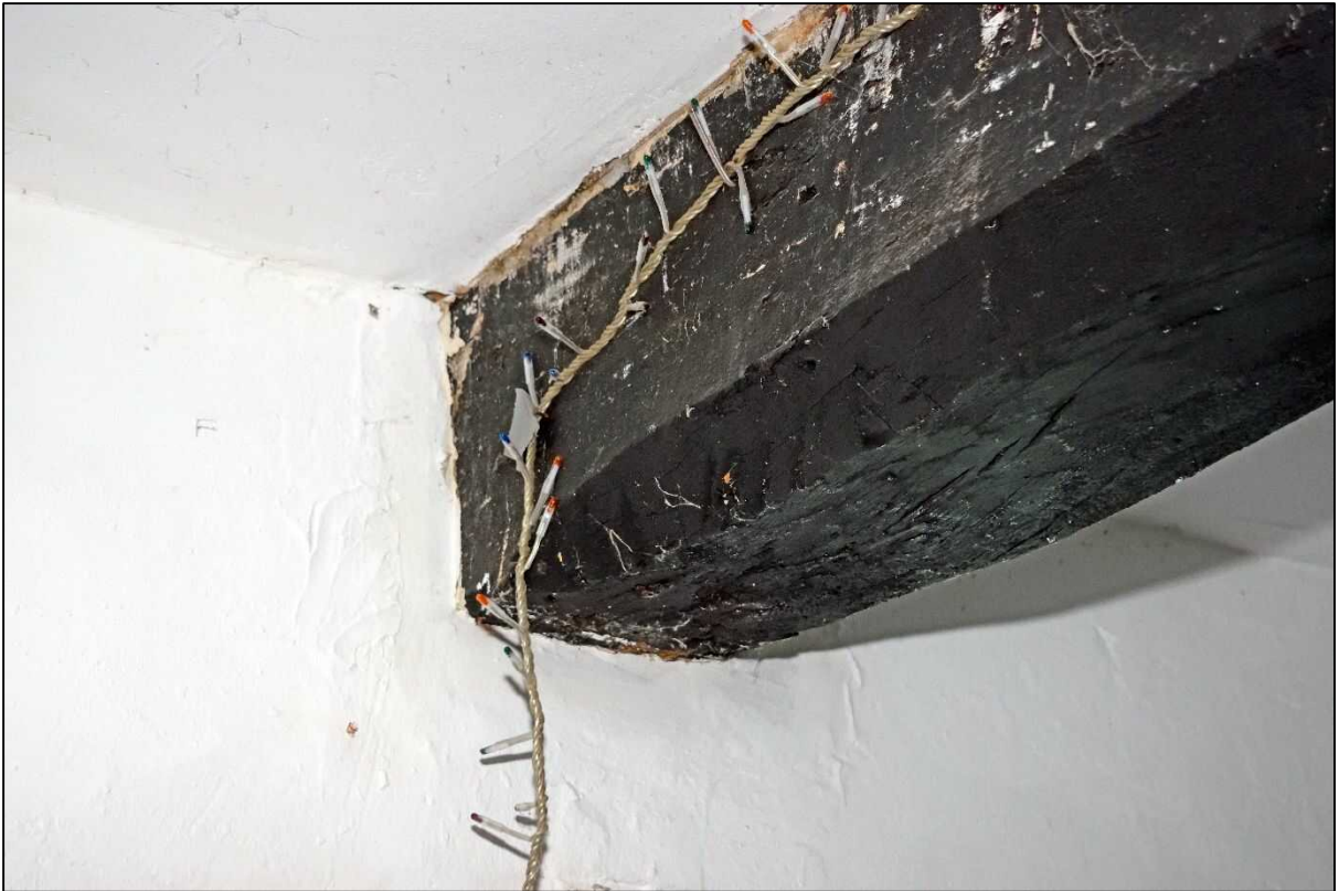
Plate 19: Runout stop on the ceiling beam 1
