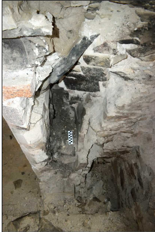
Plate 95: Blocked fireplace in northern wall of the Utility Room
