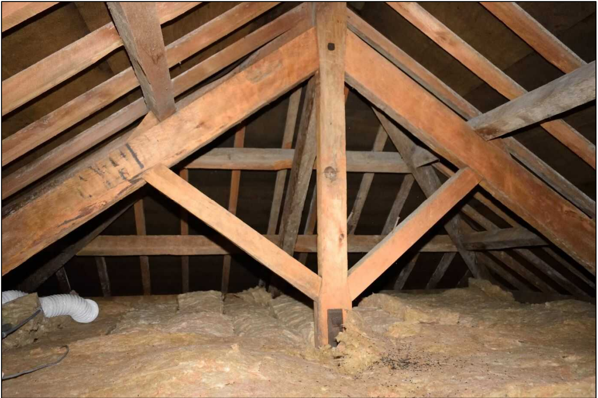
Plate 85: Truss in nineteenth century extension
