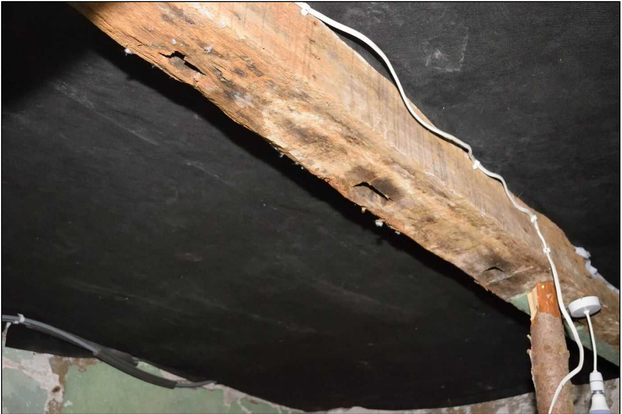
Plate 25: Mortice holes below the ceiling beam in Cellar 2
