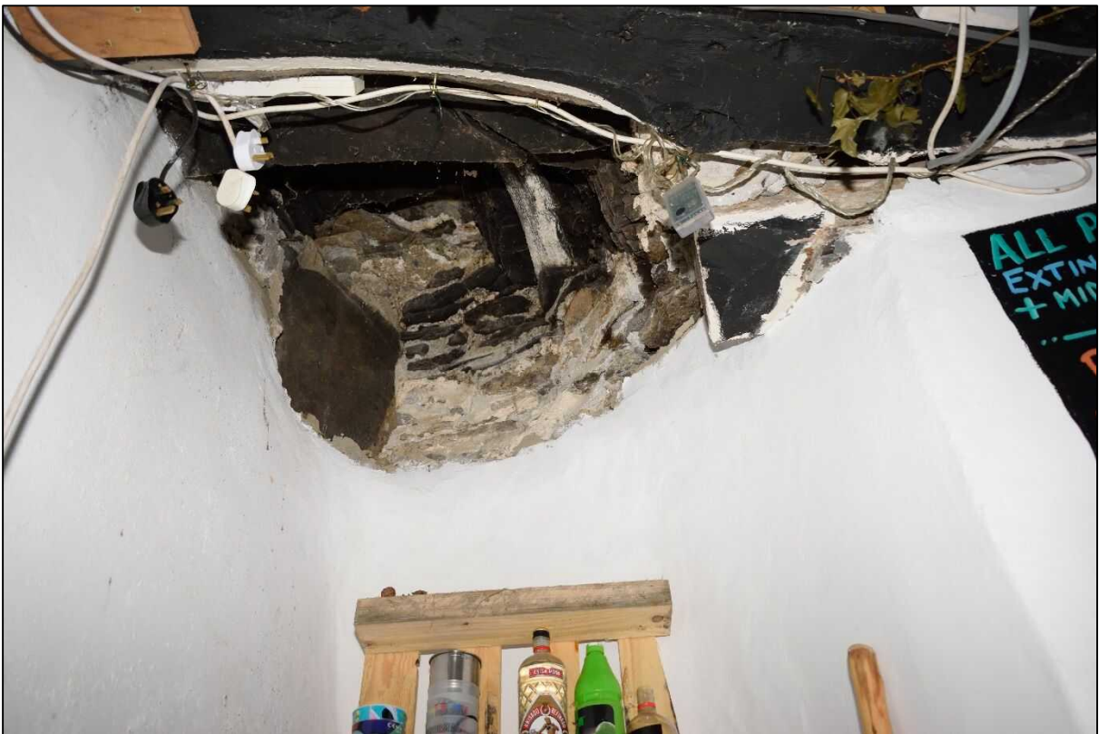
Plate 14: Probable chimney shaft in north-west corner of Cellar 1
