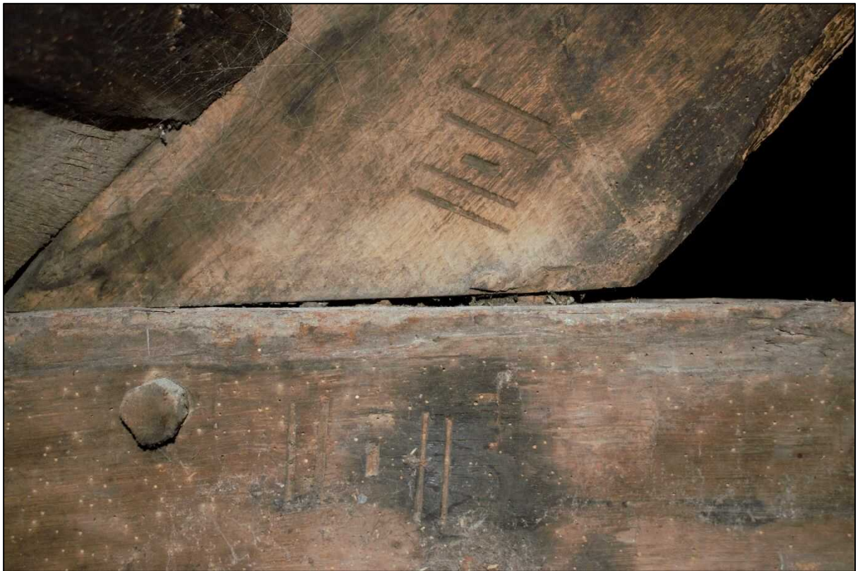
Plate 83: Carpenters marks on a truss above Bathroom 2
