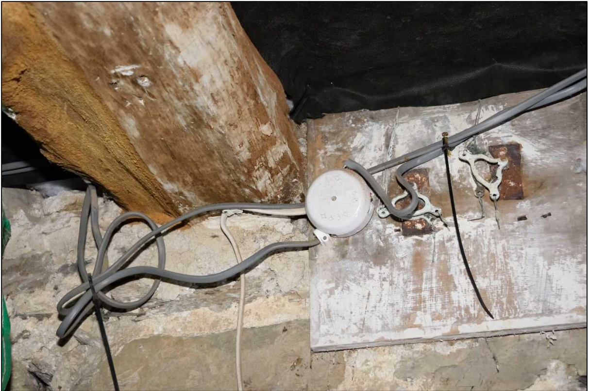
Plate 31: Pivots for a bell system in Cellar 3
