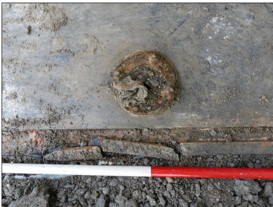
Plate 141: Detail of drain in the base of the slate tank
