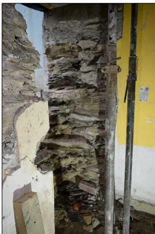
Plate 94: Section through the north wall of the Utility Room
