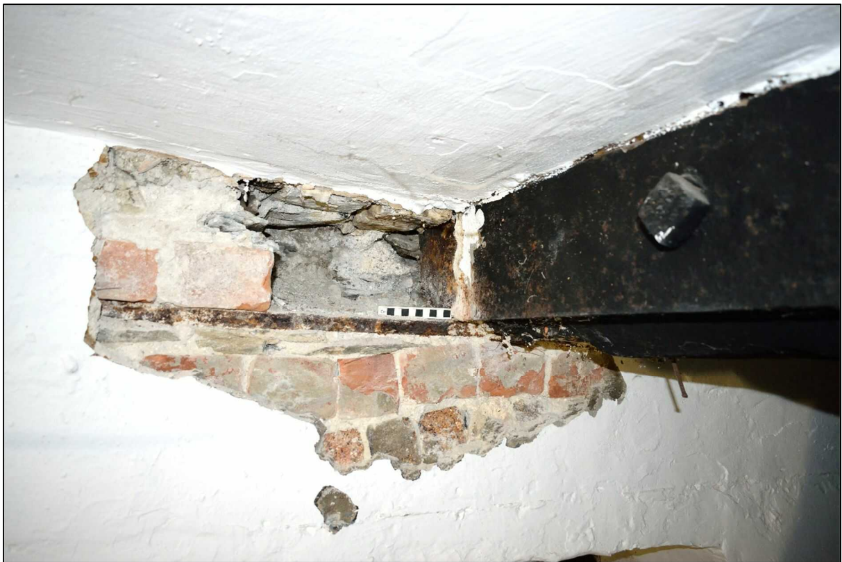
Plate 88: Metal plate supporting Beam 2 in Cellar 1
