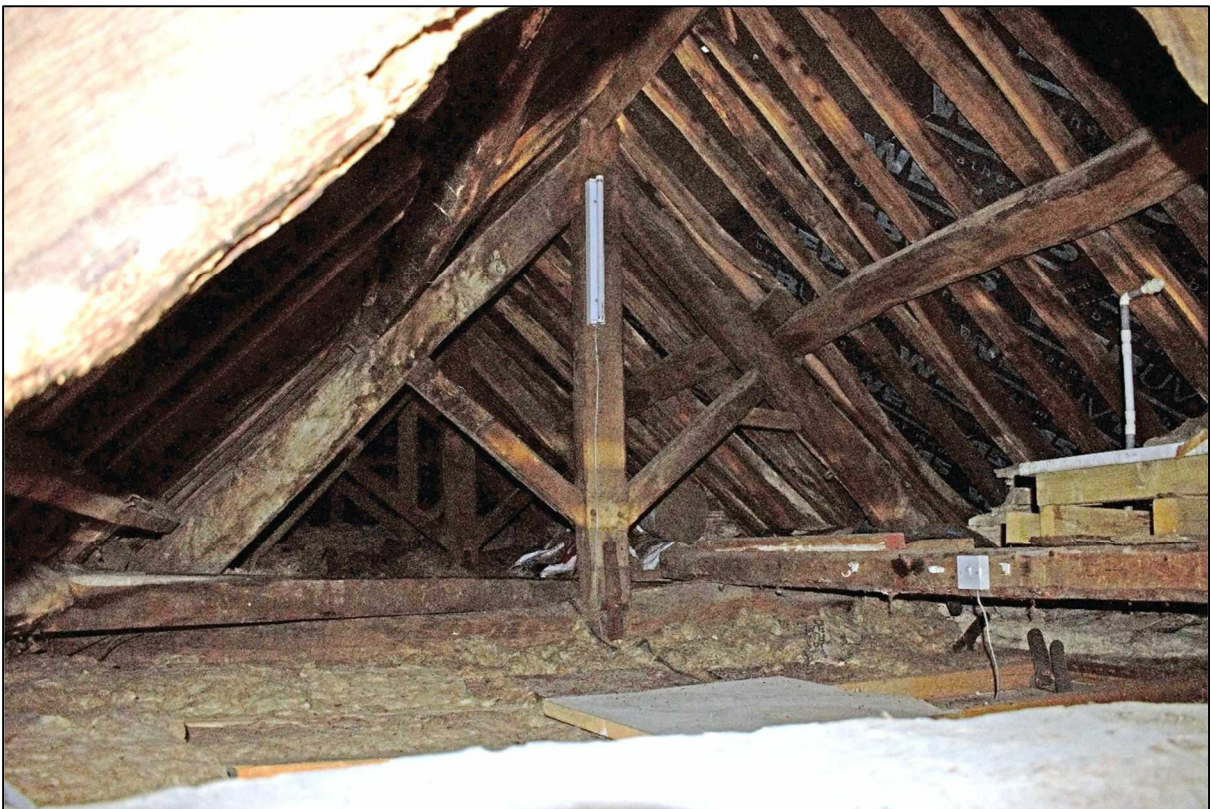
Plate 82: Truss in northern roof
