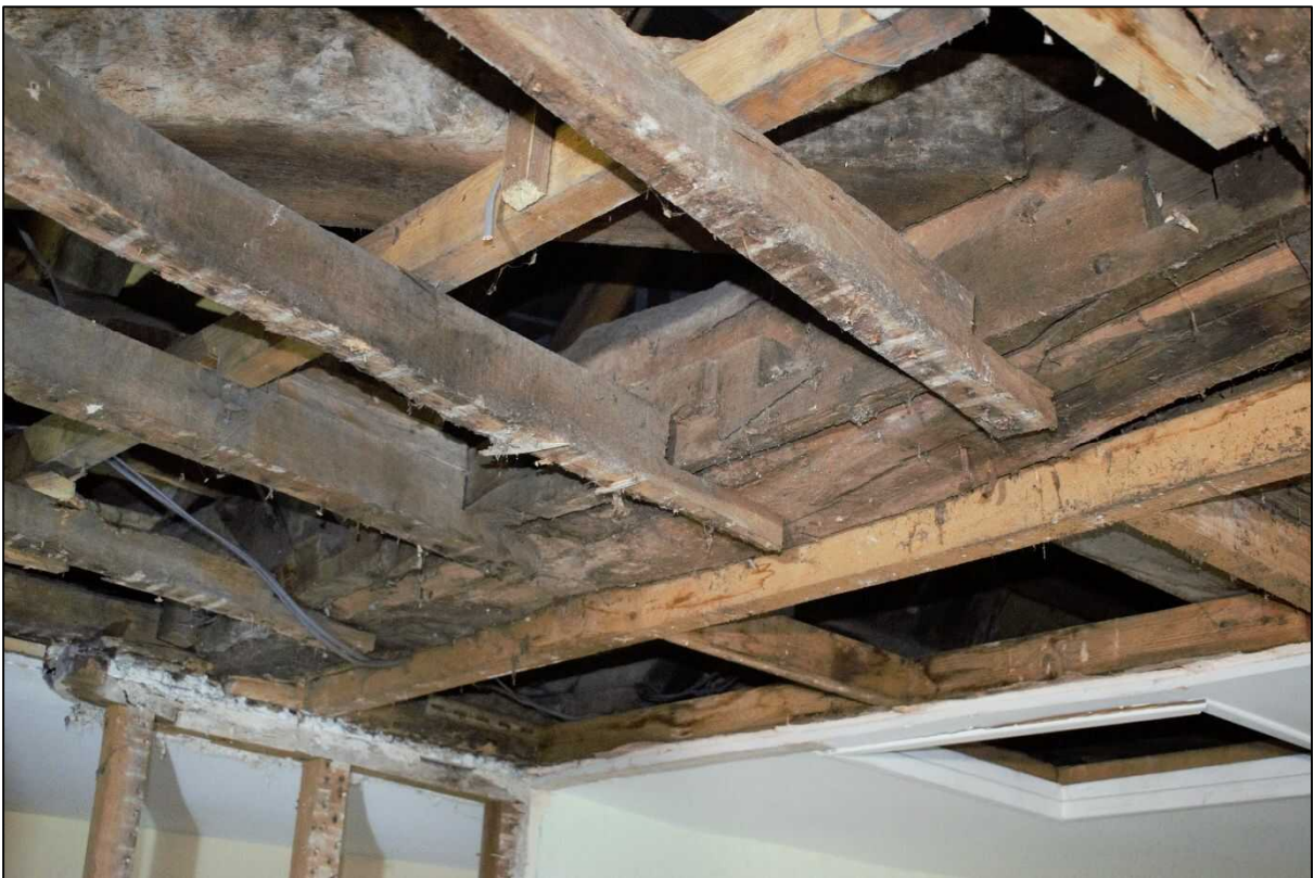
Plate 118: Plate nailed on to side of tie beam above Bathroom 2
