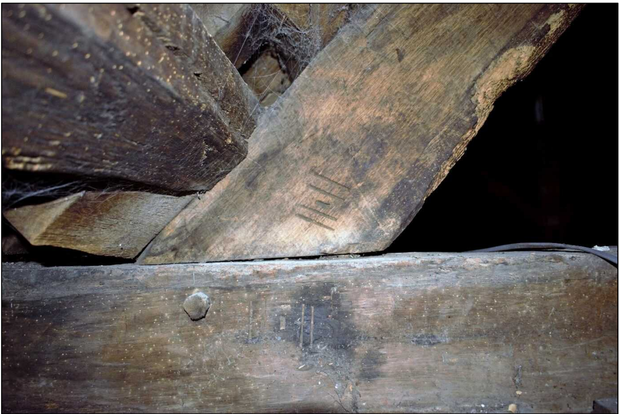
Plate 120: Carpenter's marks on truss above Bathroom 2
