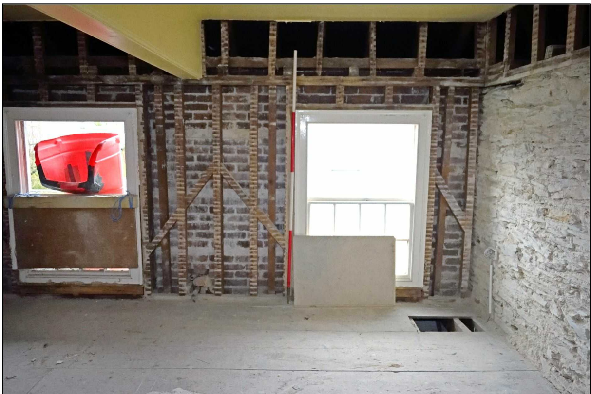
Plate 114: North wall of Bathroom 1 after the removal of the plaster
