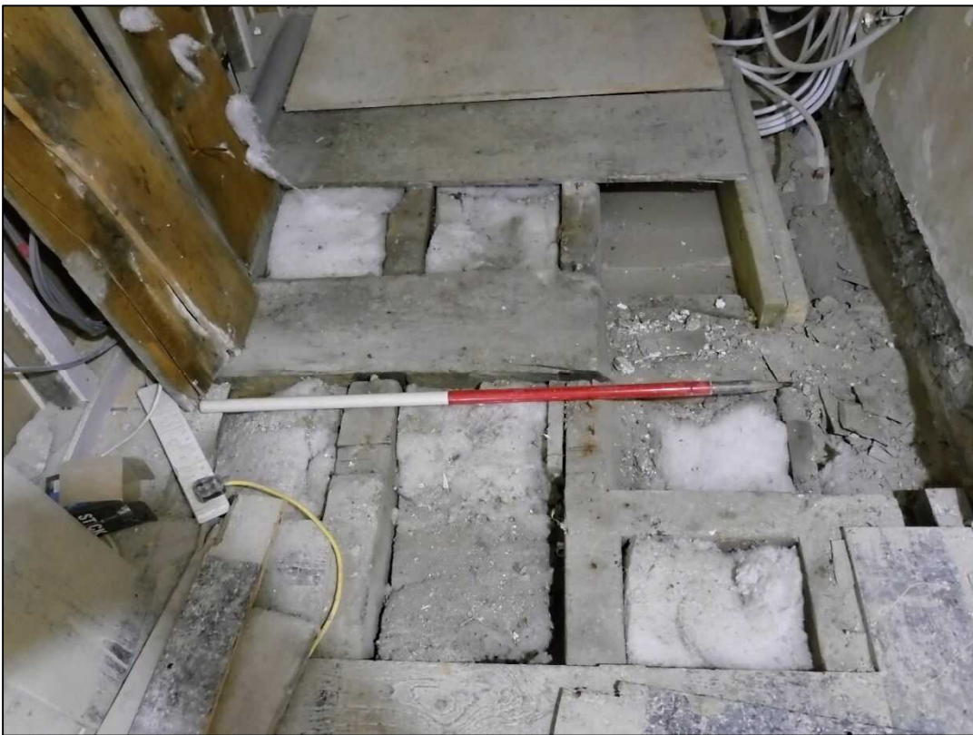
Plate 98: Beam below the ground floor corridor adjacent to the Utility Room
