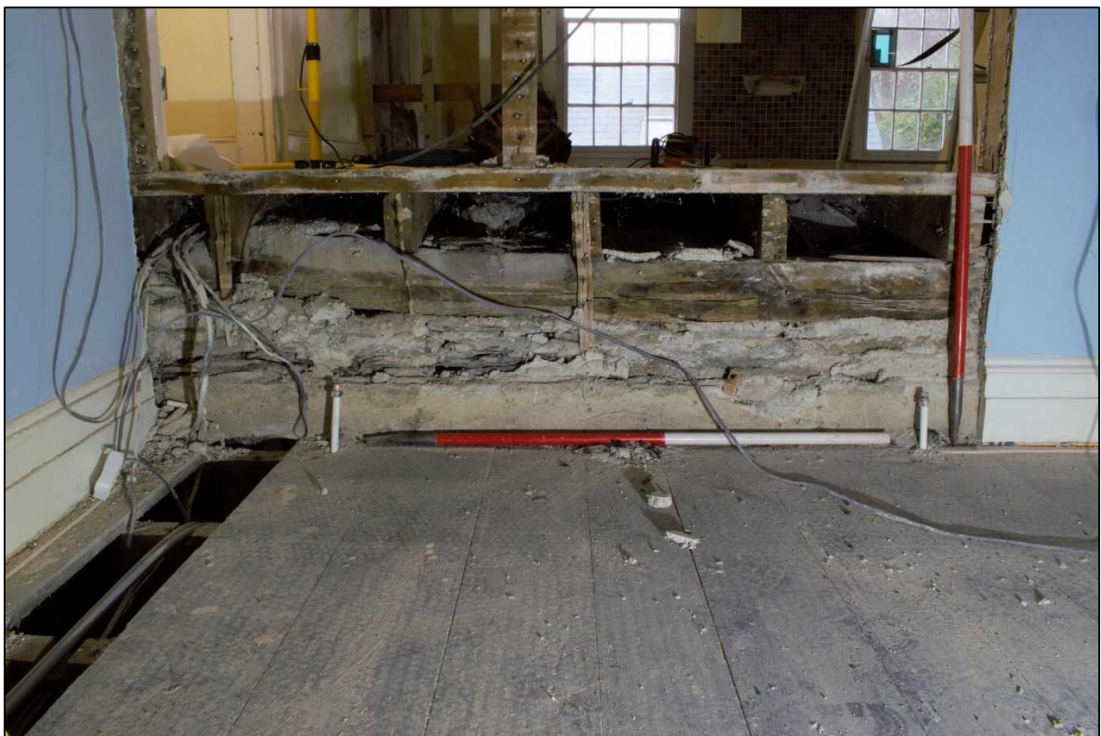
Plate 108: Structure below the partition between Bathroom 1 and Sitting Room 3 showing difference on floor levels
