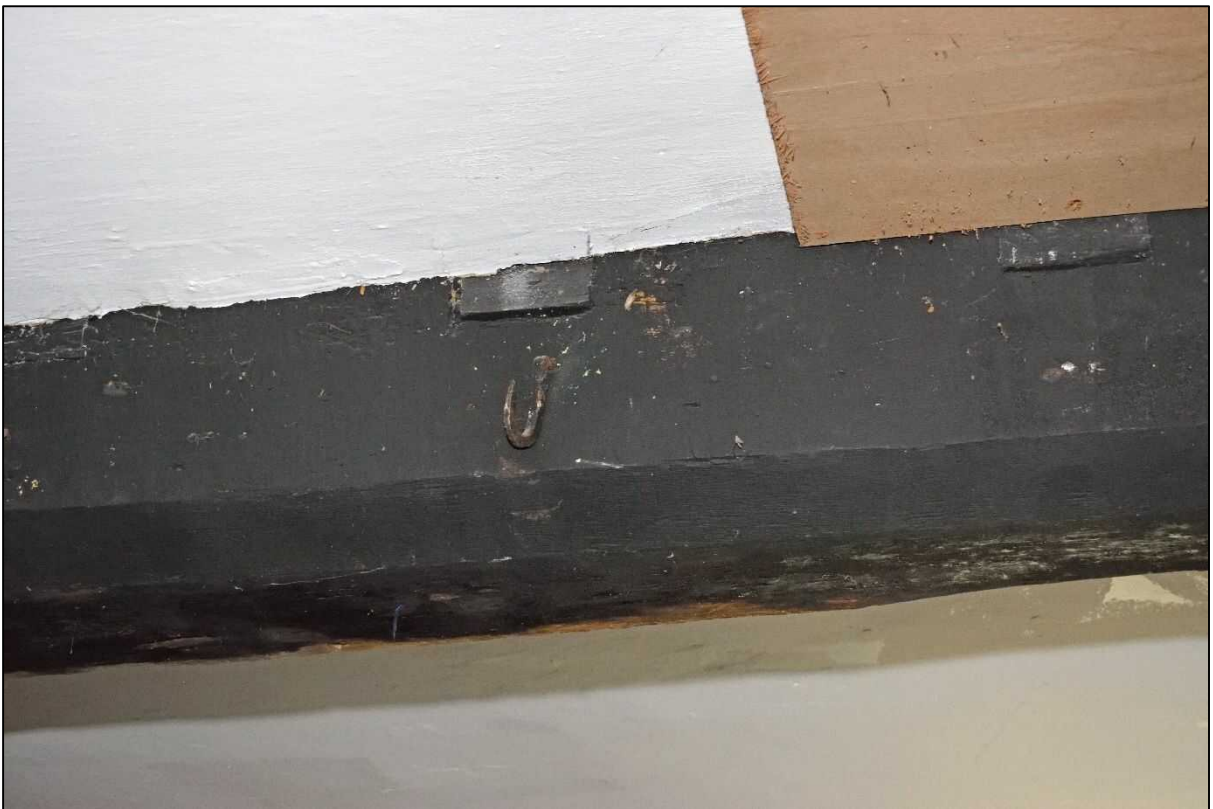
Plate 22: Hook on side of ceiling beam and filled mortices for joists
