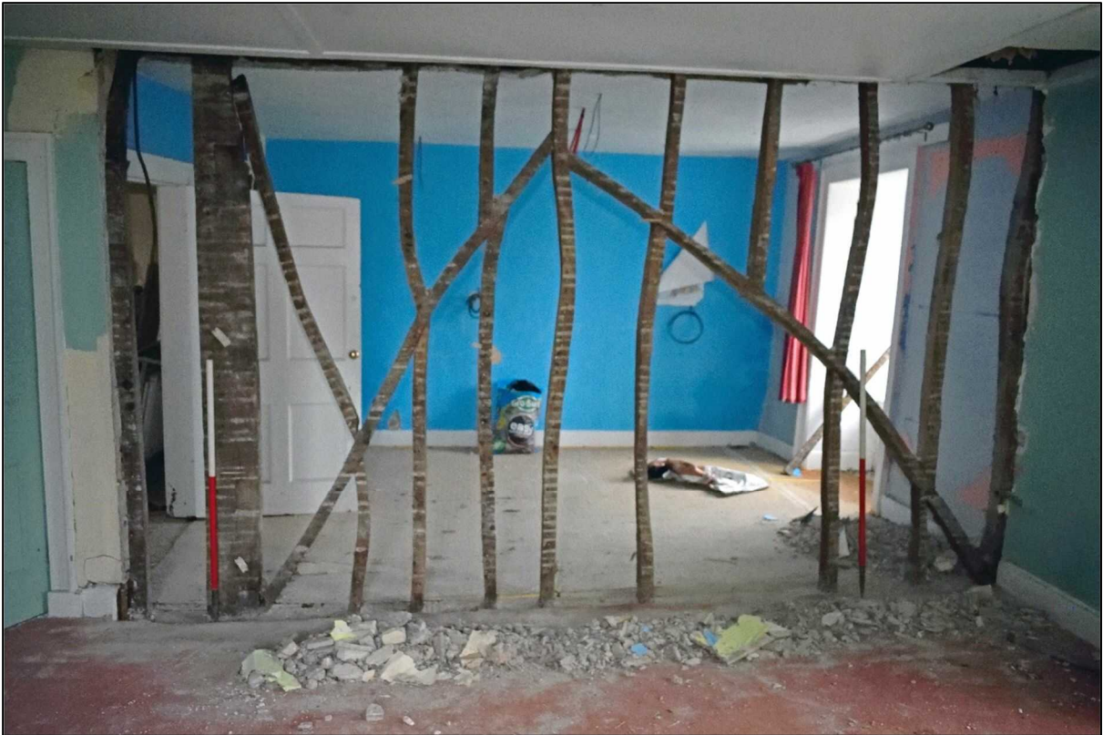
Plate 103: Framework of the partition between Bedrooms 2 and 3
