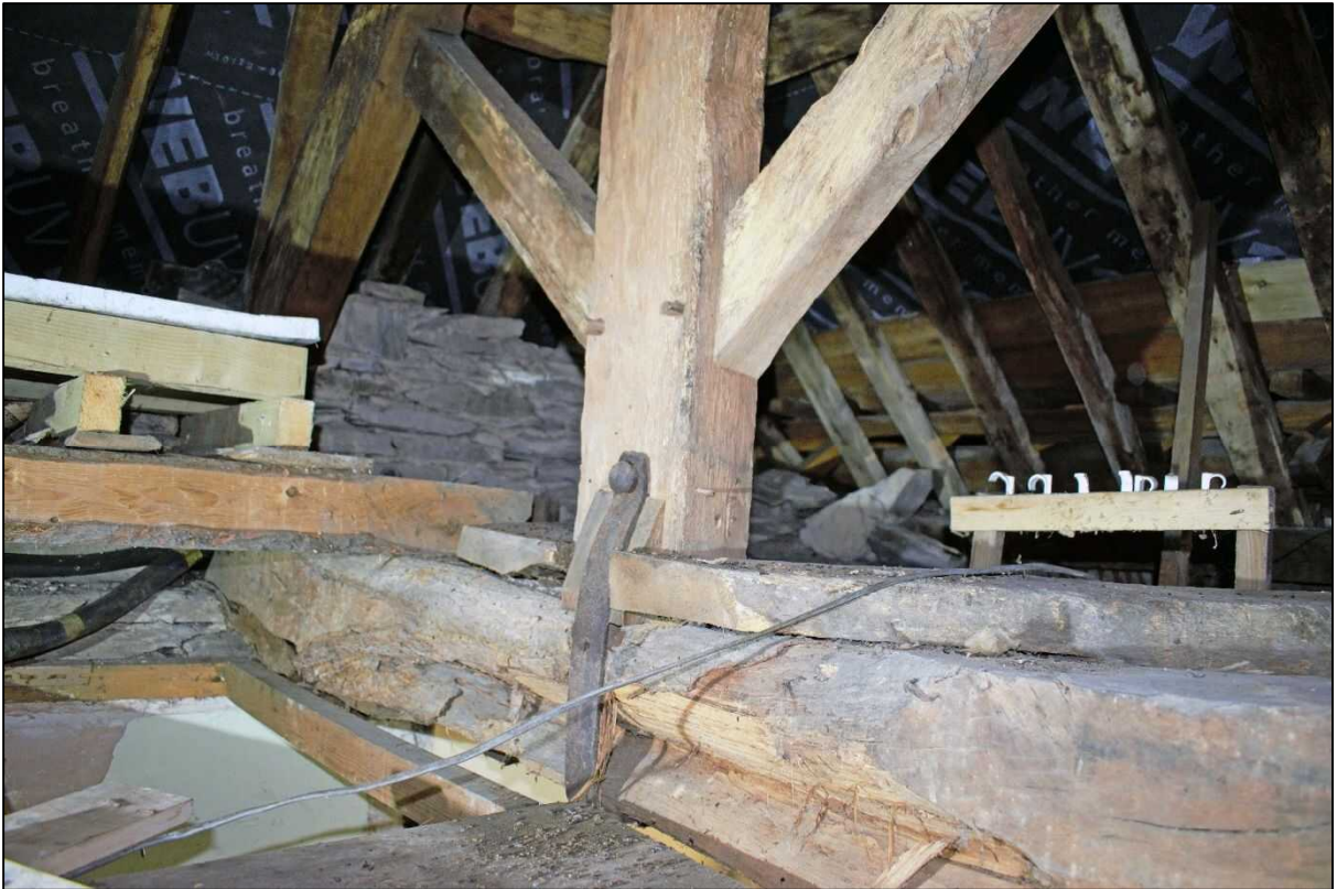
Plate 119: Twisted truss above Bathroom 2
